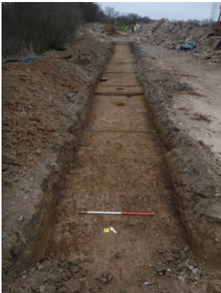
Photograph 7 T7, looking NE
