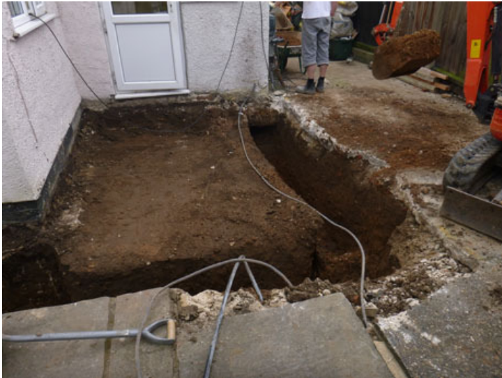
Photograph 1 Foundation trench, looking S
