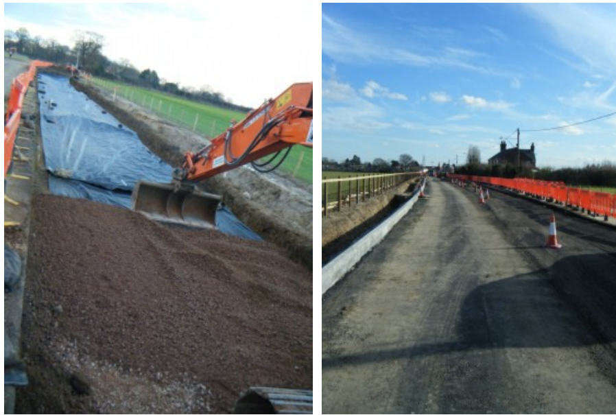
Photographs 7-8 Construction of new road/cycle path surface, looking N and S
