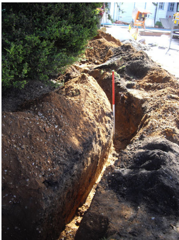
Photograph 5 Drainage trench from soakaway, looking E
