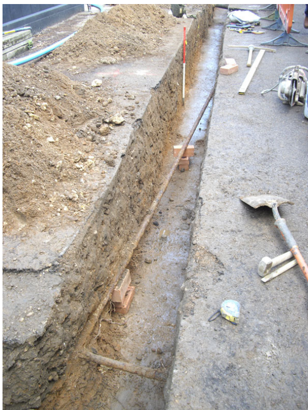
Photograph 2 Main drainage trench, looking SE
