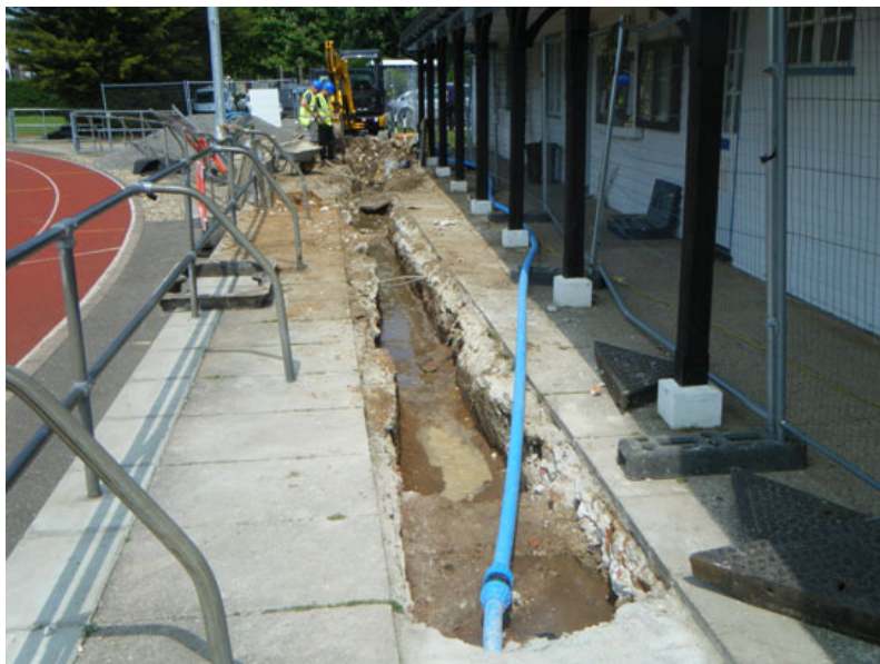
Photograph 1 Main drainage trench, looking N
