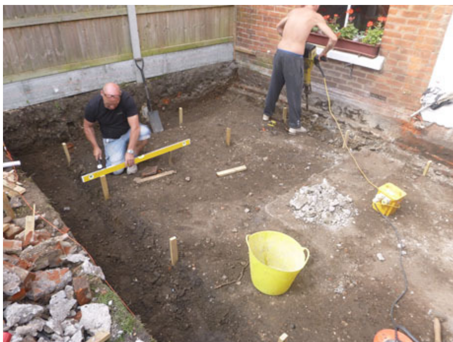
Photograph 1 Excavation of the footprint of the extension, looking SW
