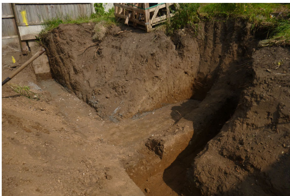
Photograph 1 Foundations of retaining wall, looking E
