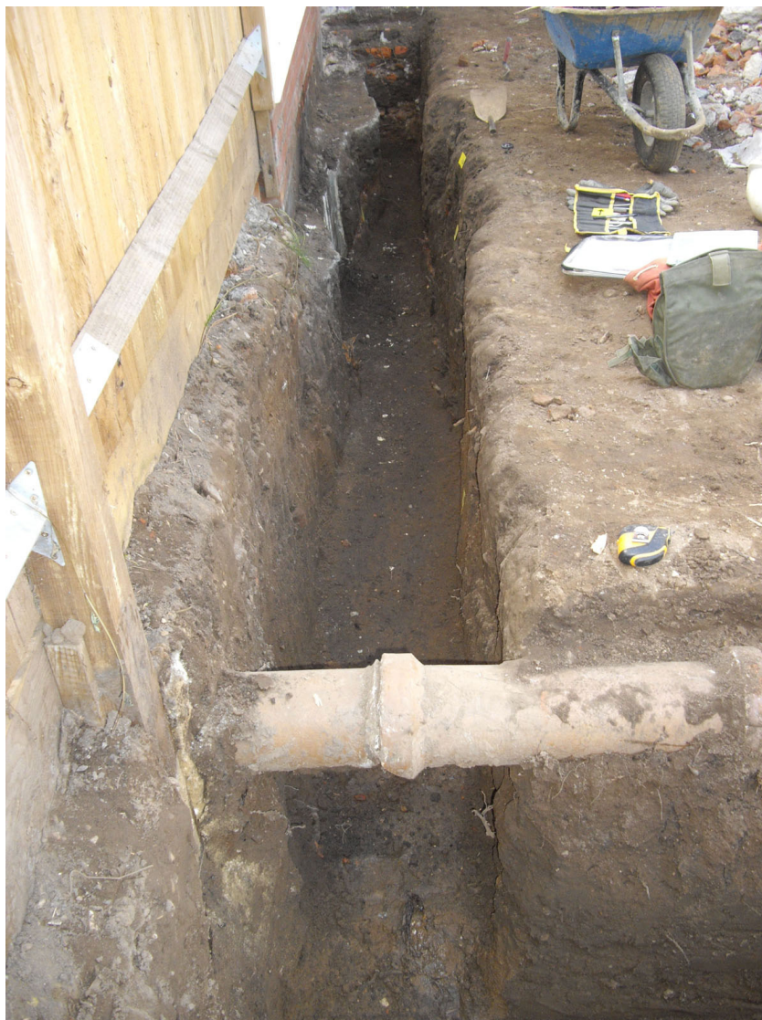
Photograph 2 Foundation trench for new extension, looking NW
