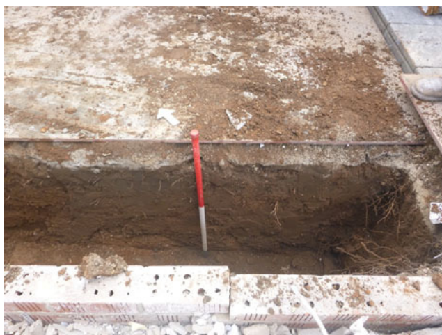
Photograph 2 Foundation trench, looking NE
