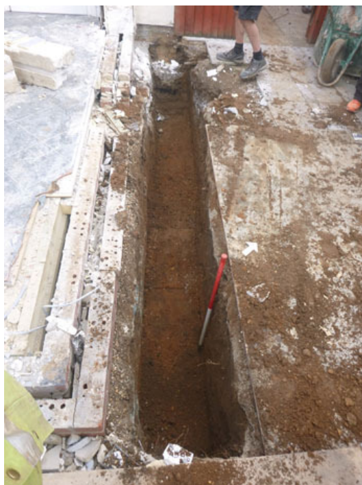
Photograph 1 Foundation trench, looking NW
