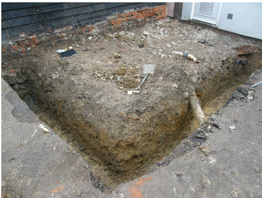
Photograph 2 Footings for the new extension, looking SW
