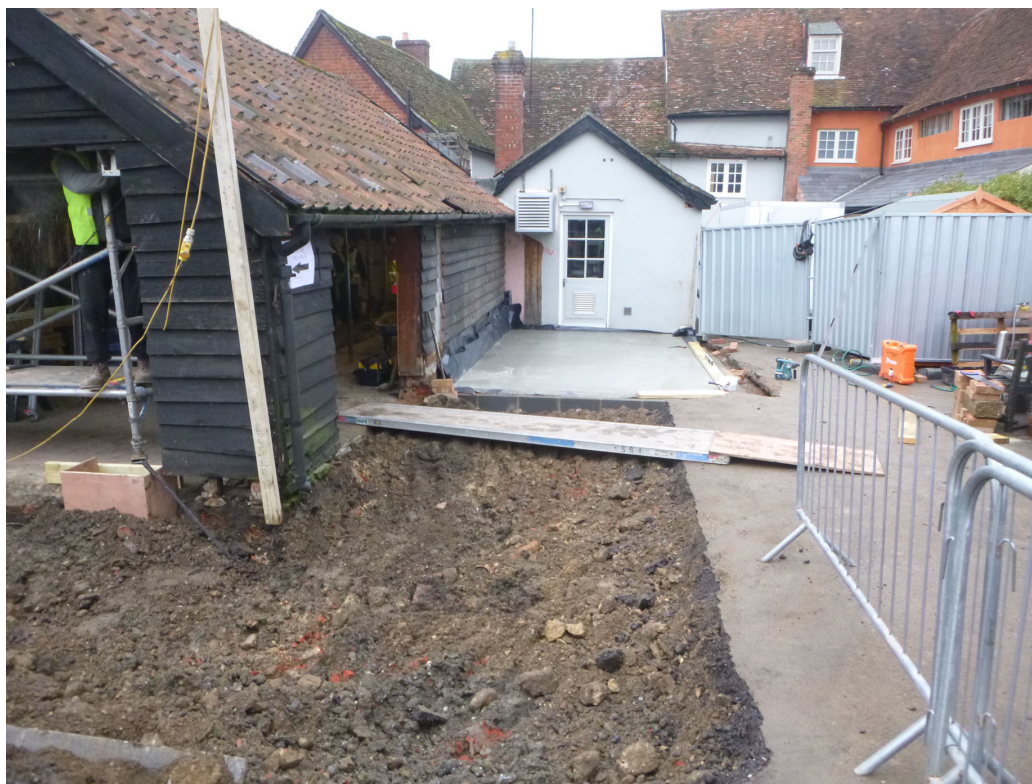
Photograph 3 Area stripped for new decking, looking W
