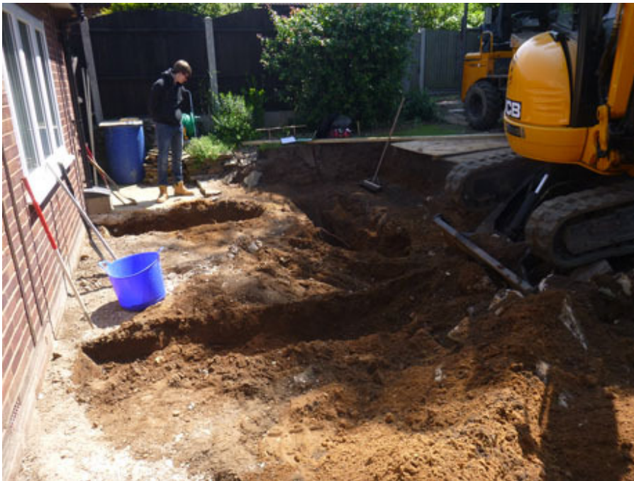
Photograph 1 Extension stripped of topsoil/subsoil and foundation trenches dug, looking E
