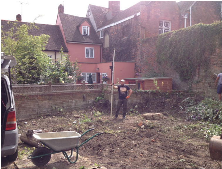
Photograph 1 The site after ground clearance
