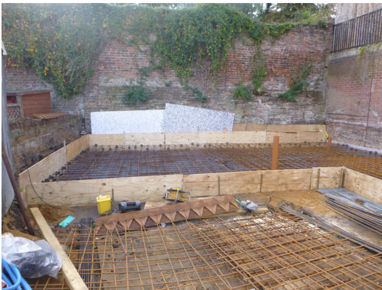
Photograph 2 Construction of the floating raft
