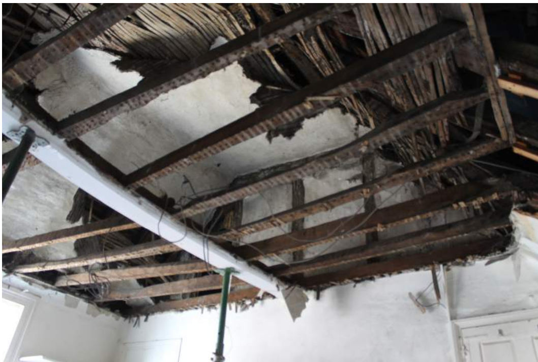
Photograph 6 Exposed ceiling joists with earlier lath and plaster ceiling above – view south-east
