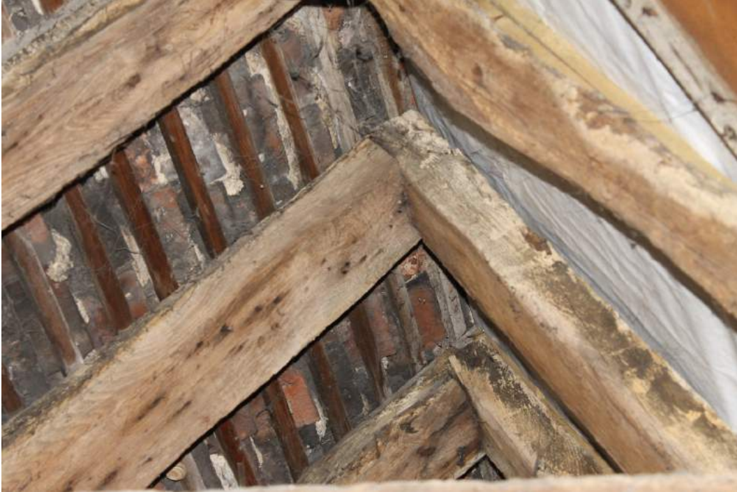
Photograph 14 Heads of the common rafters, single-pegged to each other
