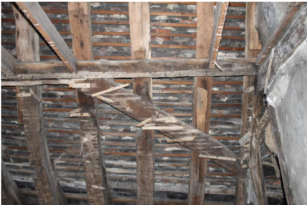
Photograph 13 Wind brace in street side roof pitch – view east
