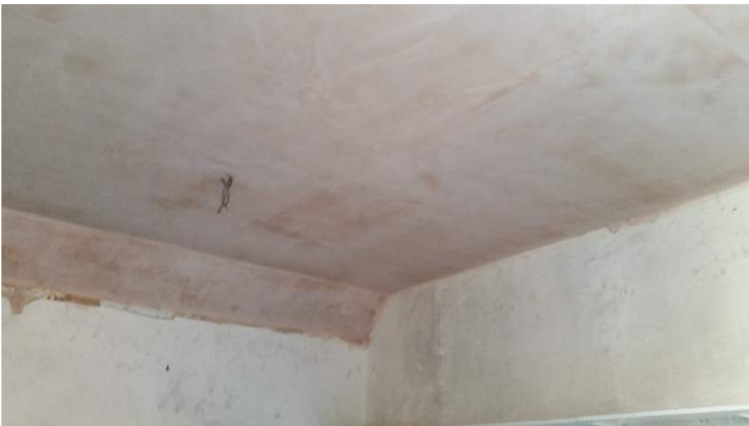
Photograph 18 The new ceiling prior to painting - view north-west
