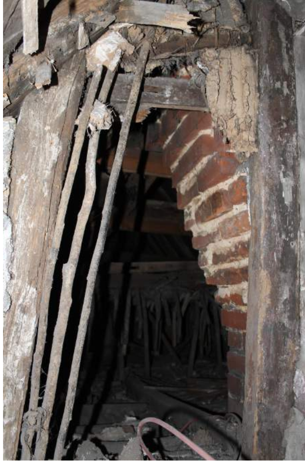
Photograph 12 Cross frame with the remains of one of the original wattle and daub infill panels – view south
