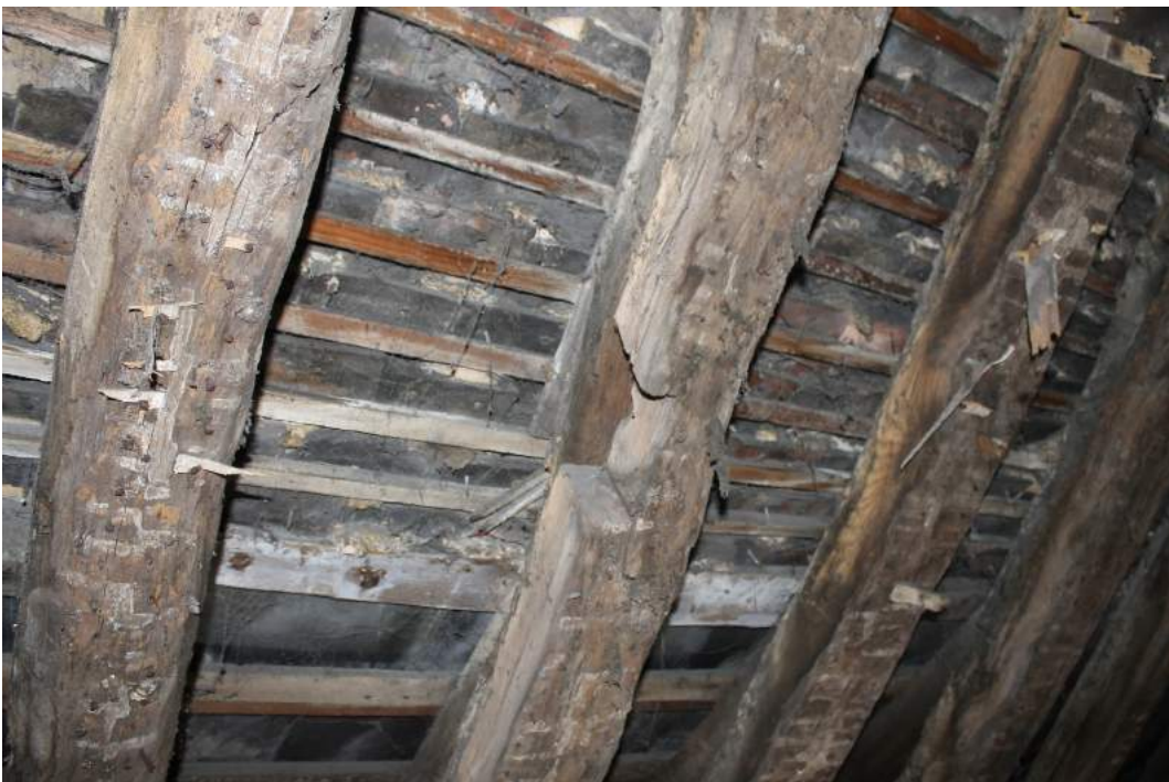
Photograph 11 Common rafter formed from re-used timber – view south-east
