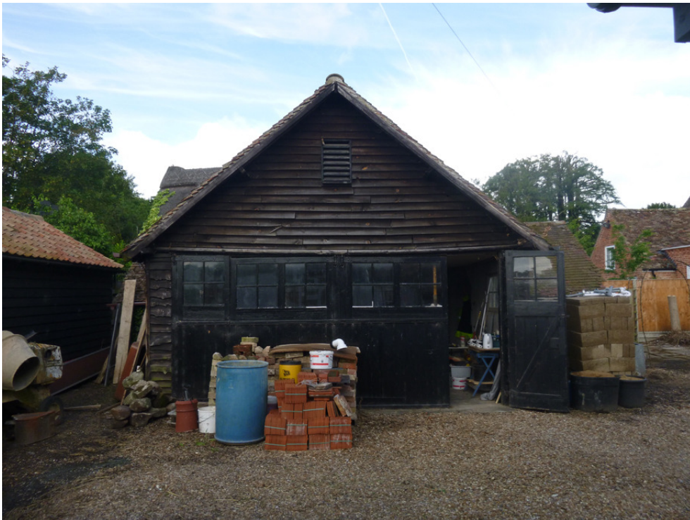
Photograph 2 East elevation – shot taken facing west.
