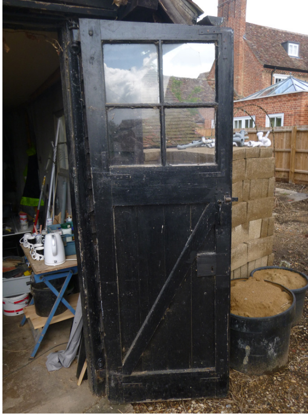
Photograph 13 Detail of single width door on east elevation – shot taken facing north-west.
