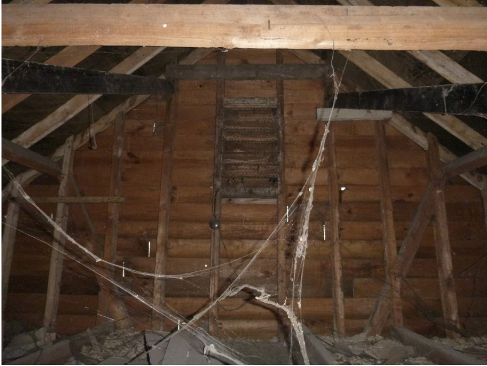
Photograph 15 Interior shot of west gable of main building. Additional timbers used to support tiled roof visible – shot taken facing west.
