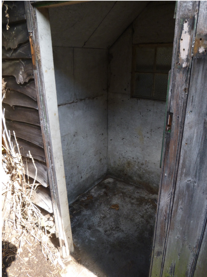
Photograph 6 Interior of separate room in south wing – shot taken facing north-west.
