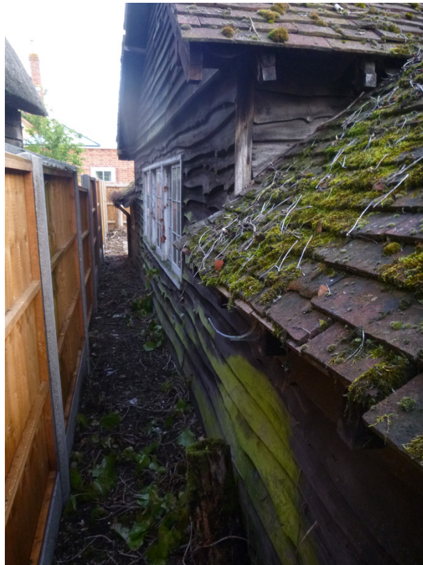
Photograph 4 West elevation – shot taken facing north.
