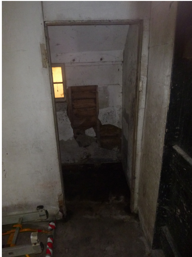
Photograph 14 Entrance into room in north wing, shot taken facing west
