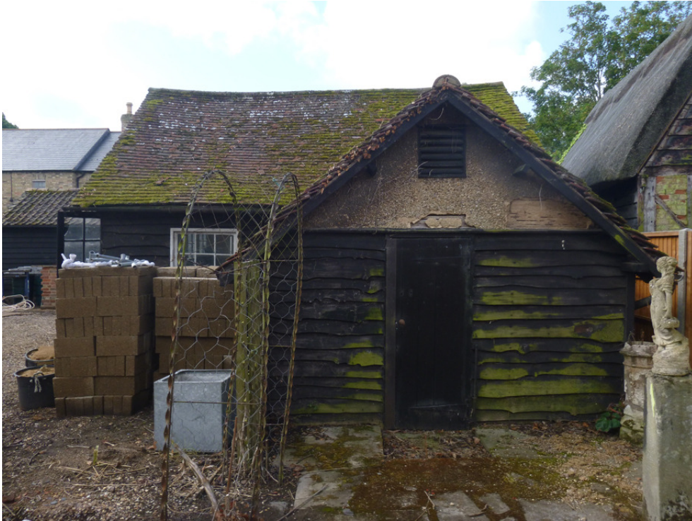
Photograph 1 North elevation – shot taken facing south.
