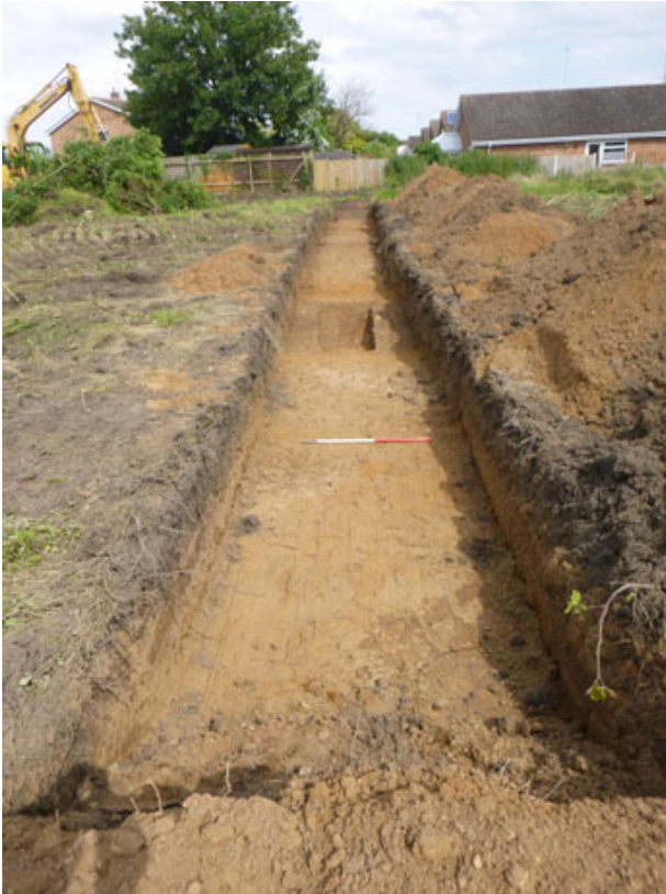
Photograph 3 T3, looking E
