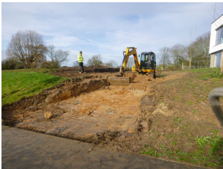
Photograph 1 Excavation of the haul road, looking NW
