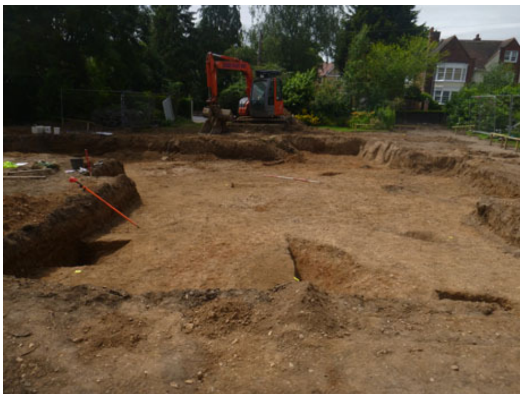
Photograph 3 General shot of strip within footprint of new dwelling, looking west
