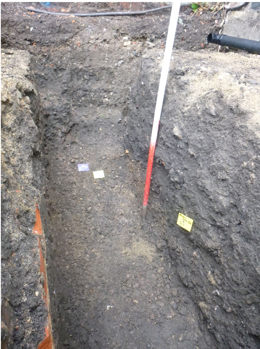
Photograph 1 Compacted gravel F1 (L2) at NW end of trench, looking NW
