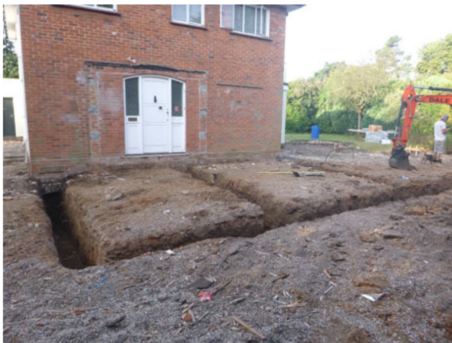
Photograph 1 Foundation trenches, looking SW
