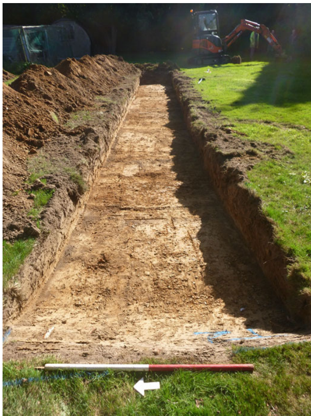
Photograph 2 T2, looking E
