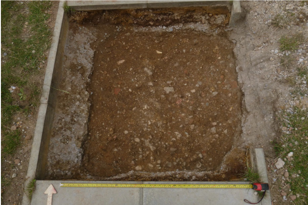
Photograph 3 Test-pit 1 showing top of 1930s backfill below footpath, looking N
