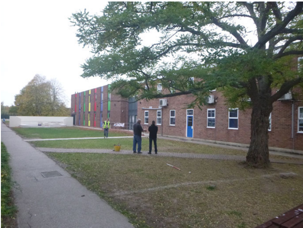
Photograph 8 Courtyard before excavation begins for the granite paving slabs, looking NW (amphitheatre can be seen in distance)
