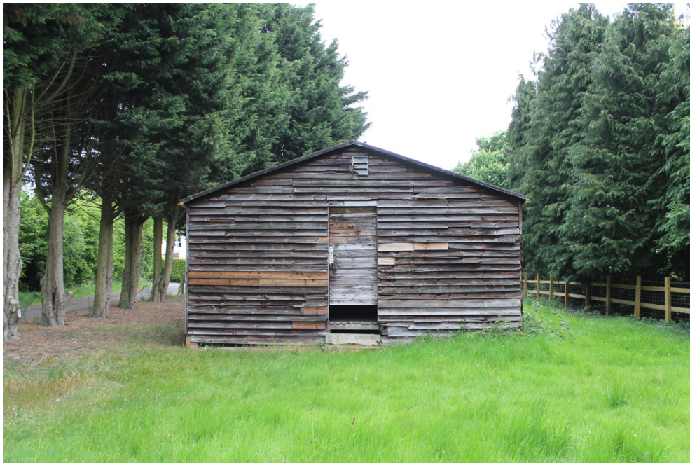
Photograph 4 West elevation of Hall. Photograph taken facing east.
