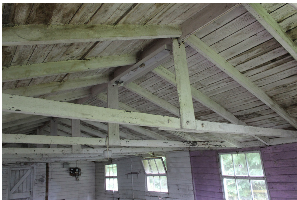
Photograph 6 King-post roof trusses. Photograph taken facing south-east.
