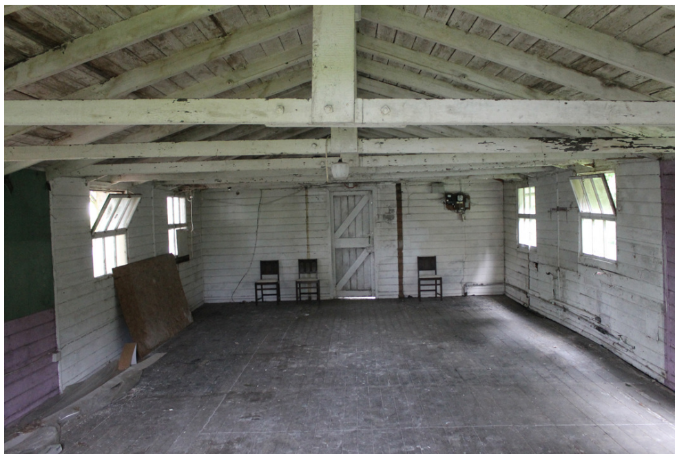
Photograph 5 Interior shot of Hall. Photograph taken facing east.
