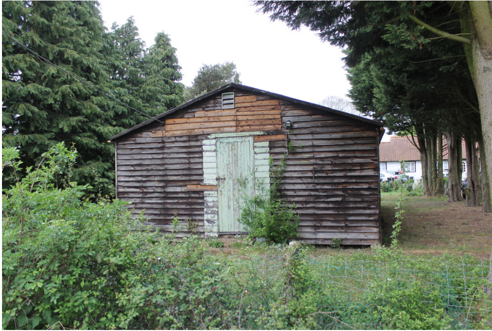
Photograph 3 East elevation of the Hall. Photograph taken facing west.
