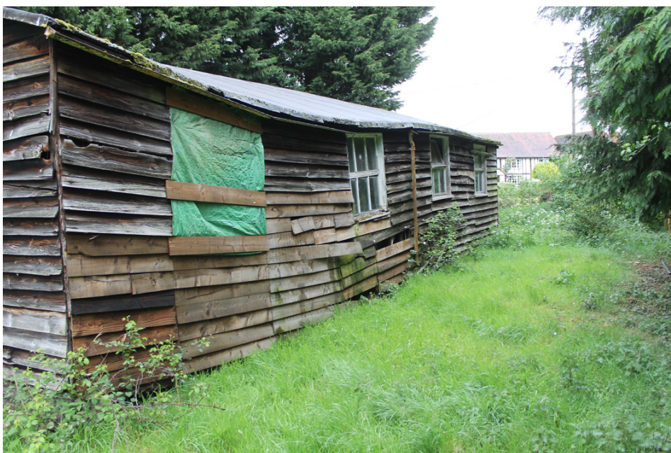
Photograph 2 South elevation of the Hall. Photograph taken facing north-east.
