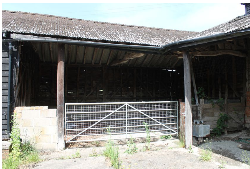
Photograph 24 South-east elevation of Building D. Photograph taken facing north-west.
