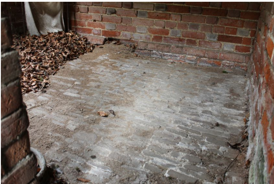
Photograph 36 Interior of original half of Building H, showing pavior brick floor. Photograph taken facing east.
