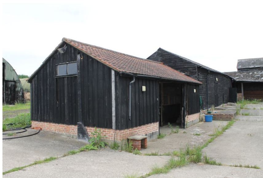
Photograph 16 South-west and south-east elevations of Building B. Photograph taken facing north-west.
