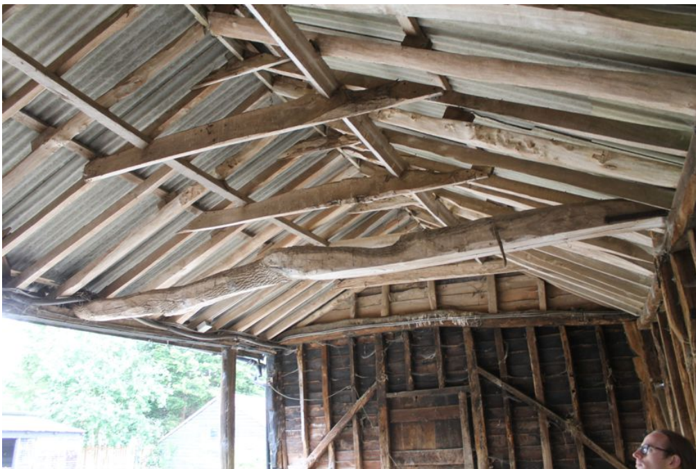
Photograph 26 Truss in Building D. Photograph taken facing south.
