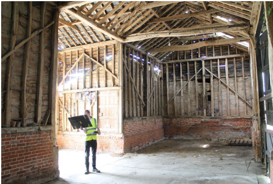
Photograph 4 Interior shot of barn, showing timber-frame. Photograph taken facing west.
