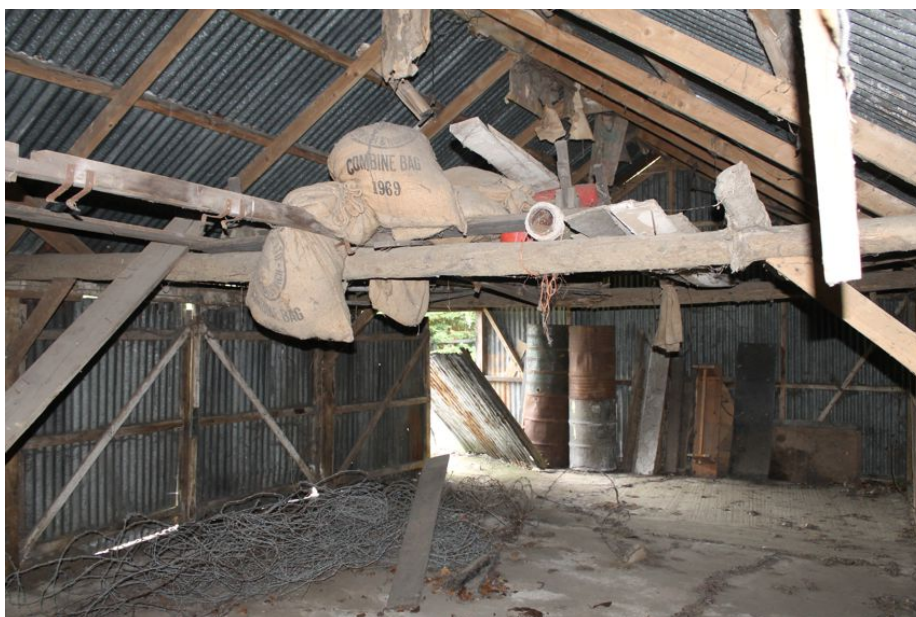
Photograph 15 Interior shot of Building A. Photograph taken facing north-west.
