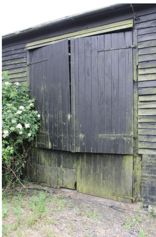
Photograph 2 North-east elevation of barn, showing barn door. Photograph taken facing south.
