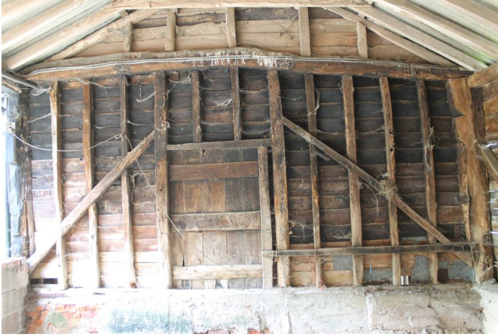
Photograph 28 South-west elevation of Building D, with double jowled corner post visible to right of photo. Photograph taken facing south-west.
