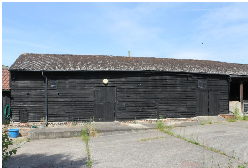
Photograph 19 South-east elevation of Building C. Photograph taken facing north-west.
