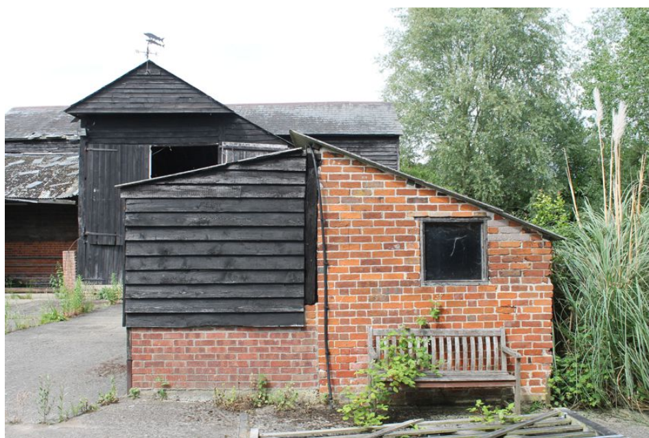
Photograph 34 South-west elevation of Building H, showing two phases of construction. Photograph taken facing north-east.
