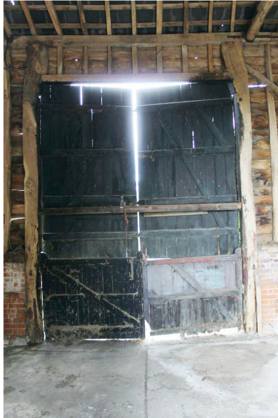
Photograph 8 Interior shot of the door on the north-west elevation of the barn. Large posts with jowled heads visible on either side of doorway. Photograph taken facing north-west.
