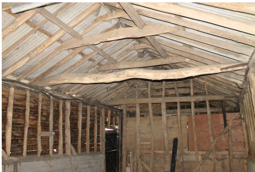
Photograph 22 Roof truss in Building C. Photograph taken facing south.
