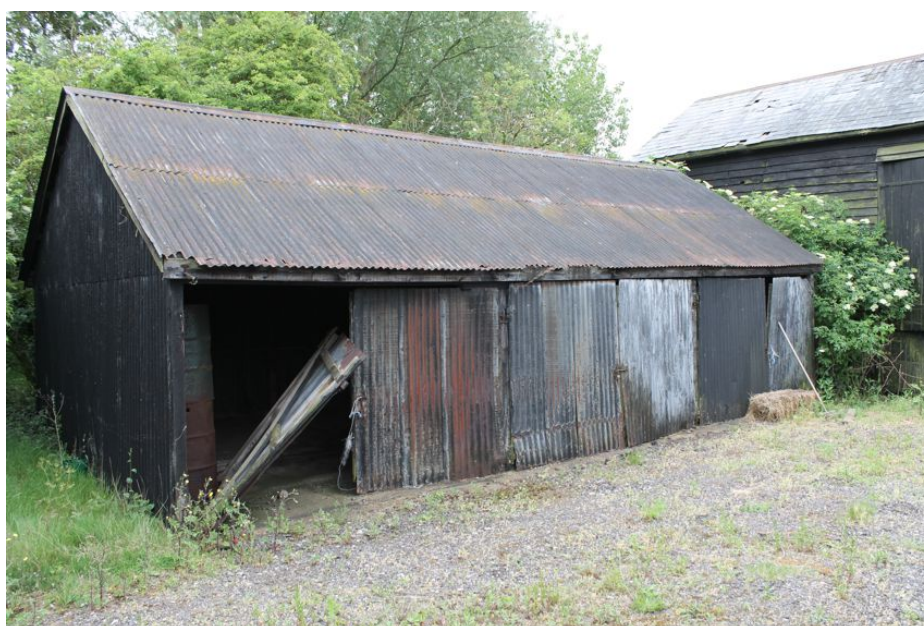
Photograph 14 Exterior shot of Building A. Photograph taken facing south-east.
