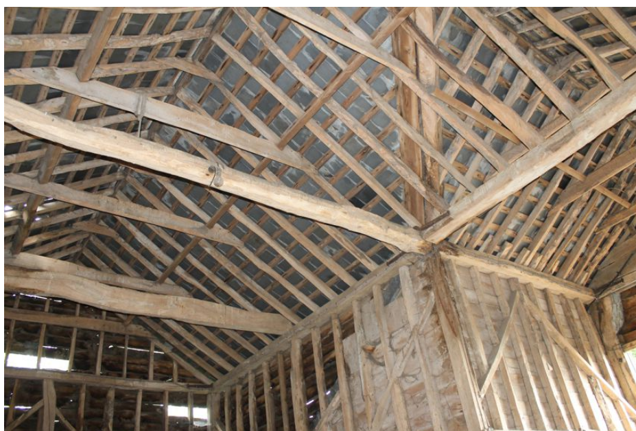
Photograph 13 Shot showing the tie-beam between bays 3 and 4 is the same timber as the wall-plate of the midstrey. Photograph taken facing south.
