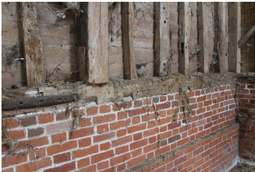
Photograph 5 Detailed shot of sill-beam on the south-east end of bay 1. Photograph taken facing west.
