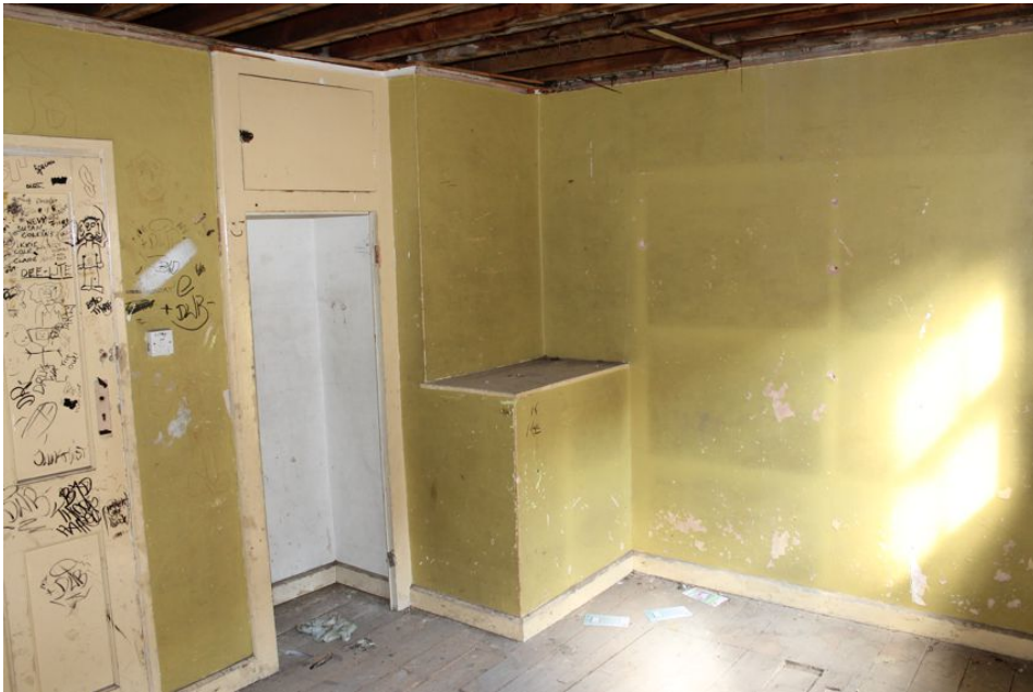
Photograph 74 First-floor of Building D, showing internal divisions. Photograph taken facing north-east.
