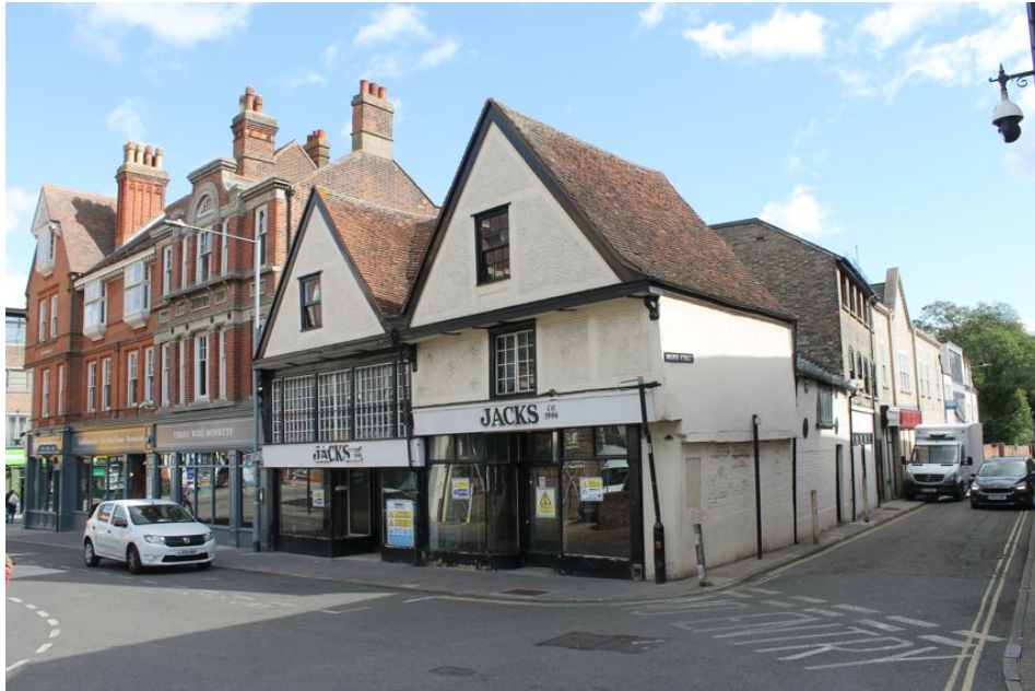
Photograph 36 Entire site, showing Buildings A, B, C and D. Underbuilding in brick below Building B's southern jetty visible. Photograph taken facing north-east.
