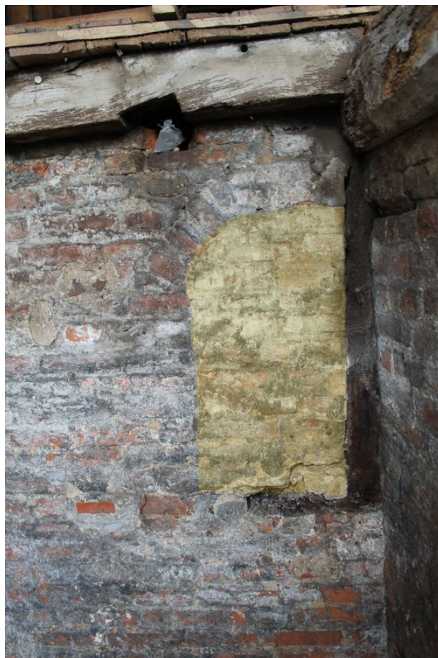
Photograph 50 Highlighted blocked archway in eastern wall of cellar, including post supporting binding-beam. Photograph taken facing east.
