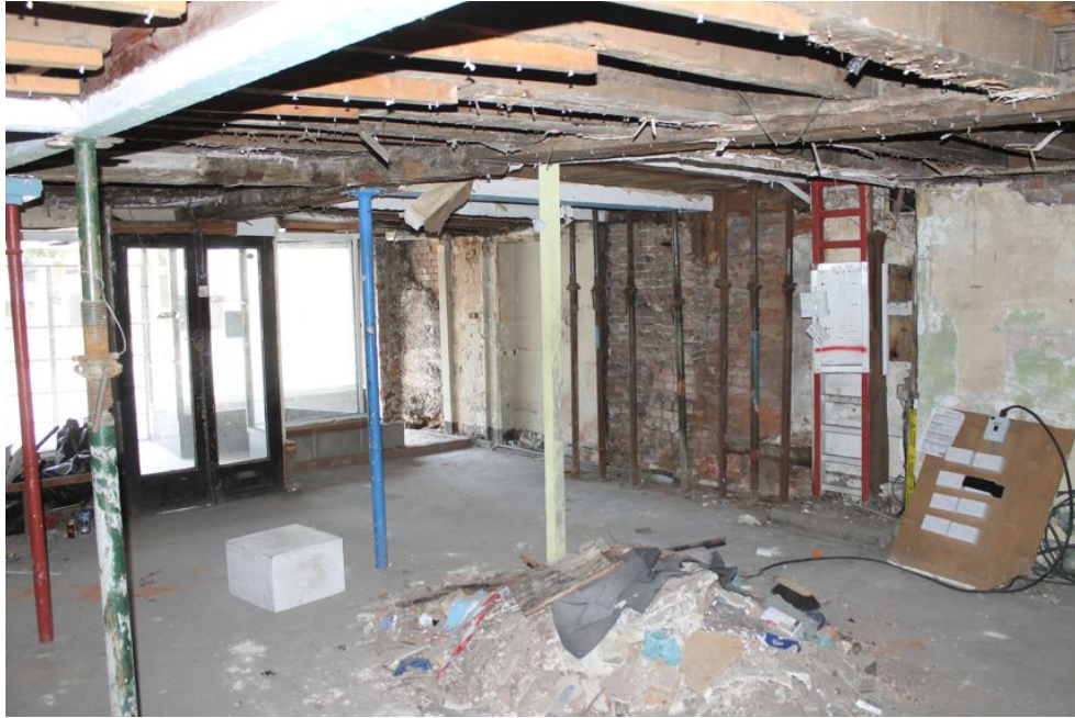
Photograph 6 Ground-floor of Building A. Photograph taken facing north-west.
