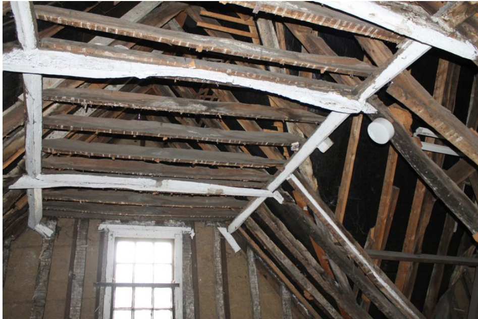
Photograph 60 Roof of Building B, showing original collars and purlins, as well as later braces. Photograph taken facing west.
