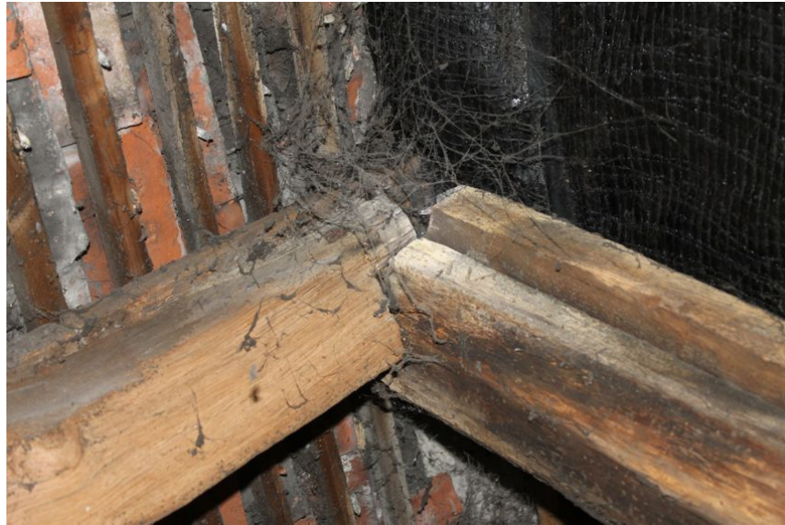
Photograph 28 Carpenter's mark "IV" at apex of rafters in Building A.
