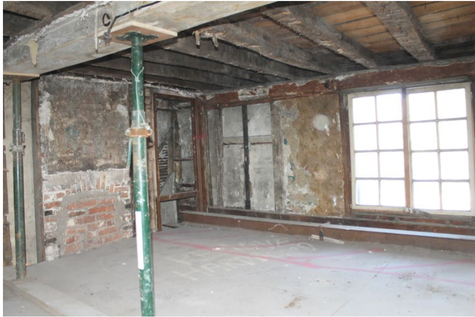
Photograph 54 First-floor of Building B, showing blocked fireplace and raised floor level. Photograph taken facing south-west.
