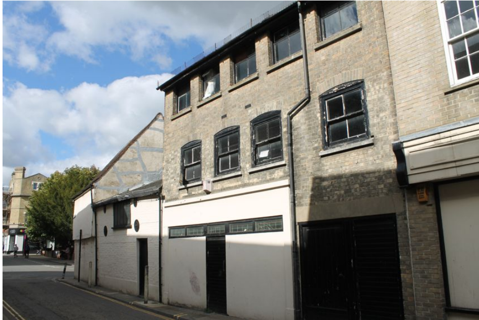
Photograph 70 Southern elevation of Building D in foreground, with Buildings D and B in background. Photograph taken facing north-west.
