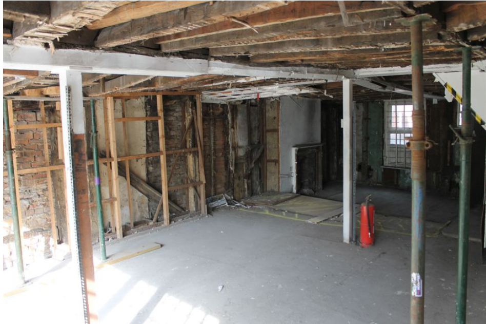
Photograph 15 First-floor in Building A. Photograph taken facing north-east.
