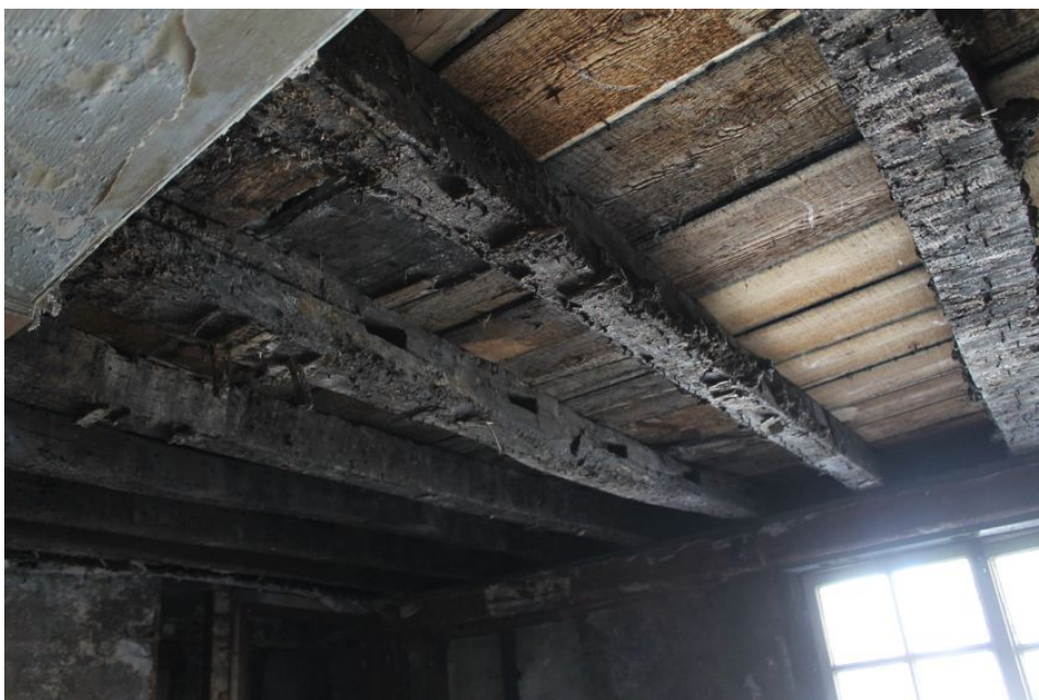
Photograph 59 Unused mortices on joist of second-floor of Building B. Photograph taken facing south-west.
