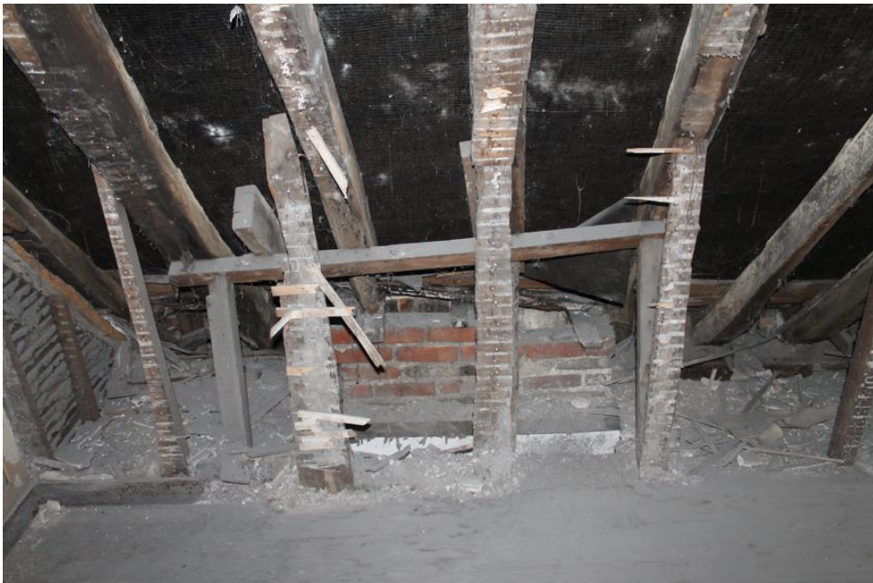
Photograph 35 Remaining top of chimney-stack in Building A. Possible original lath and plaster on east side of modern skylight visible to left. Photograph taken facing north.
