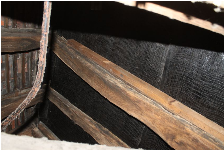
Photograph 29 Carpenter's mark "IIII" on side of rafters in Building A.
