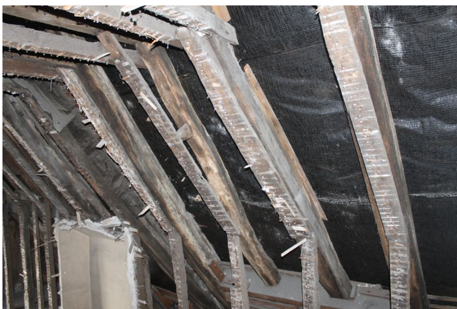
Photograph 27 Smoke-blackening on rafters in Building A. Shows variation in smoke-blackening from centre of building (right) outwards. Photograph taken facing north-west.
