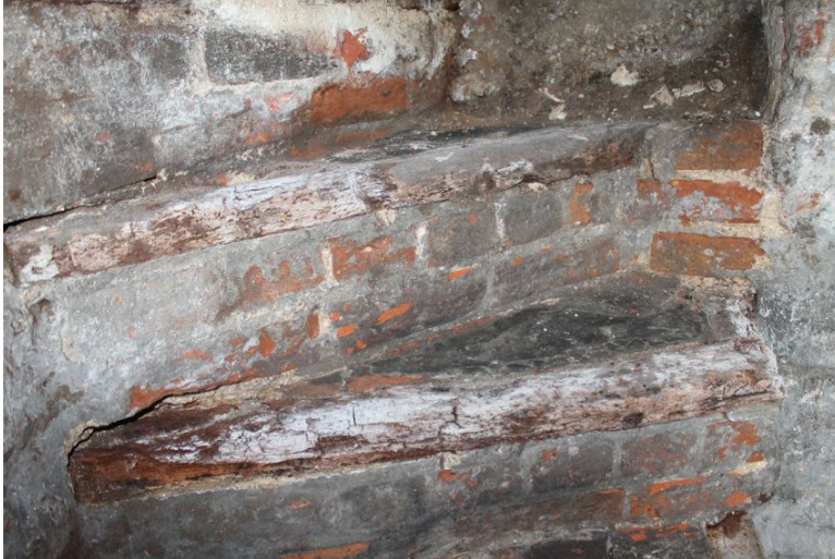
Photograph 44 Detail of steps on stairway. Photograph taken facing north-east.
