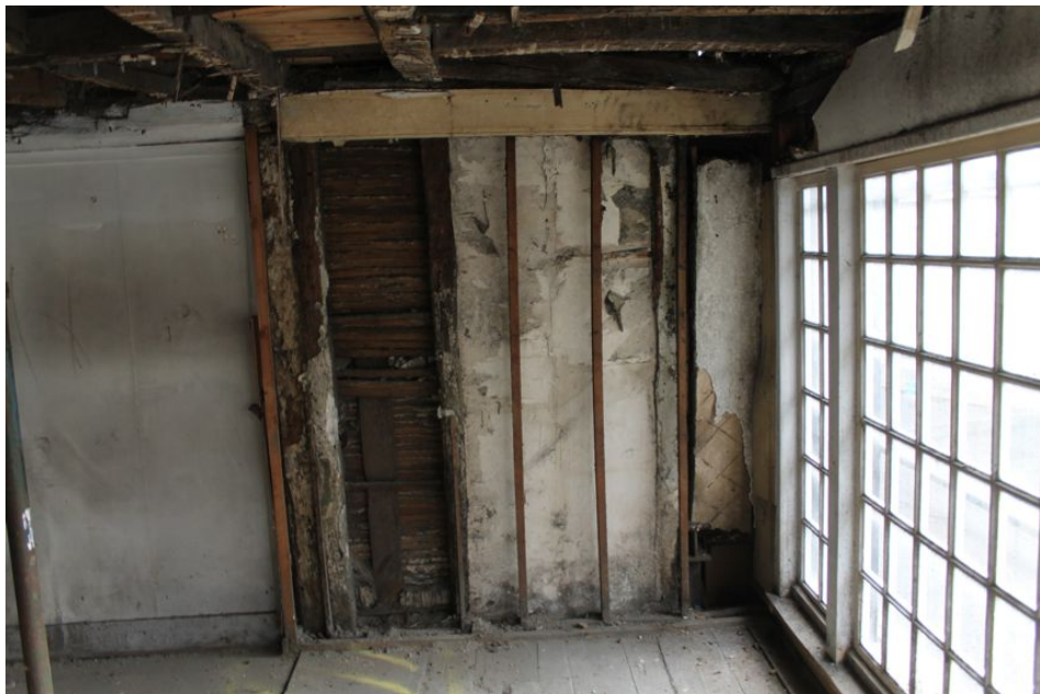
Photograph 20 Photograph of internal southern elevation of first-floor in Building A. Exposed lath and plaster render visible on exterior of building, as well as bricked over inserted door between Buildings A and B. Photograph taken facing south.
