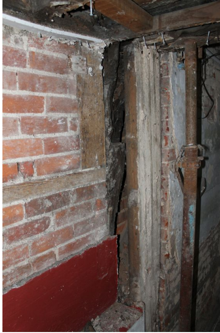
Photograph 7 Remains of north-east corner-post of Building A at the ground floor. Photograph taken facing north-east.
