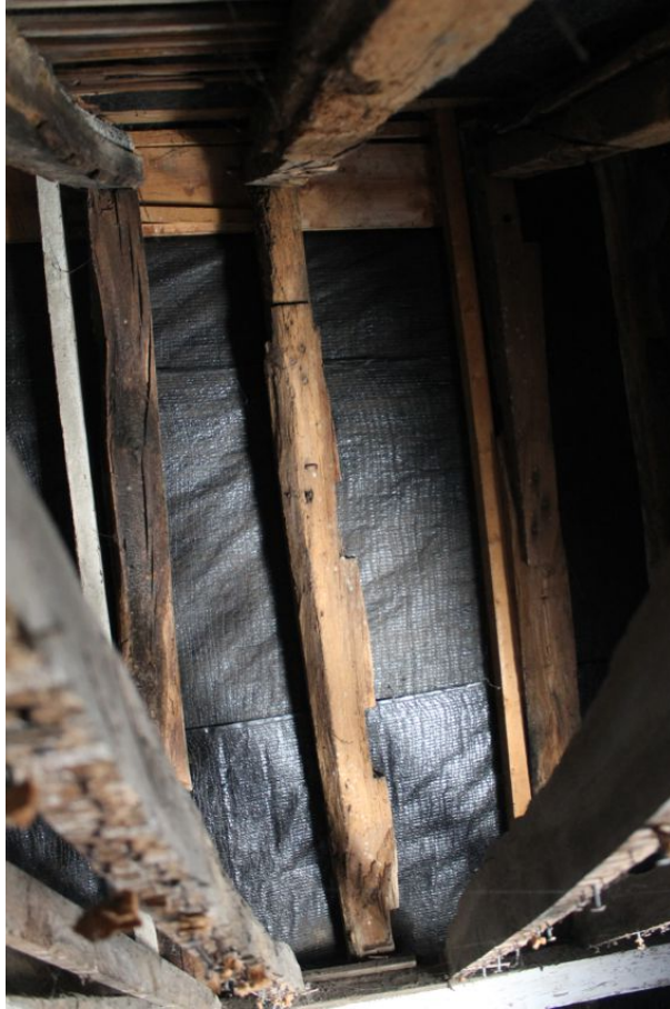
Photograph 62 Reused timber in roof of Building B, and evidence of smoke-blackening. Photograph taken facing south.
