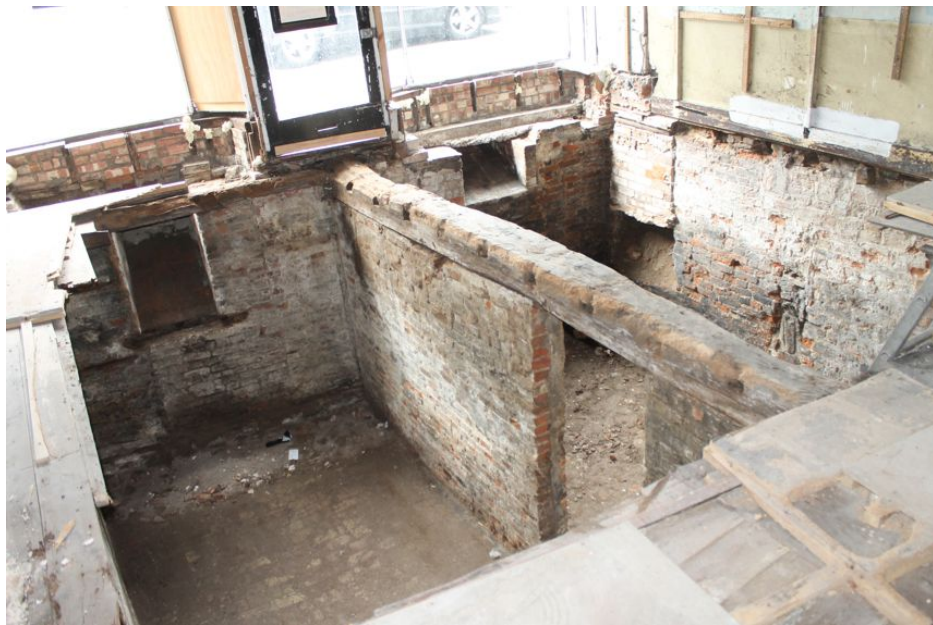
Photograph 37 Brick-built cellar below Building B. Photograph taken facing north-west.
