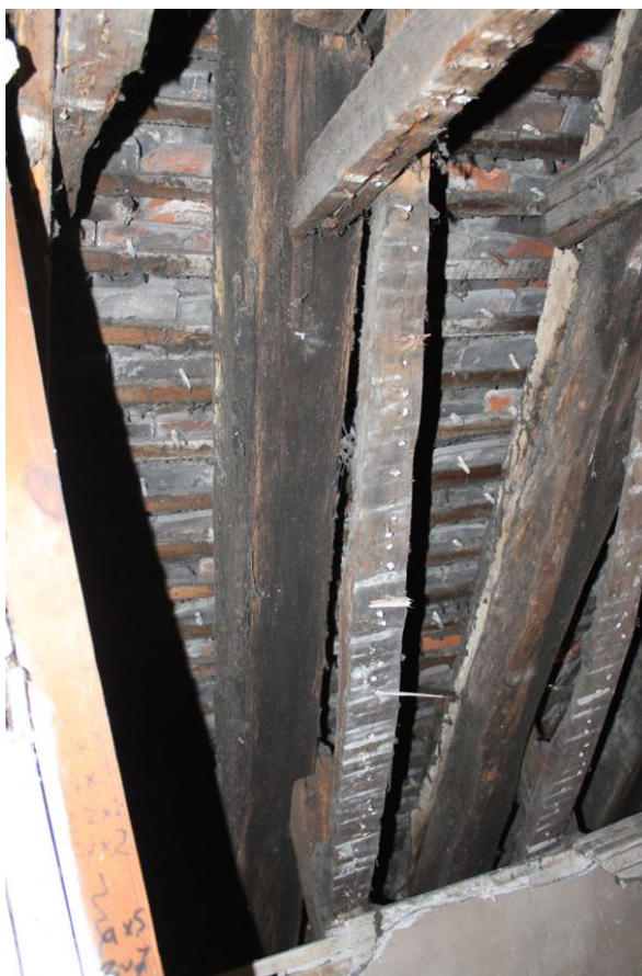
Photograph 26 Detail of smoke-blackening on rafters in centre of Building A. Photograph taken facing south-west.
