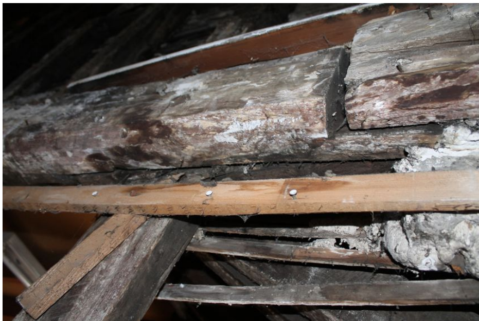
Photograph 56 Detail of scarf joint on eastern wall-plate of Building B.
