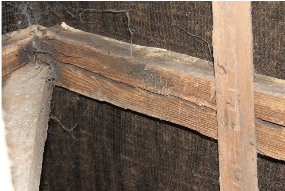
Photograph 30 Carpenter's mark "XIII" on side of rafters in Building A.
