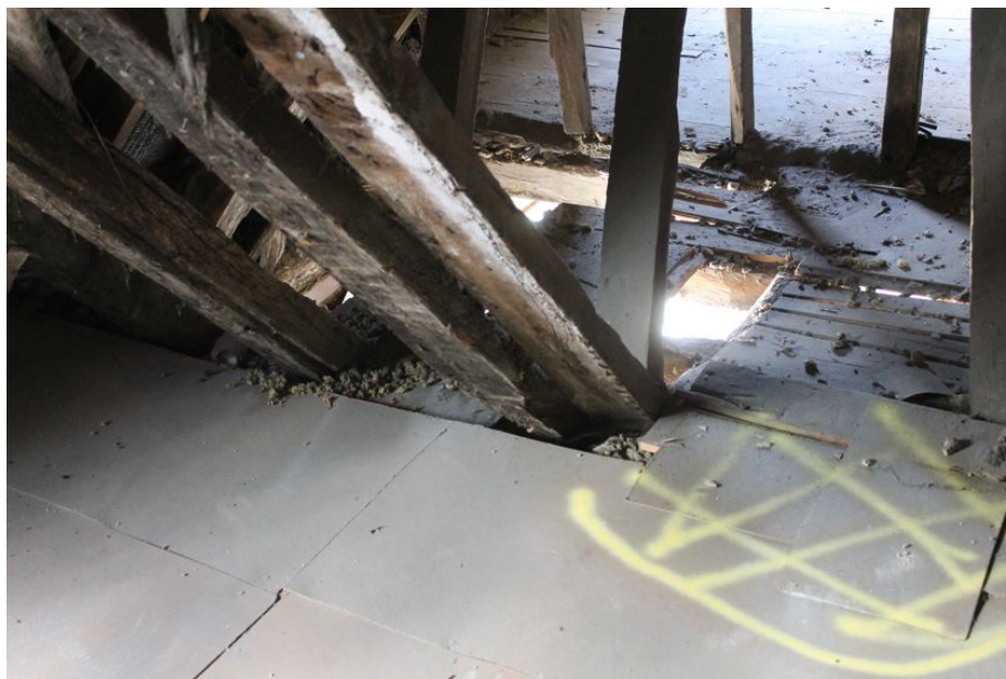
Photograph 66 Two rafters rising from one point on wall-plate to north of Building B. Photograph taken facing north-west.
