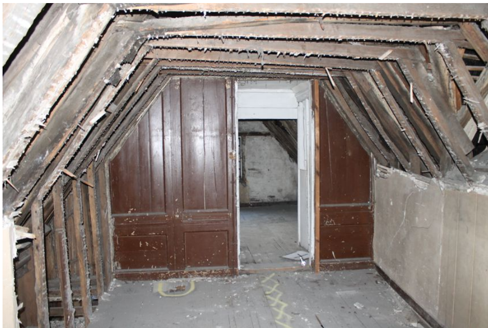
Photograph 23 West room on second-floor of Building A. Photograph taken facing east.
