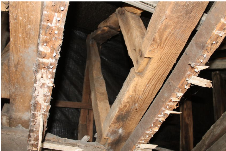
Photograph 31 Queen and king-posts nailed in place on the two westernmost collars in Building A.
