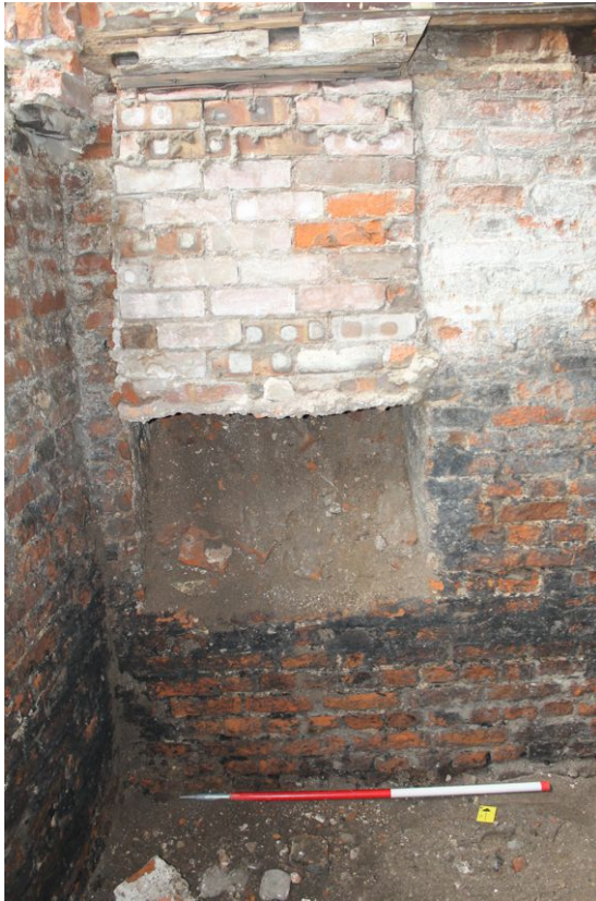
Photograph 42 Bricked-up opening in northern elevation of cellar. Photograph taken facing north.
