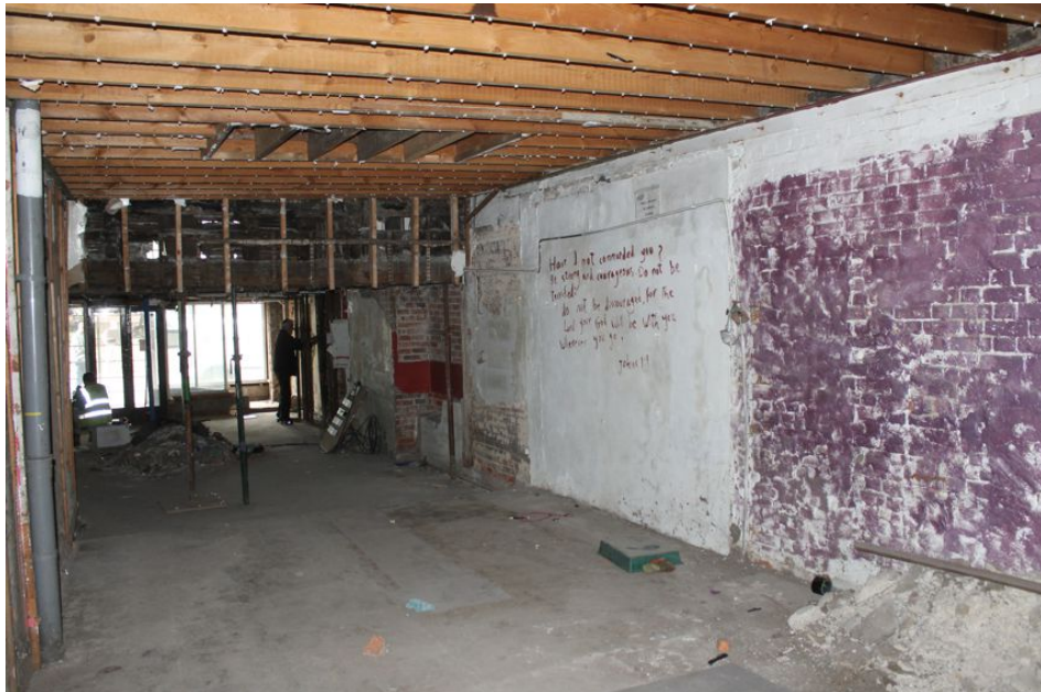
Photograph 78 Interior of Building E. Photograph taken facing north-west.
