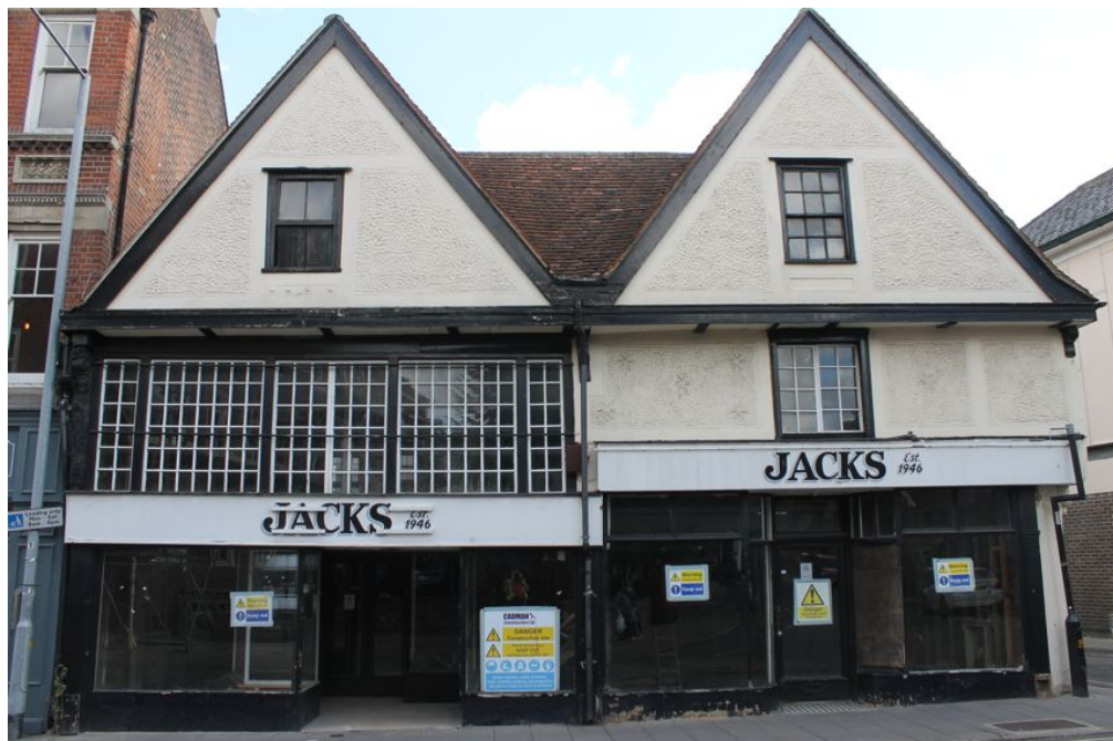
Photograph 2 Current western elevation of Buildings A (left) and B (right).
