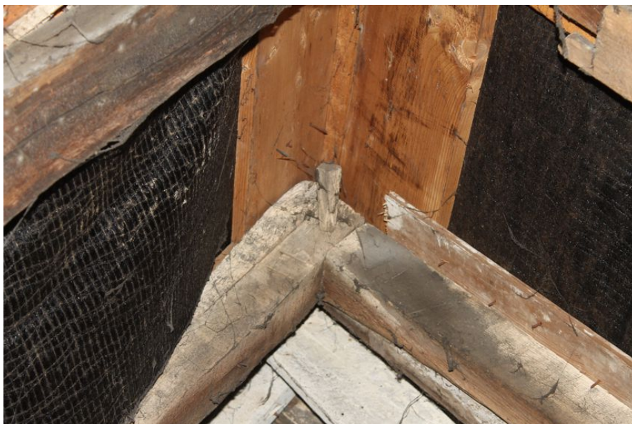
Photograph 63 Carpenter's mark "III" at apex of roof in Building B. Photograph 63 Carpenter's mark 'III' at apex of roof in Building B.
