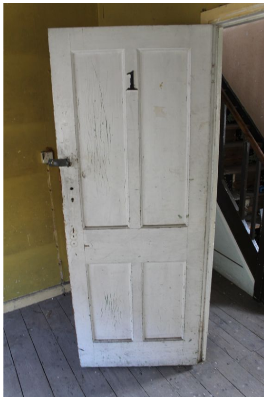
Photograph 75 Four-paneled door on first-floor of Building D. Photograph taken facing north-west.
