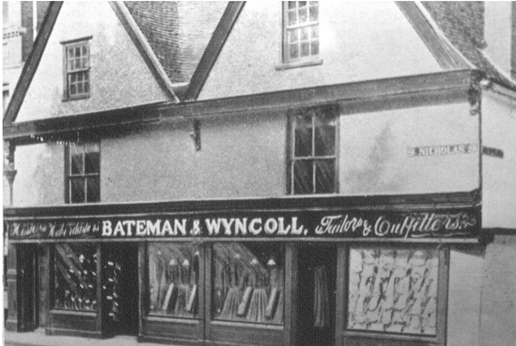
Photograph 1 Western elevation of 5 & 6 St Nicholas Street (Buildings A and B), taken in 1908. Note different windows and shop front (and lack of pargeting) compared to modern appearance (Photograph 2). Taken from www.gazette-news.co.uk/history/1528359.NOSTALGIA_Pictures_of_the_1d_JacksHardware_store_as_it_used_to_be Labelled as being from a Colchester Guide book in 1908.
