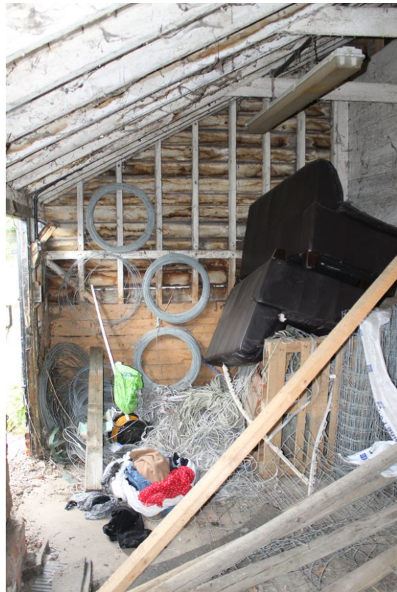
Photograph 6 Interior of outshot A. Photograph taken facing west.
