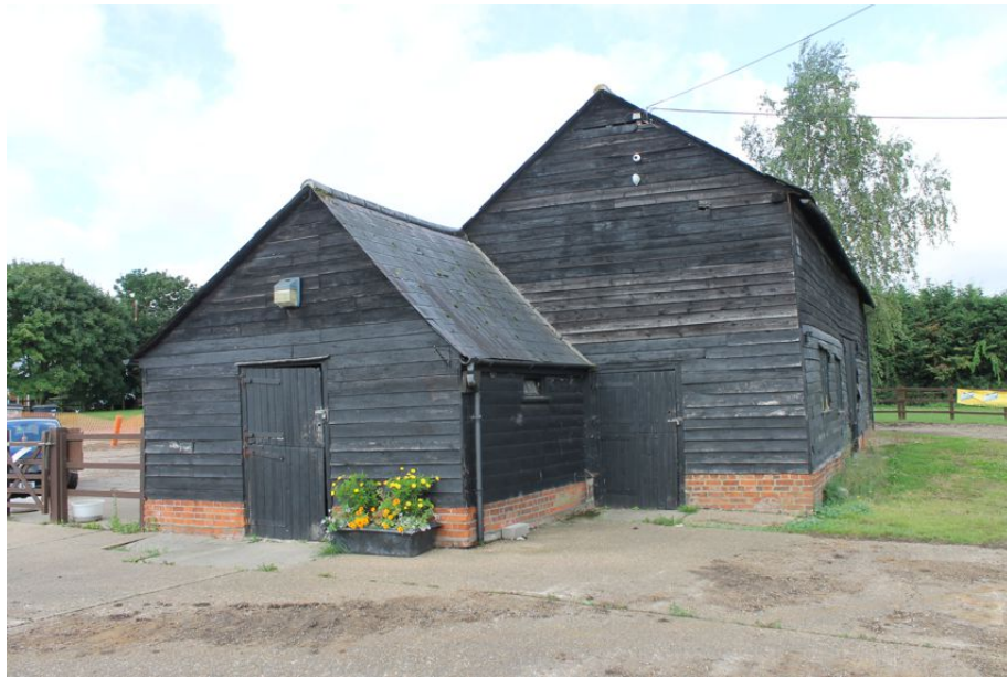
Photograph 5 Eastern elevation of barn and outshot B. Photograph taken facing west.
