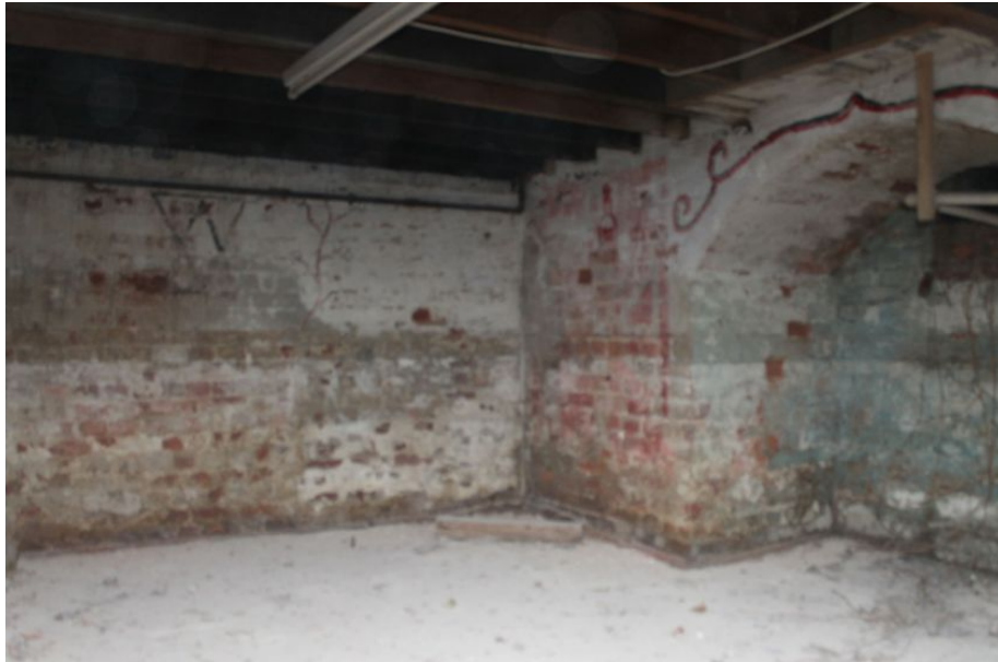
Photograph 28 Interior of farmhouse cellar. Photograph taken facing southwest.
