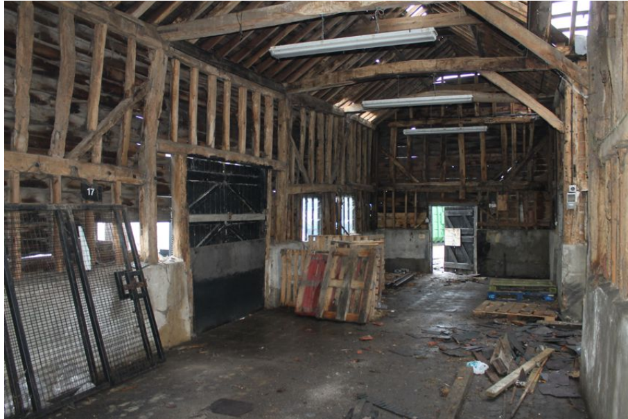
Photograph 8 Interior of barn. Photograph taken facing north-east.
