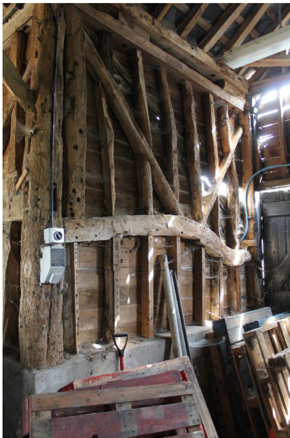
Photograph 20 Eastern elevation of midstrey. Photograph taken facing south-east.
