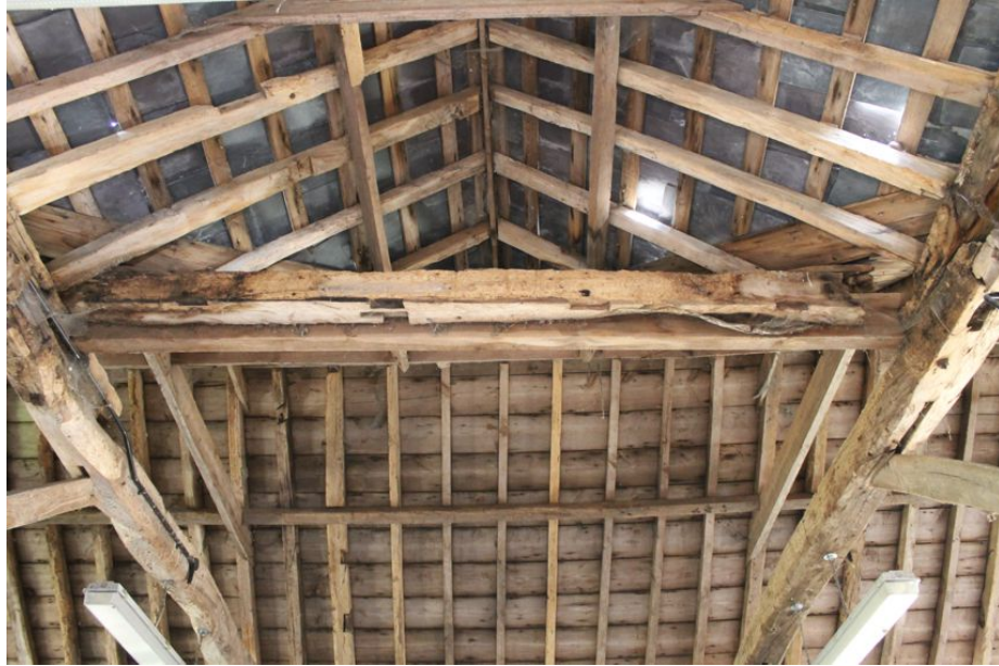
Photograph 19 Timber supported between two central tie-beams in the barn. Might possibly have been the original wall-plate on the southern elevation of bay 3. Photograph taken facing north.
