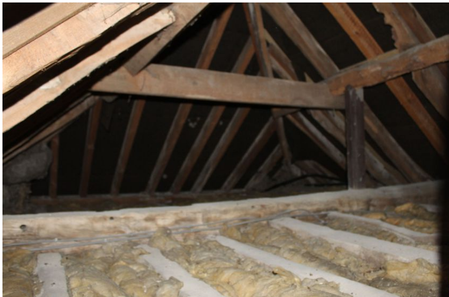
Photograph 39 Roof of farmhouse, showing rebuilt south hip. Photograph taken facing south-west.
