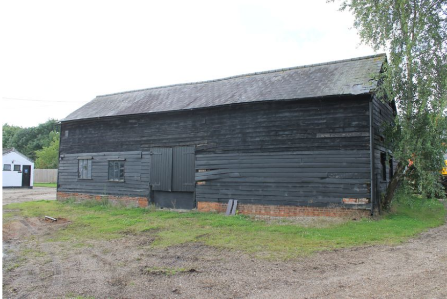
Photograph 2 Northern elevation of barn. Photograph taken facing south-east.
