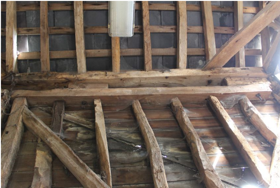
Photograph 21 Eastern wall-plate of midstrey, with multiple timbers. Photograph taken facing east.
