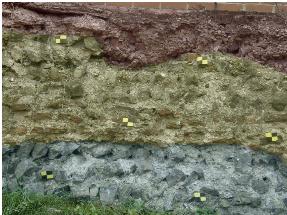
Photograph 7 Section of wall highlighted to show differing phases of fabric. At the top is the modern concrete capping, the middle is medieval facing, the bottom is the Roman core. Photograph taken facing south.
