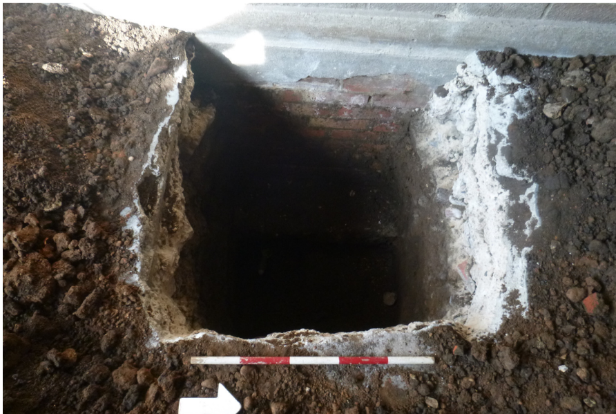
Photograph 2 Excavation of TP2 view west.
