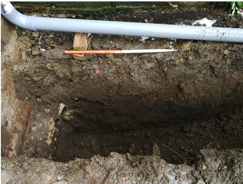
Photograph 4 Excavation of footings for new conservatory view west.
