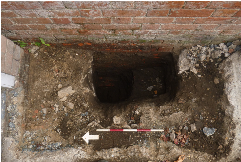
Photograph 3 Excavation of TP3 view east.
