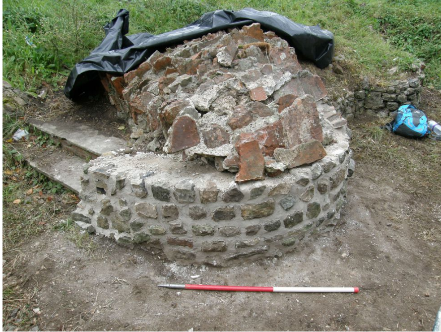
Photograph 4 Masonry during conservation work, showing partial reattachment of tile courses. Photograph taken facing south-west.
