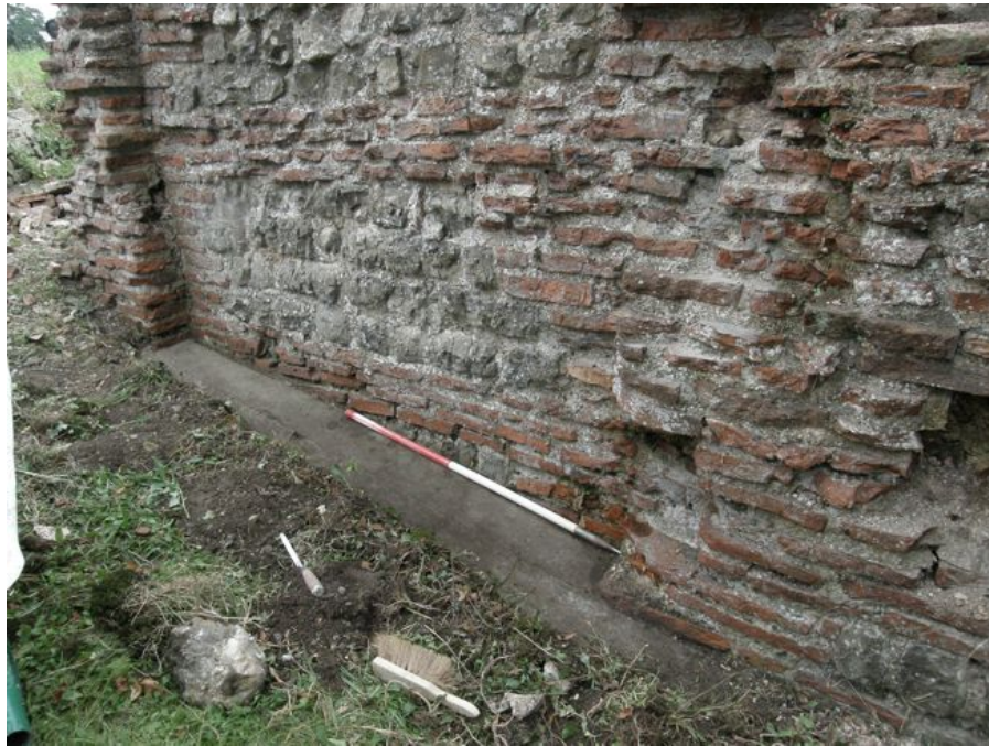
Photograph 8 Concrete drainage channel adjacent to the western side of Duncan's Gate. Photograph taken facing south-west.
