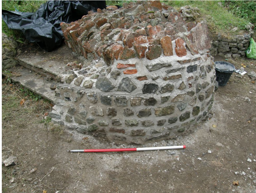
Photograph 6 Collapsed masonry after complete conservation. Photograph taken facing south-west.
