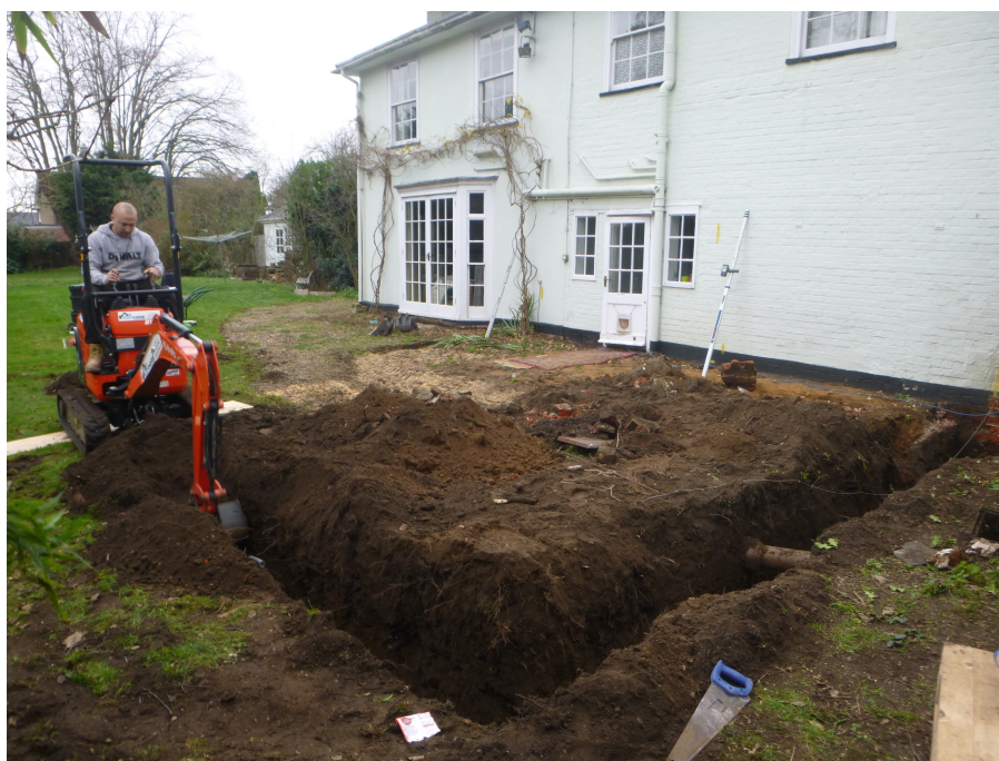
Photograph 1 Foundation trenching for the rear extension, looking northwest
