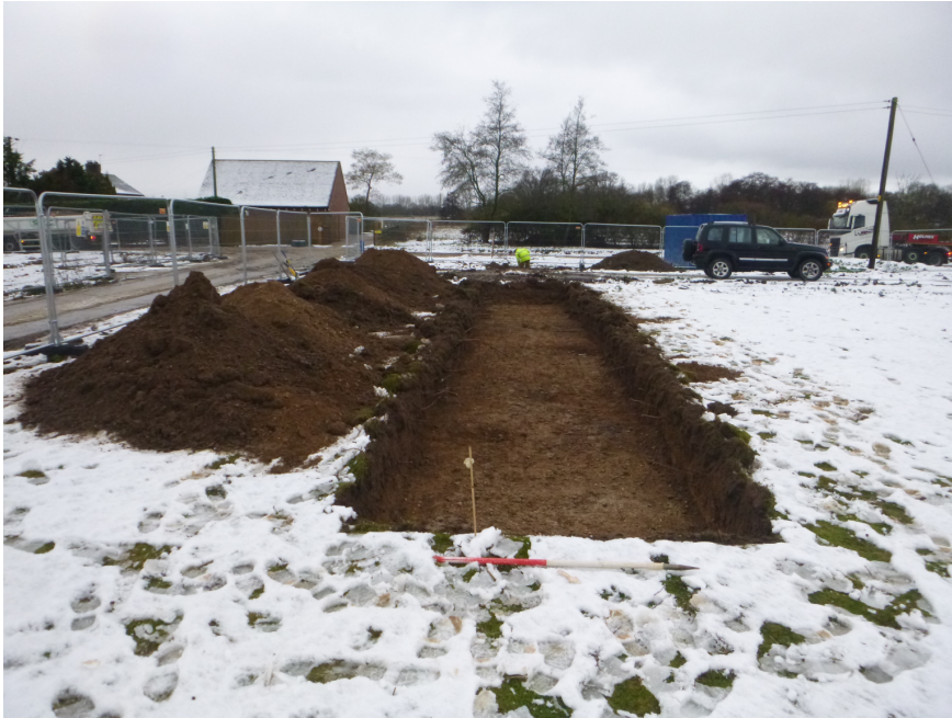
Photograph 2: T6 general shot, looking southwest.
