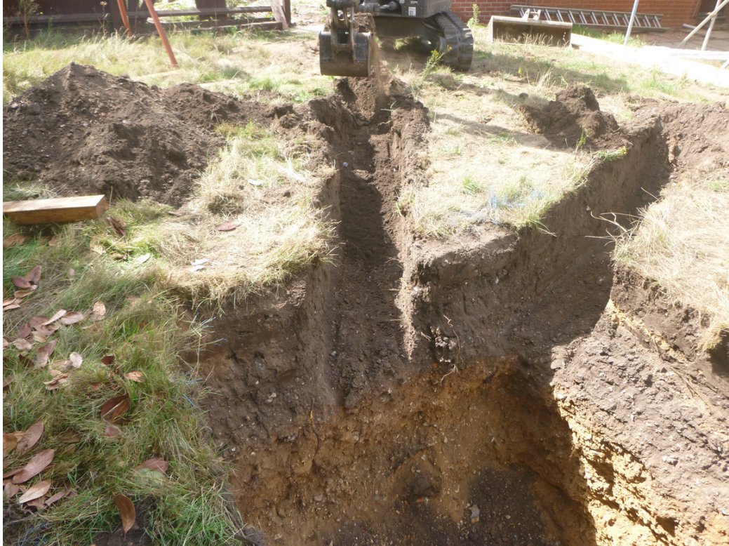
Photograph 2 Soakaway and drainage trenches, looking southwest
