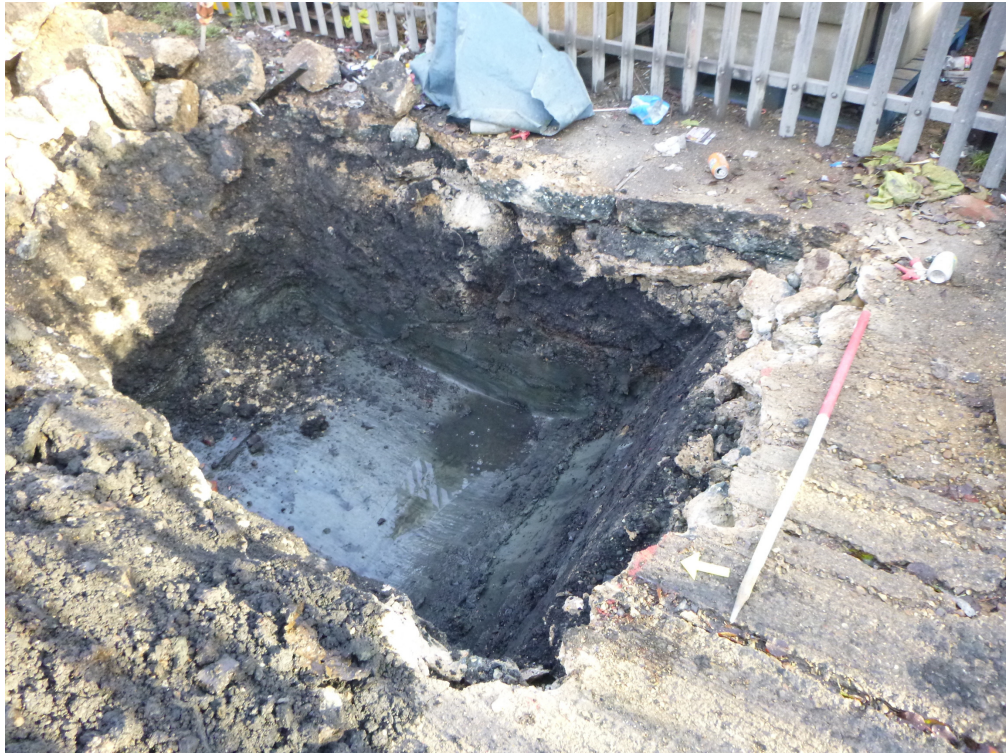
Photograph 1 TP1, looking east northeast
