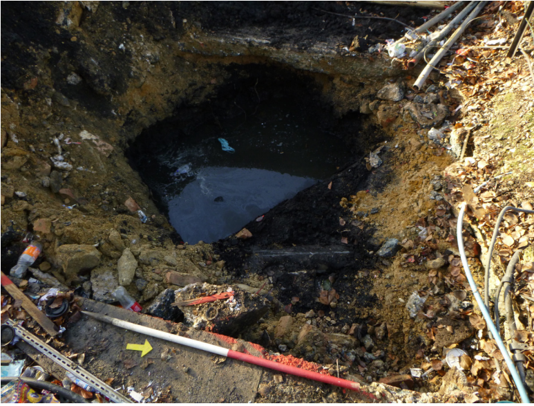
013 TP2 - looking west southwest
