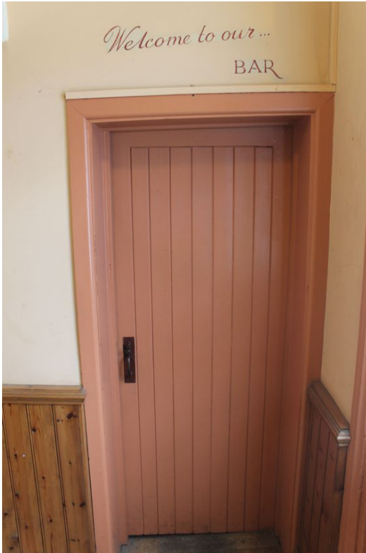
Photograph 16 Vertical-planked door leading into northern bar from foyer. Photograph taken facing north-east.
