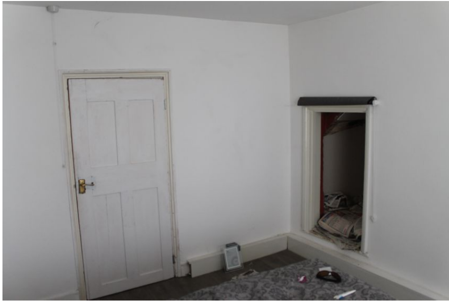
Photograph 23 Interior of northern bedroom in pub, showing original door (to left) and crawl-space into loft of extension A (to right).
