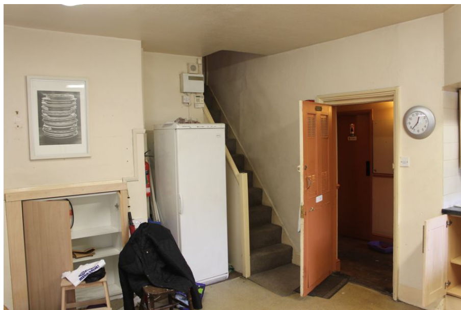
Photograph 20 Interior ground-floor of extension A, showing the blocked fireplace, door into corridor and stairway to first-floor. Photograph taken facing south.
