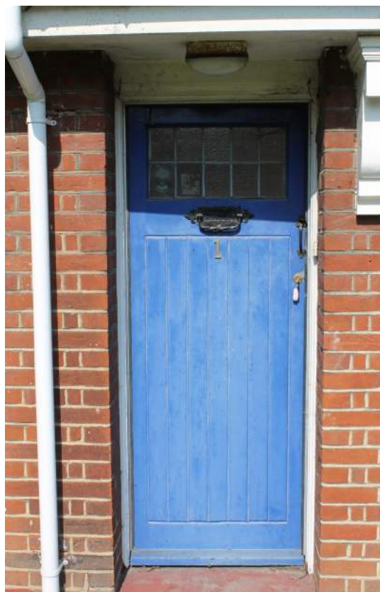
Photograph 4 Original door to No.1 Winnocks – view north-west.
