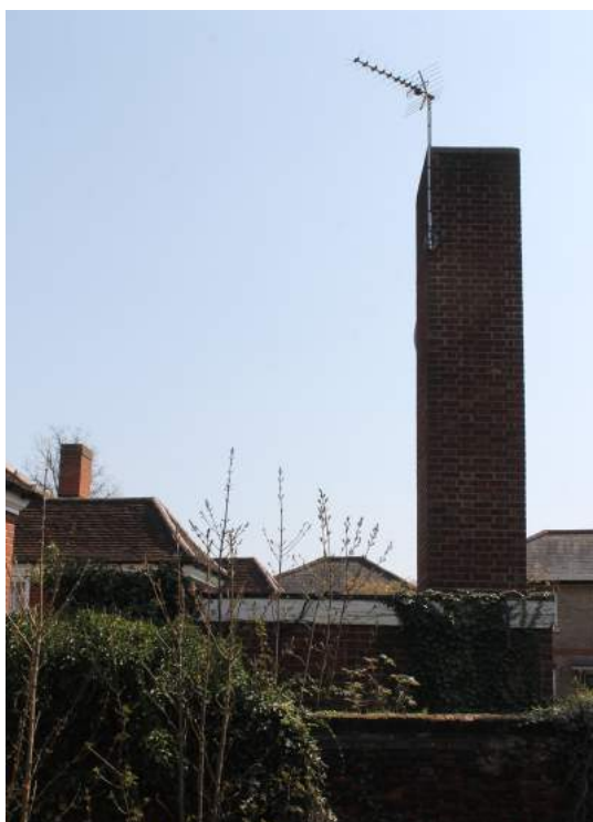
Photograph 24 Boiler house to the rear of the 17th-century range, dating from the early 1970s – view south-east.
