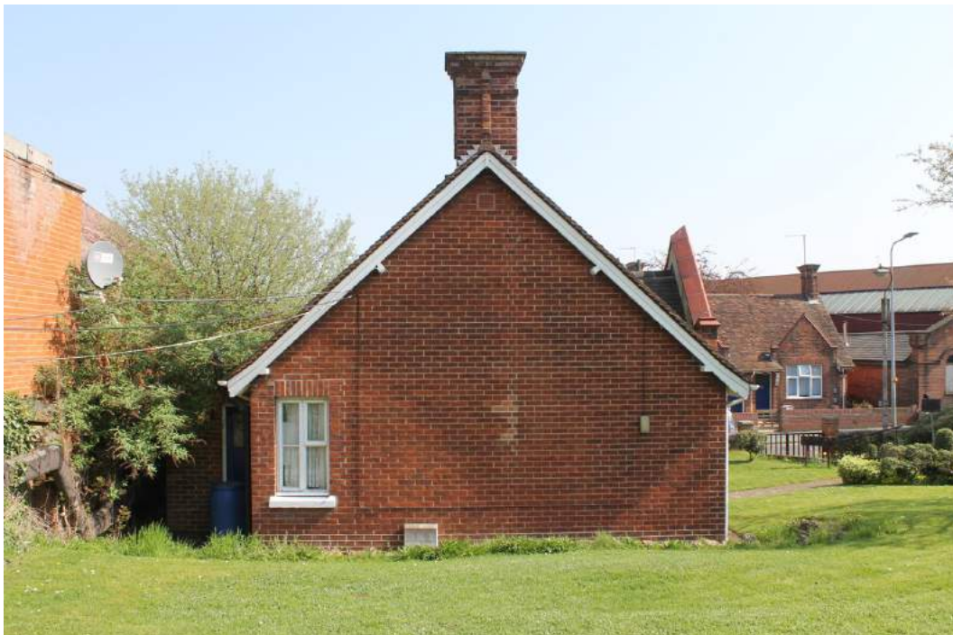
Photograph 6 South-west elevation of No.2 Winnocks, identical to the other gable elevations except for an inserted timber-framed casement – view north-east.
