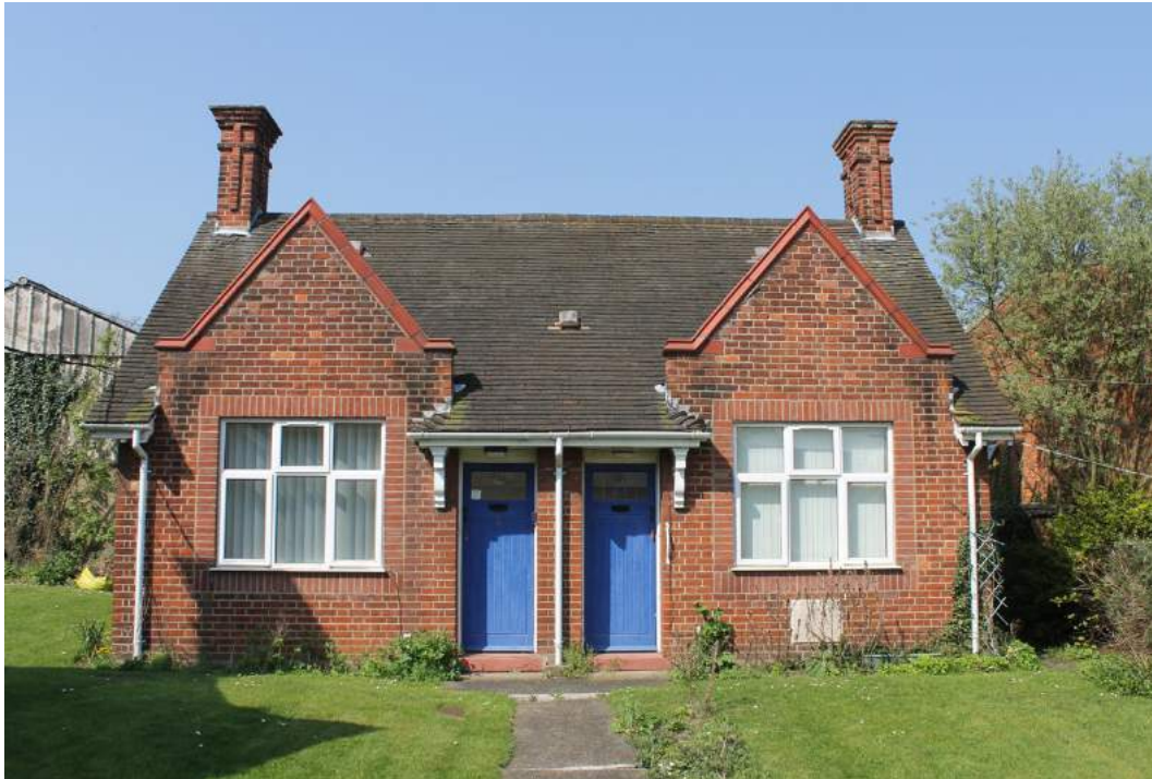
Photograph 3 East elevation of Nos.3-4 Winnocks: the windows are replacement UPVC frames set into a brick surround. The doors appear to be original – view west.
