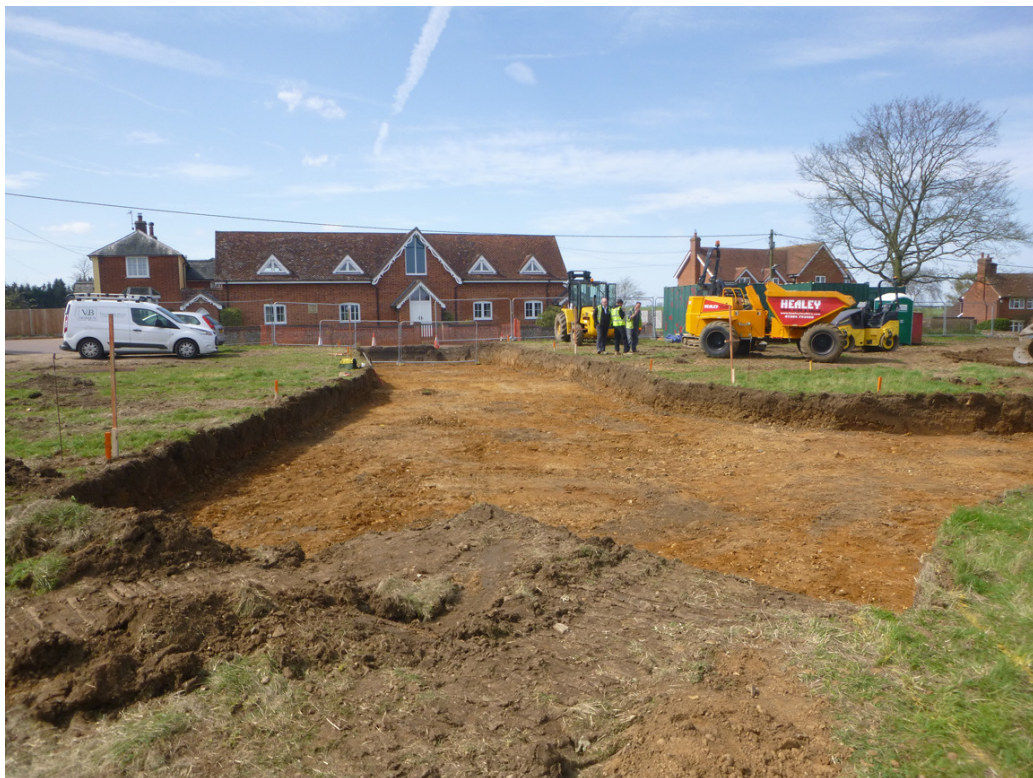
Photograph 1 Access road strip, looking west
