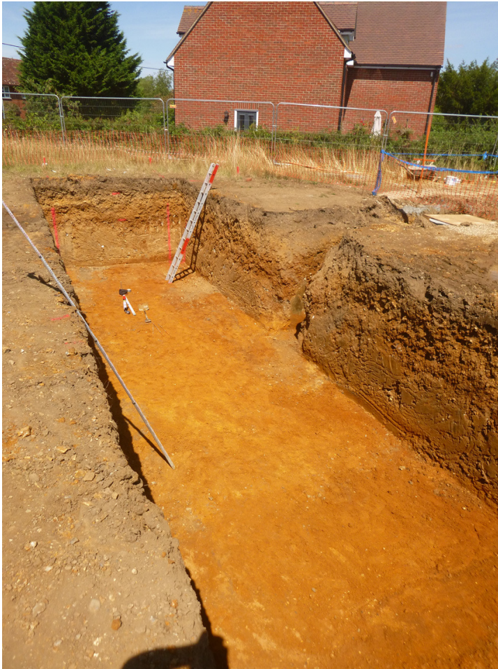
Photograph 4 Attenuation tank fully excavated, looking north
