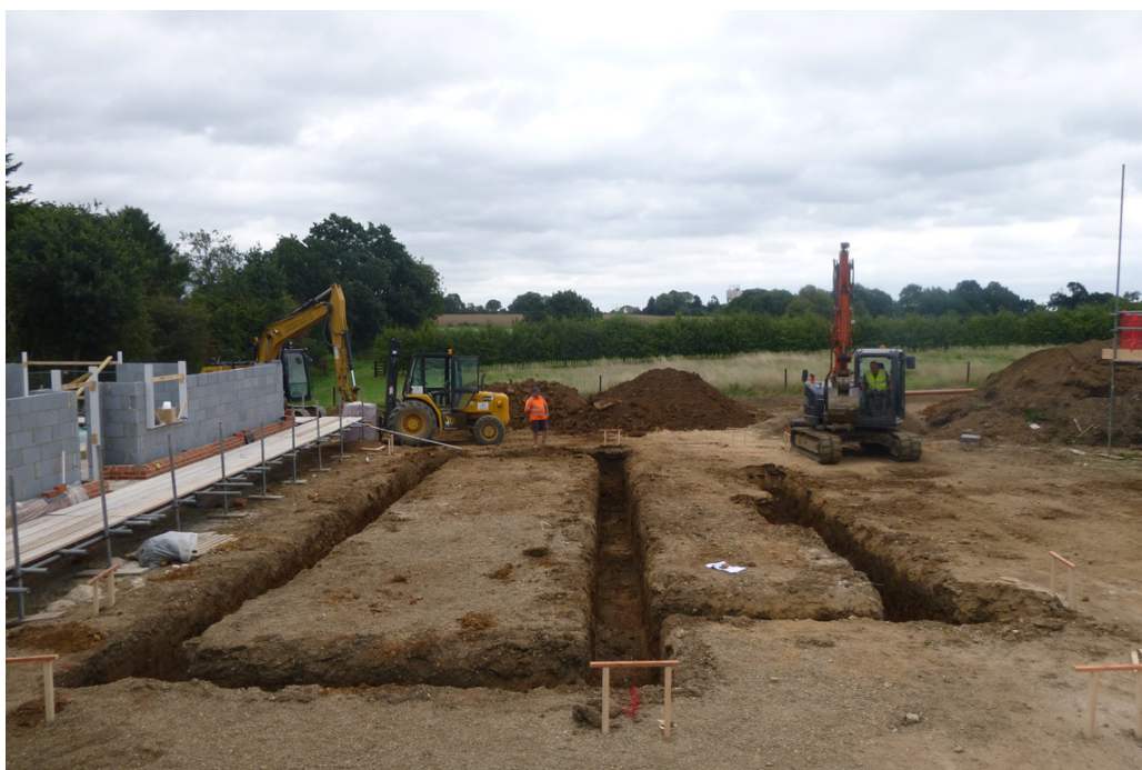
Photograph 2 Foundation trenches, looking east
