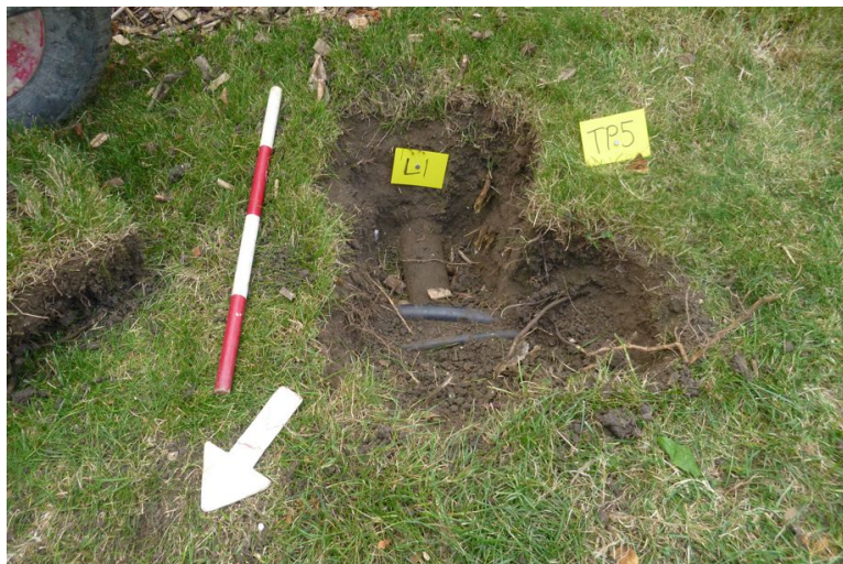
Photograph 6 TP5 after excavation. Oil pipe visible beneath electric cables. Photograph taken facing south-east.
