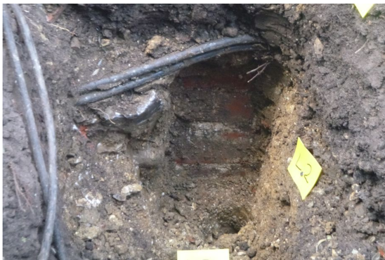
Photograph 3 Detailed shot of red-brick foundation of house (F1) in TP2. Photograph taken facing south-west.
