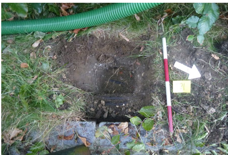
Photograph 1 TP1 after excavation. Photograph taken facing south-west.
