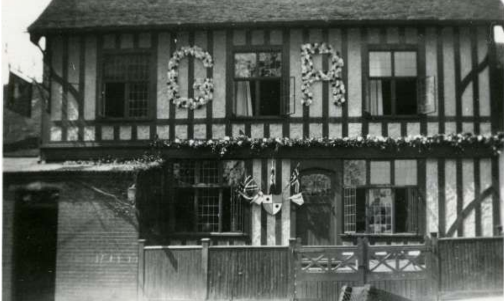
Photograph 5 South-east elevation of Building C, with faux timber-framing and leaded windows. Earlier frontage has been removed entirely, as attested by the visible fascia (compare to Photograph 1 and 2). Hotel is decorated to celebrate the coronation of George VI, which dates the photograph to 1937. Taken from www.merseamuseum.org.uk .
