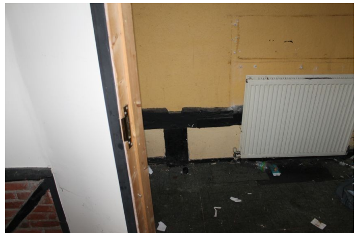
Photographs 25 and 26 Empty lap-joints on south-east (left) and north-west (right) walls of Structure A that would have supported the original binding-beam and floor.
