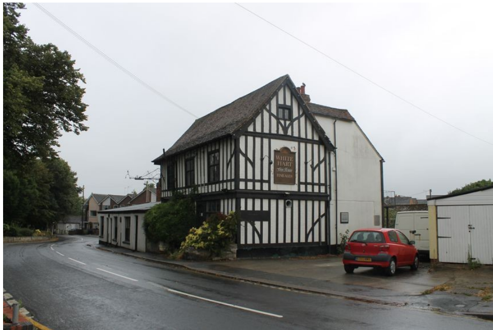
Photograph 12 North-east elevation of the White Hart. Photograph taken facing south-east.
