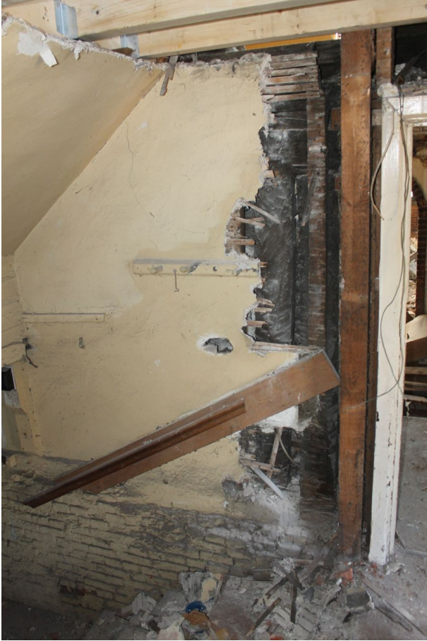
Photograph 53 Partially exposed sill-beam and reused studs behind fireplace in Structure A, supported on the 16th century cellar walls. Photograph taken facing south-east.
