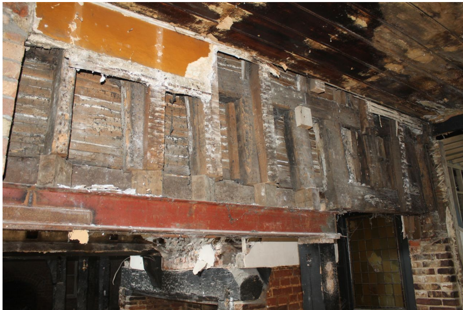
Photograph 42 Exposed partially surviving studs and girding-beam on south-east elevation of Structure A after soft strip. Photograph taken facing north.
