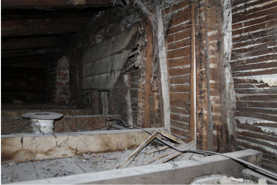
Photograph 45 Upper register of Structure A's south-east elevation, showing surviving weatherboarding. Photograph taken facing west.
