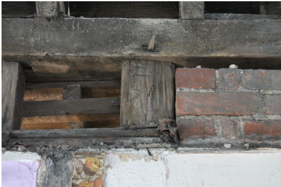
Photograph 57 Detail of carpenter's mark "VII" on stud/storey-post in north-west elevation of Structure C. Photograph taken facing north-west.
