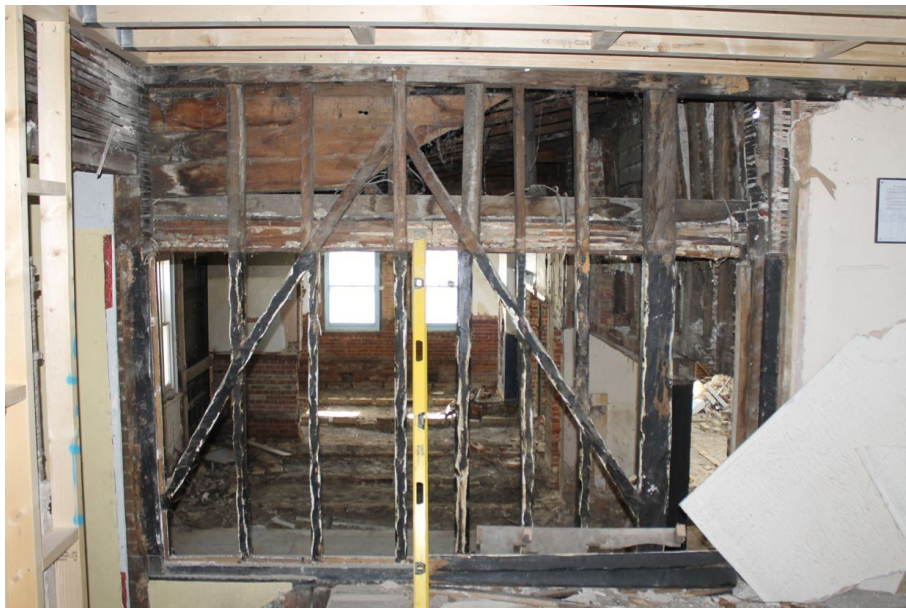
Photograph 59 Timber-framing in north-east end of Structure F, showing machine-cut timbers that have been altered to appear hand-sawn. Photograph taken facing south-west.
