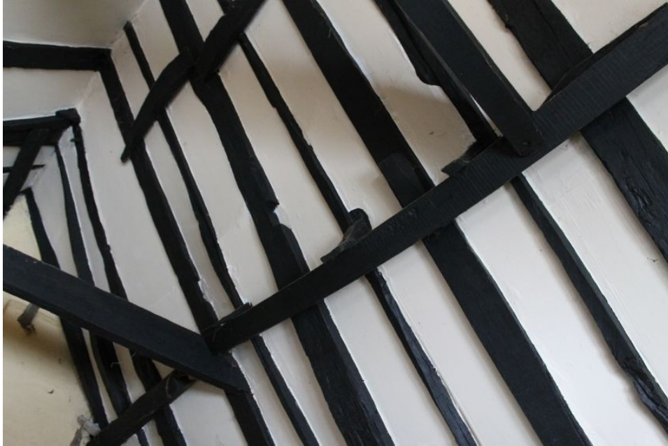
Photograph 24 North-west pitch of Structure A's roof. Showing later bracing, collars and purlin. Photograph taken facing west.
