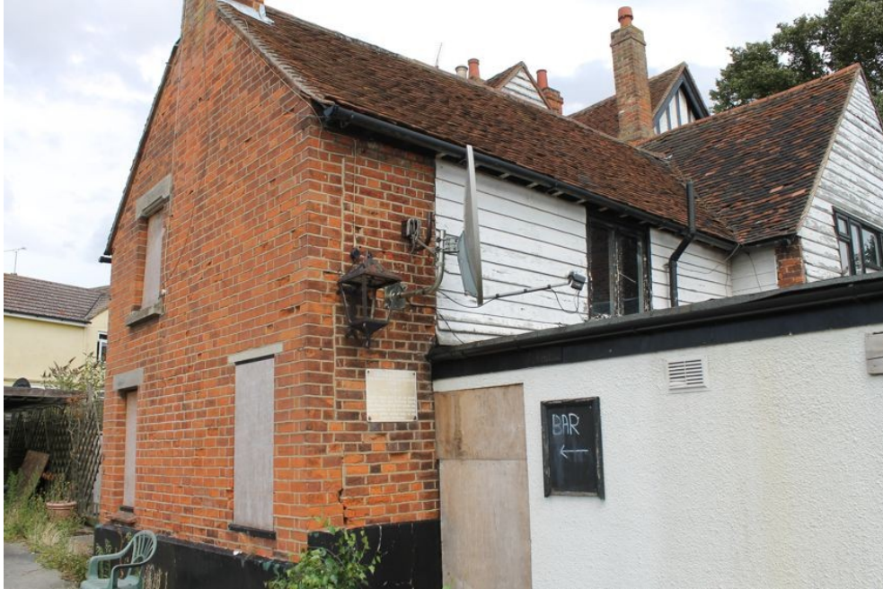
Photograph 9 North-west and south-west elevations of Structure B, showing mismatched brickwork adjacent to timber-frame. Photograph taken facing east.
