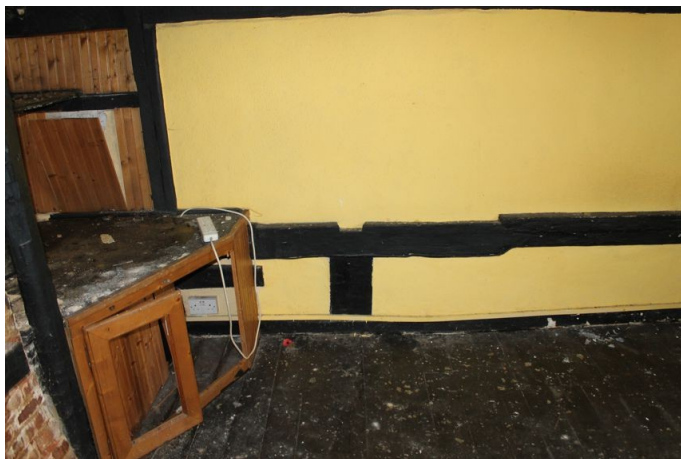
Photographs 25 and 26 Empty lap-joints on south-east (left) and north-west (right) walls of Structure A that would have supported the original binding-beam and floor.
