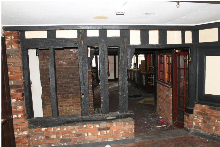
Photograph 18 Original stud-work viewed from Structure B. Inserted modern timber clear, as is original header for doorway. Photograph taken facing south-east.
