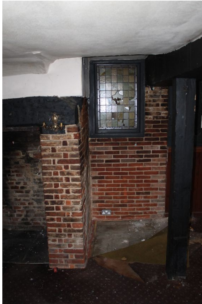
Photograph 16 North-east ground-floor wall to Structure A, showing inserted brickwork and stained-glass window. Photograph taken facing north-east.
