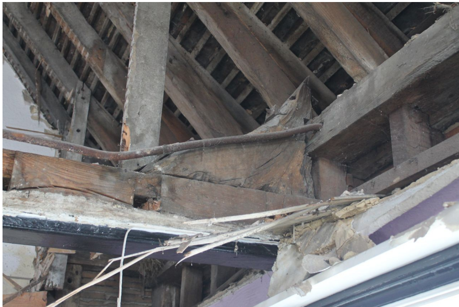
Photograph 55 Detail of inverted knee brace on south-eastern end of the northernmost tie-beam in Structure C. Photograph taken facing north-east.
