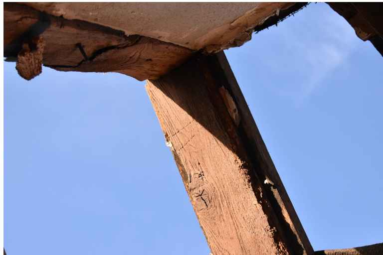
Photograph 62 Detail of carpenter's mark "II" on western rafter of Structure A. Photograph taken facing west.
