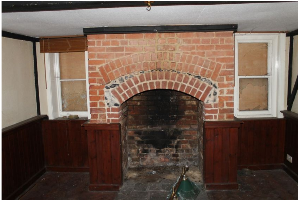
Photograph 27 Repaired fireplace on north-west ground-floor elevation of Structure B. Photograph taken facing north-west.
