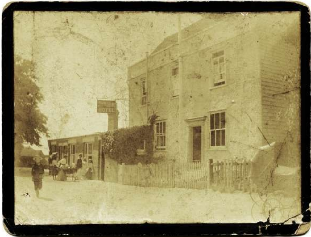
Photograph 1 Early 20th-century photo showing the original frontage of Structure C with no faux timber-framing. There are sash windows on its south-eastern face, and weatherboarding on its north-eastern face. The lack of extension of the adjacent building to the north (see Photograph 2) dates this photo to some point pre-1920. Taken from www.merseamuseum.org.uk .
