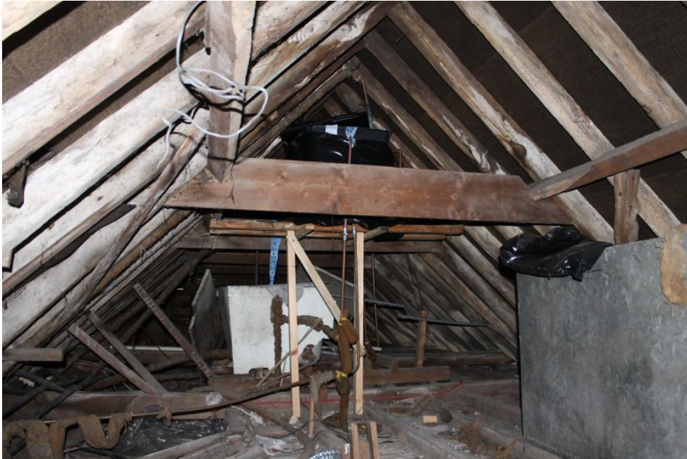
Photograph 36 Roof structure of Structure D. Photograph taken facing south-west.
