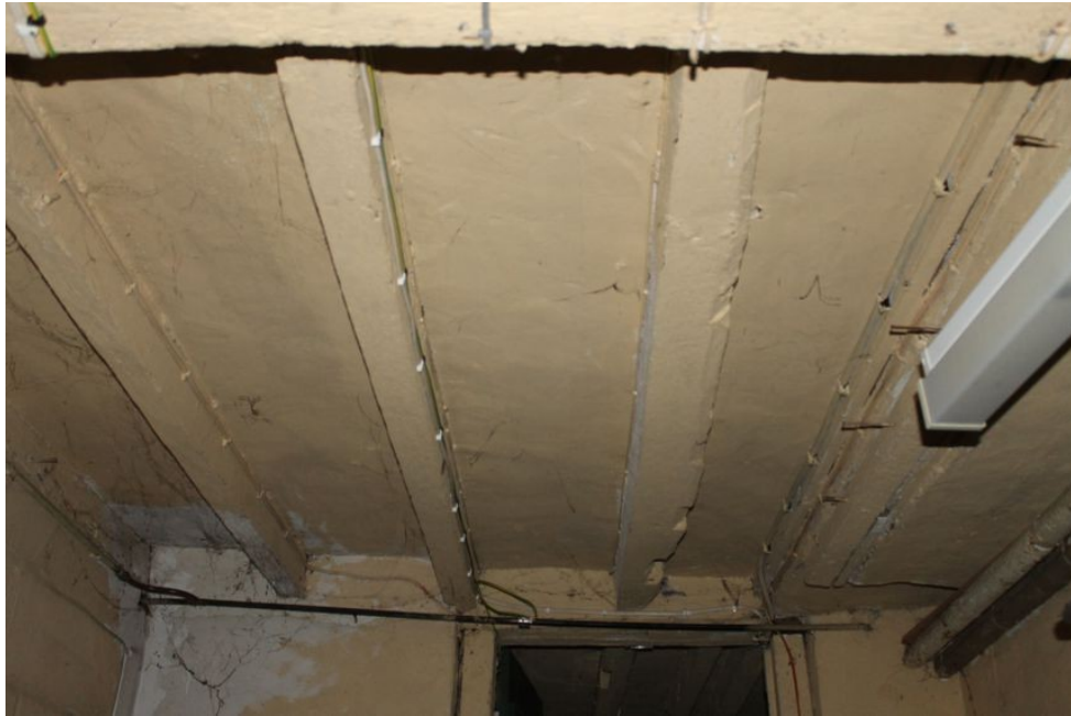
Photograph 31 Underside of ground-floor of Structure C, observed from cellar. Re-used timbers visible. Photograph taken facing north-west.
