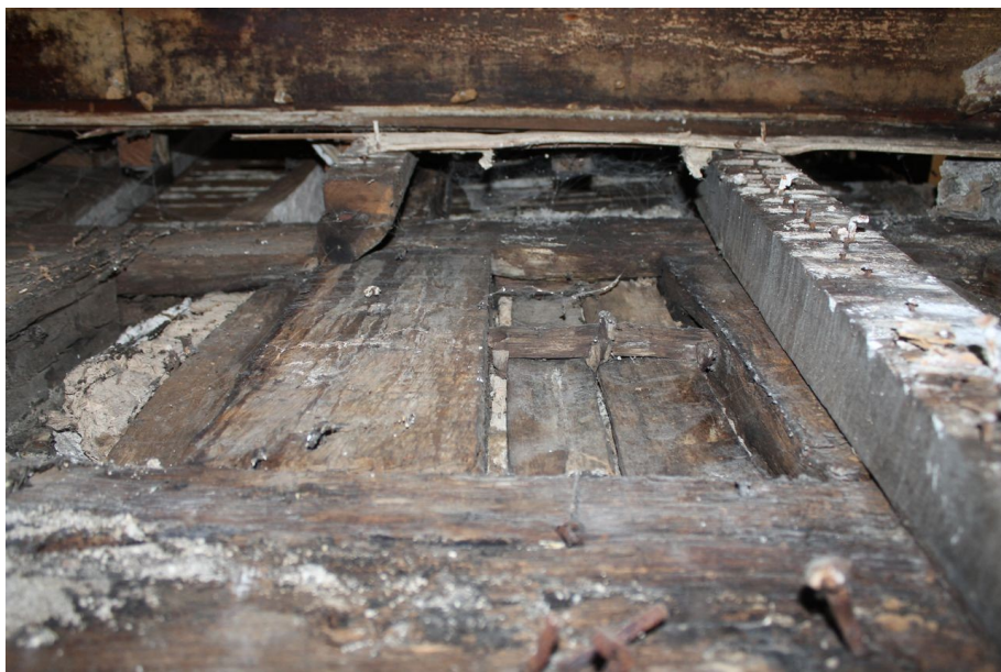
Photograph 44 Detail of timber panelling infill on south-east elevation of Structure A, showing grooves for planks and strap. Photograph taken facing north-west.
