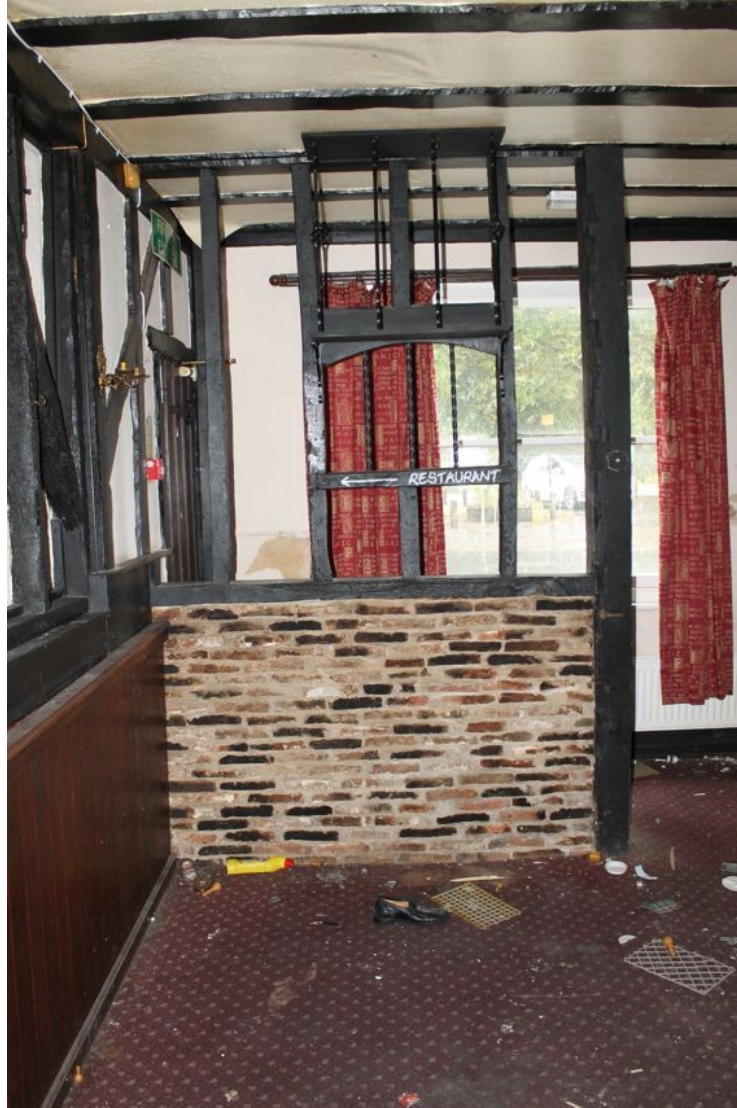
Photograph 39 Modern wall in Structure F consisting of re-used bricks and a re-used tie-beam (to right). Photograph taken facing south-east.
