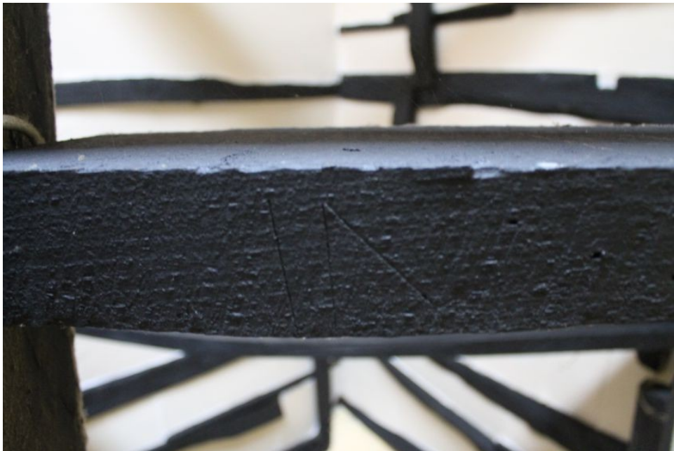
Photograph 23 Detail showing carpenter's mark "VI" on underside of brace to collar-purlin.
