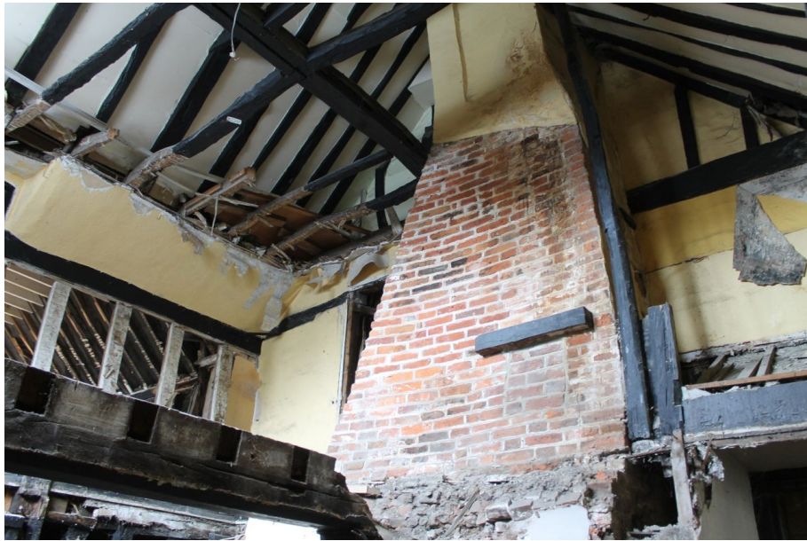
Photograph 41 Chimney-stack in Structure A after soft strip. Photograph taken facing north.
