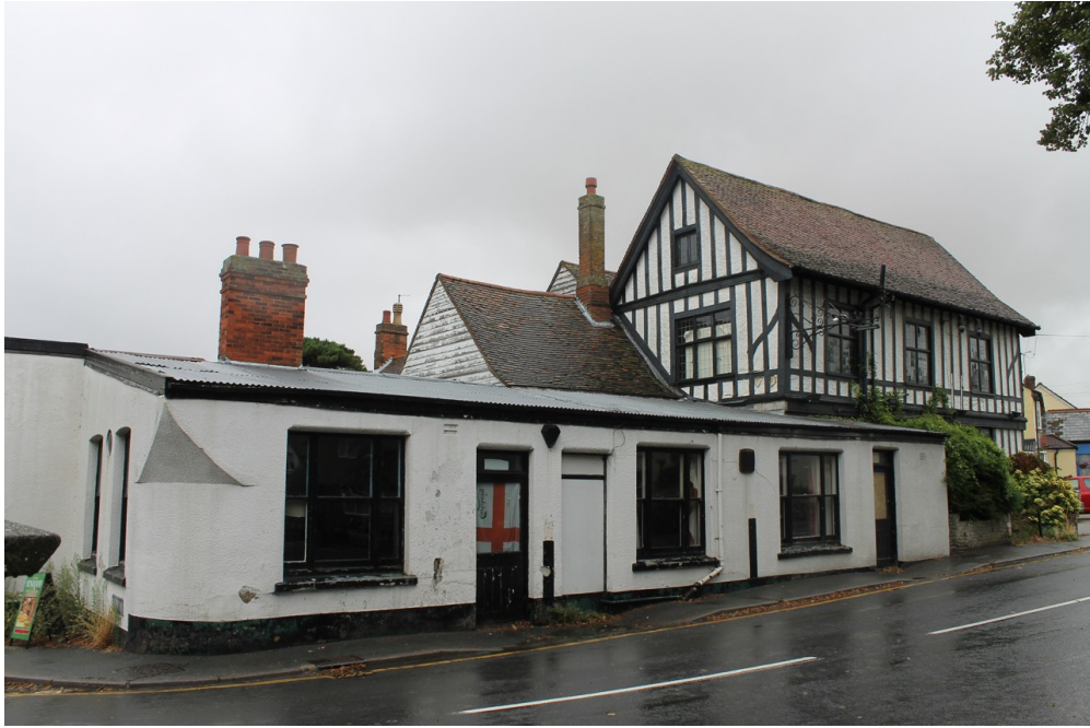
Photograph 7 The White Hart as it is today. South-east elevations of Structures C and F visible. Photograph taken facing north.
