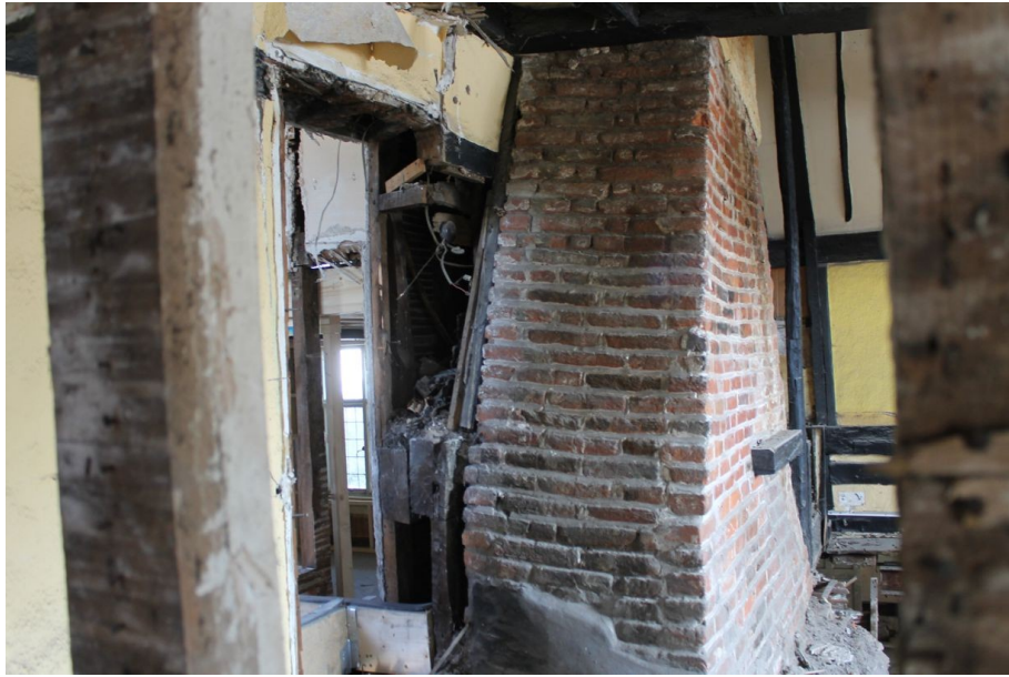
Photograph 49 Detail of north-west side of chimney stack, showing beams and surviving plaster behind in Structure A. Photograph taken facing east.
