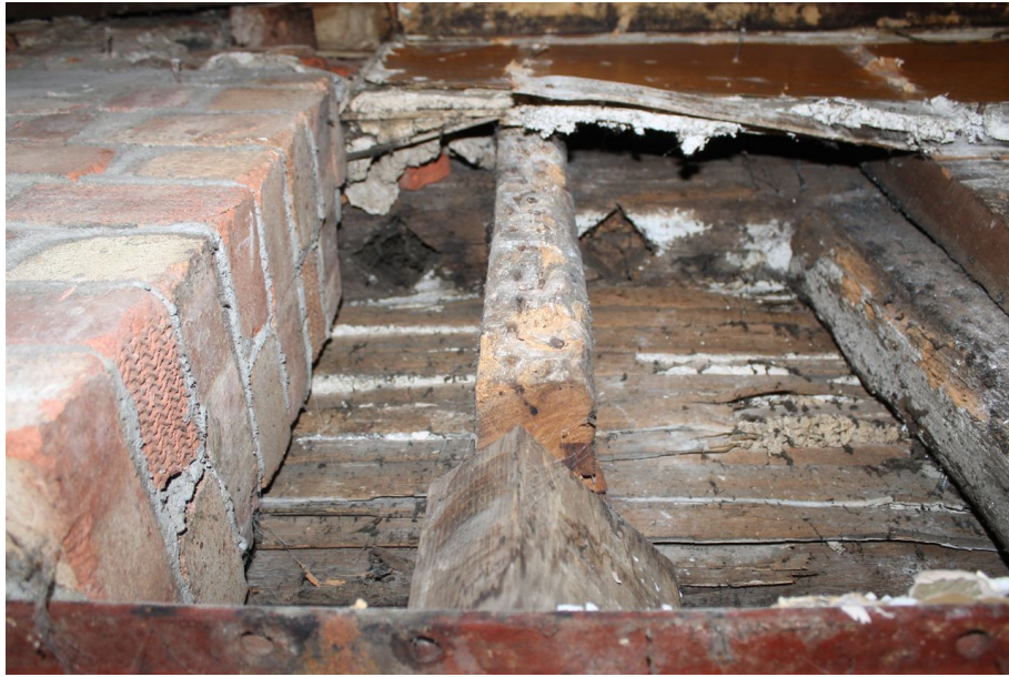
Photograph 47 Detail of diamond mullion mortices on underside of Structure A's south-east girding-beam. Photograph taken facing north-west.
