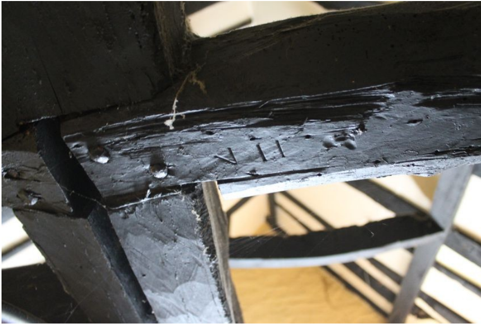
Photograph 22 Detail showing carpenter's mark "VII" on underside of brace to collar-purlin. Photograph taken facing north-east.
