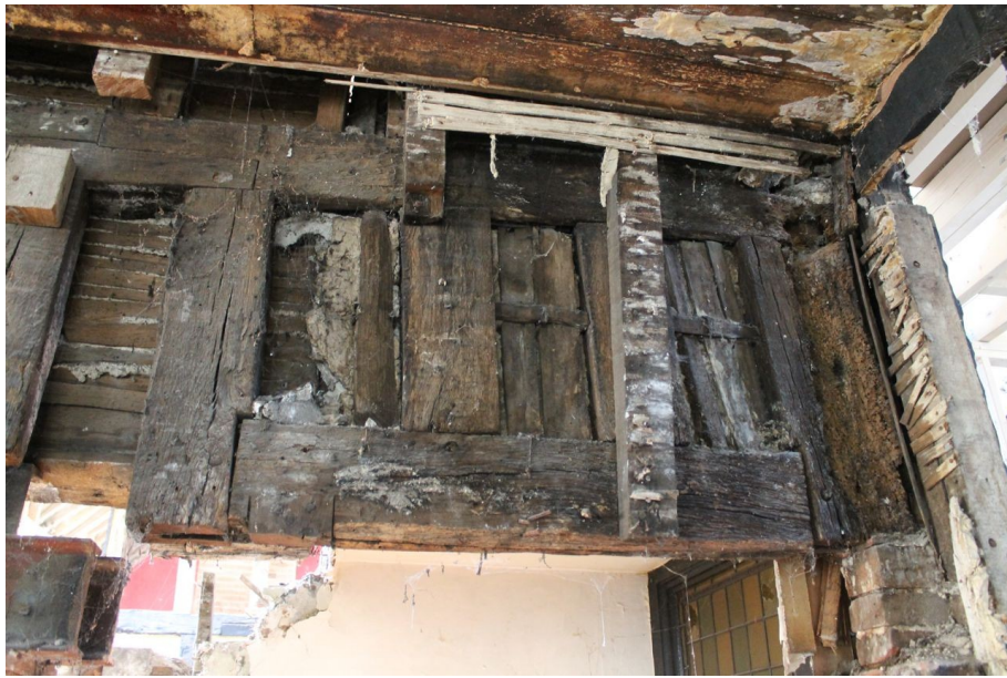
Photograph 43 Detail of timber panelling infill on south-east elevation of Structure A, above original doorway lintel. Photograph taken facing north-west.
