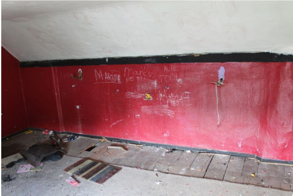
Photograph 28 North-east first-floor elevation of Structure B. Rendered over, but shows end of brickwork (to left) and timber-framing. Photograph taken facing north.
