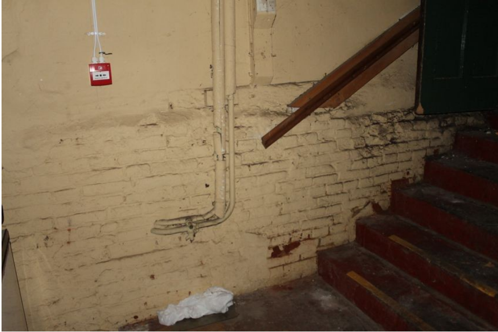
Photograph 29 English-bond brickwork on south-west elevation of cellar, probably associated with Structure A. Photograph taken facing south-west.
