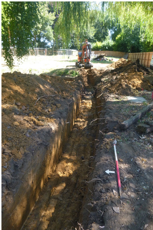
Photograph 1 Service trench, looking east
