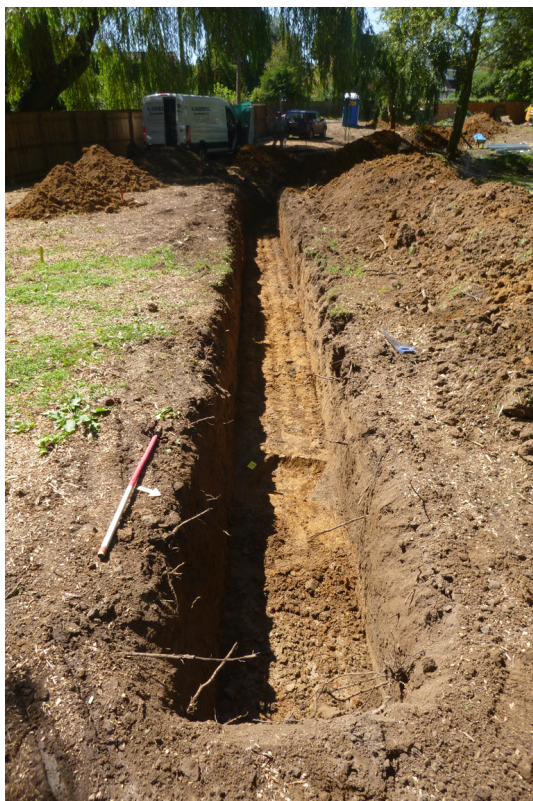
Photograph 2 Service trench, looking west
