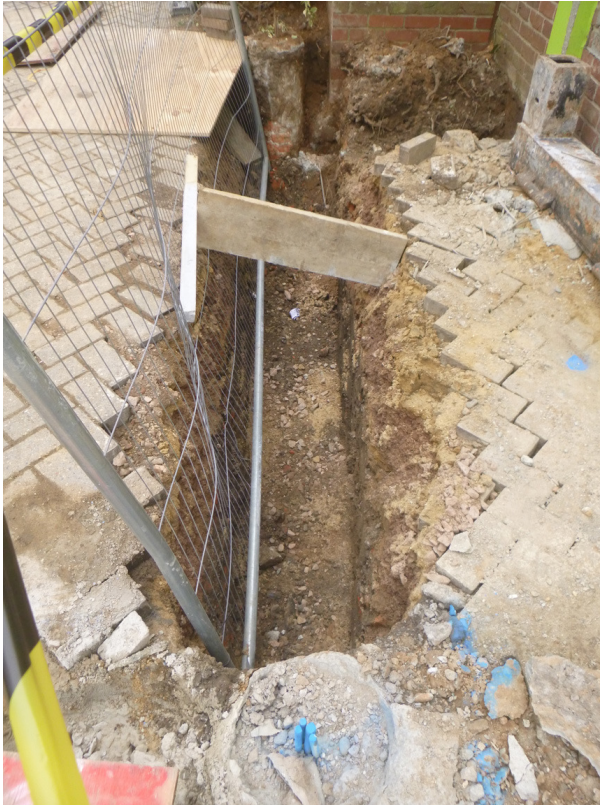
Photograph 4 Trench for the ground beam, looking west
