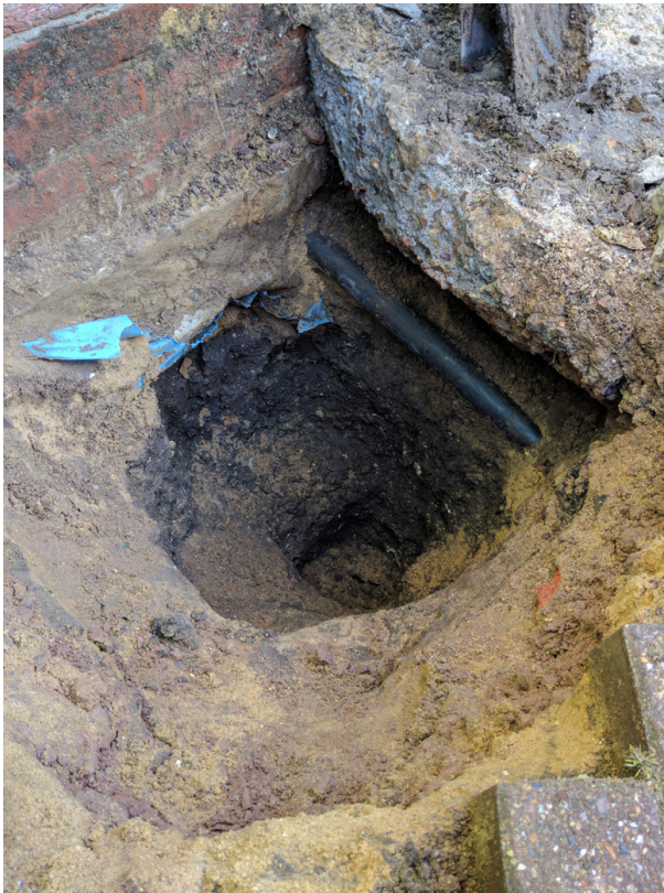
Photograph 1 Test-pit 3, looking northeast
