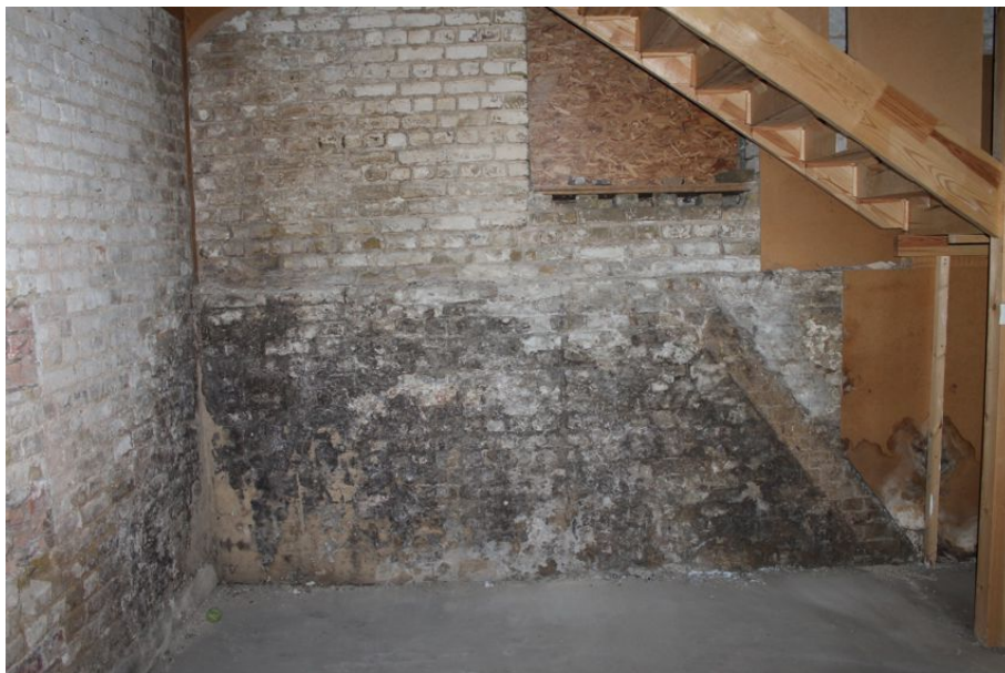
Photograph 86 Visible scarring on brickwork of original staircase in ground-floor of Structure 8. Modern staircase visible to right of frame. Photograph taken facing west.
