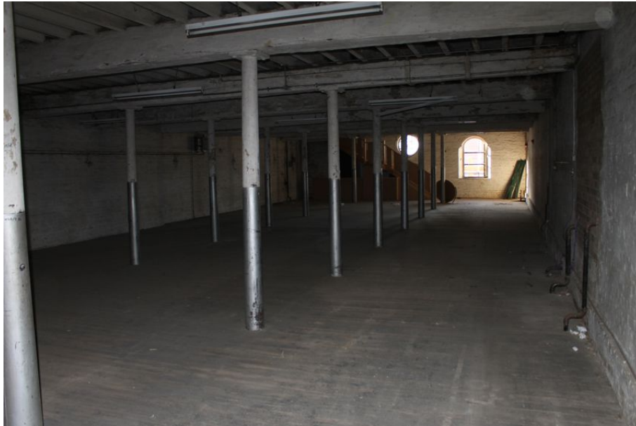
Photograph 89 First-floor of Structure 8. Photograph taken facing south-west.
