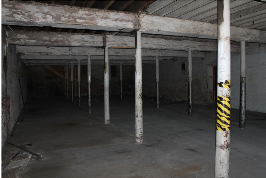
Photograph 85 Ground-floor of Structure 8. Photograph taken facing north-west.
