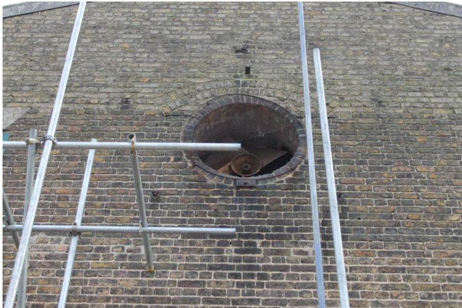
Photograph 70 Inserted metal fan with brick-surround on west elevation of Structure 7. Photograph taken facing east.
