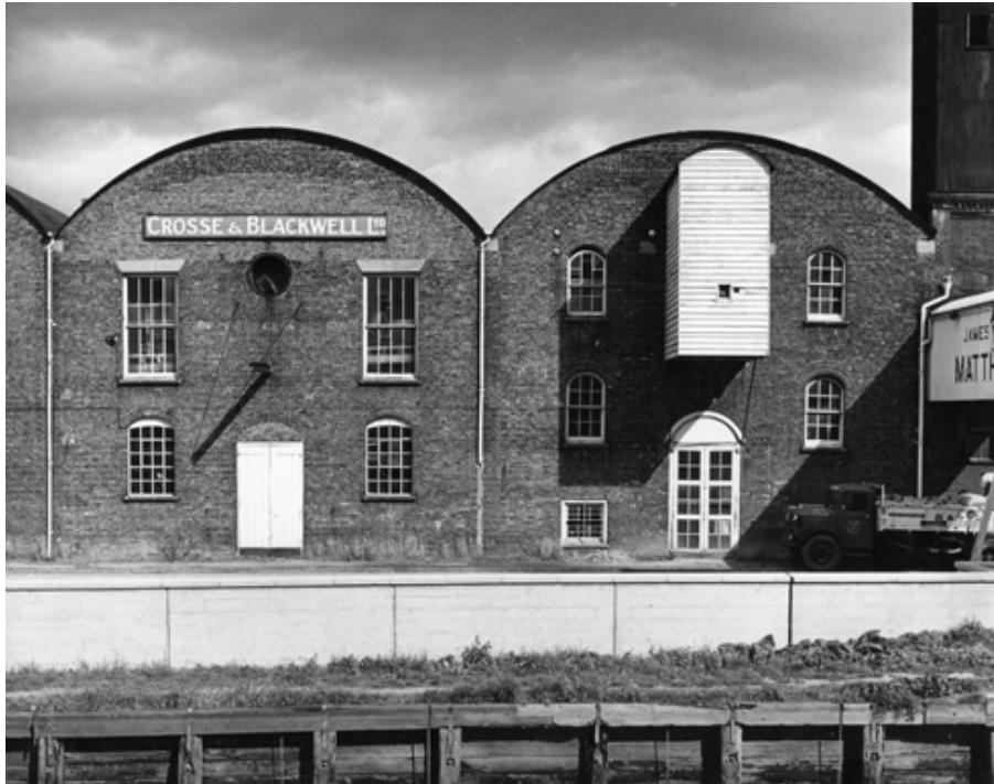
Photograph 4 West elevation of warehouses in 1956 (Structures 7 and 8), showing original barrel roofs. Shows warehouses were occupied by Crosse and Blackwell Ltd. Also visible is the lift on the frontage of Structure 8. The large chimney in the top right, rising from the adjacent warehouse, is much taller than it is today.
