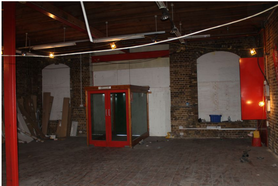
Photograph 75 Eastern end of ground-floor of Structure 7. Photograph taken facing north-east.
