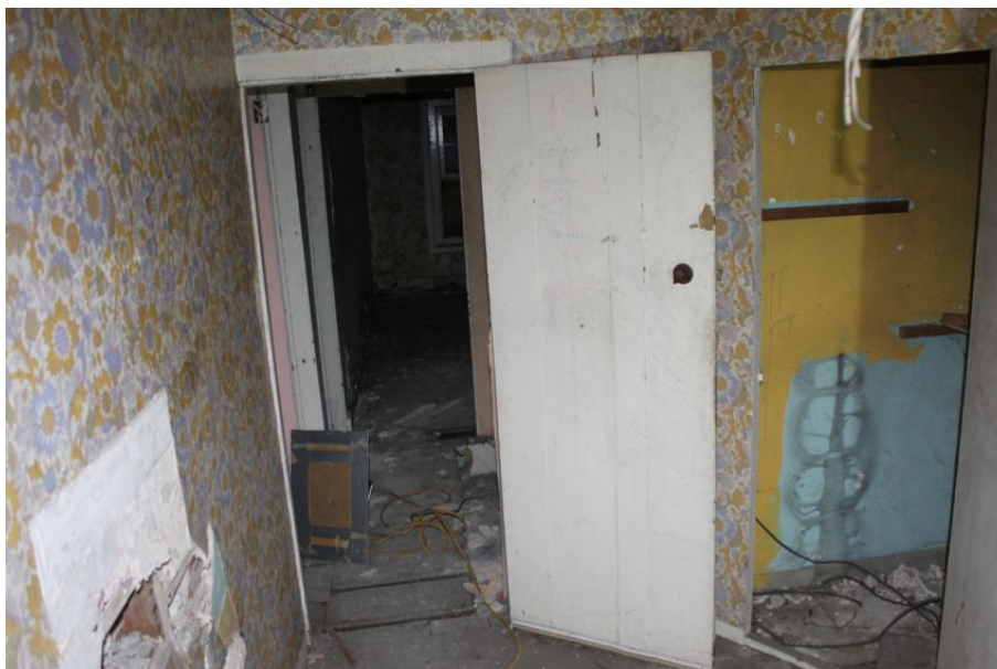
Photograph 32 Vertical-planked door on first-floor of the house extension. Photograph taken facing north-west.
