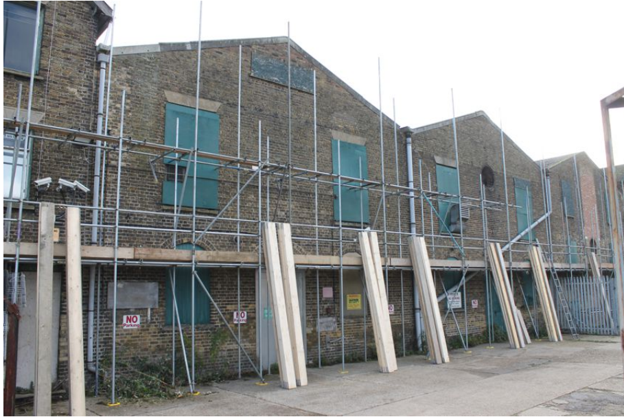
Photograph 56 Western elevation of range of warehouses. Structure 6 to left, Structure 8 to right. Photograph taken facing south-east.
