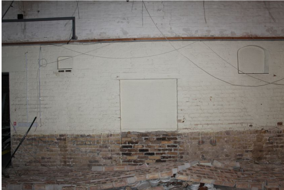
Photograph 62 Original entrance with arch between Structures 6 and 7 at ground-floor level, now bricked over. Photograph taken facing north.
