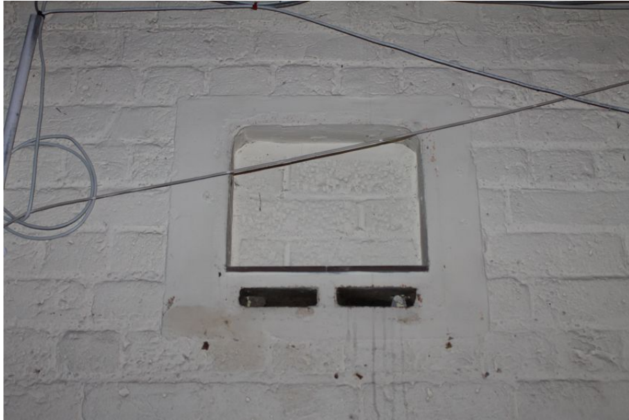
Photograph 74 Possible ?gas-light holder in northern brickwork on ground-floor of Structure 7. Photograph taken facing north.
