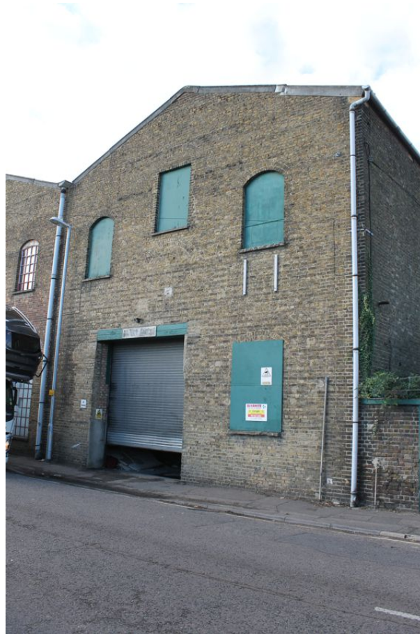
Photograph 53 Eastern elevation of northern warehouse (Structure 6). Photograph taken facing south-west.
