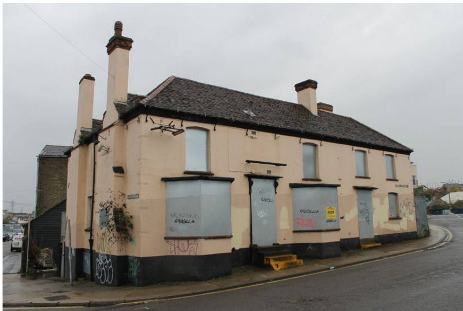
Photograph 5 North-west and north-east elevations of the Rising Sun (left of frame; Structure 1) and the house extension (right of frame; Structure 2). Photograph taken facing south.
