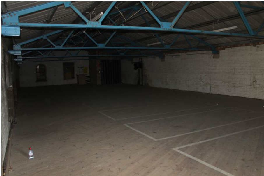
Photograph 90 Second-floor of Structure 8. Photograph taken facing south-east.
