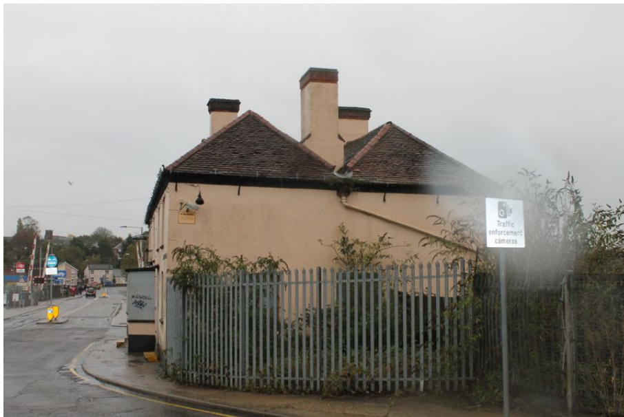
Photograph 20 South-west elevation of the house extension (Structure 2). Photograph taken facing east.
