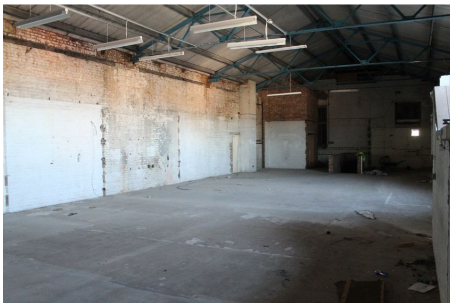
Photograph 65 First-floor of Structure 6. Photograph taken facing south-west.
