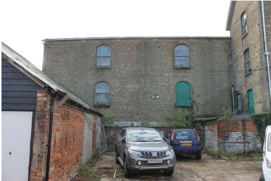
Photograph 36 Northern elevation of Structure 6 (northern warehouse). Also shows Structure 4 to right of frame. Photograph taken facing south.
