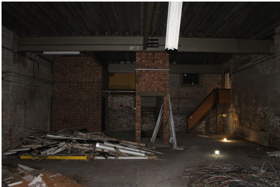
Photograph 59 Inserted modern features in western end of Structure 6's ground-floor. Stairway leading down from first-floor to external door visible in centre. Staircase up to first-floor of Structure 5 visible to right. Photograph taken facing west.
