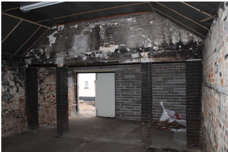
Photograph 35 Internal division within Structure 3, showing brick pillars. Cement block wall visible behind. Photograph taken facing north-west.
