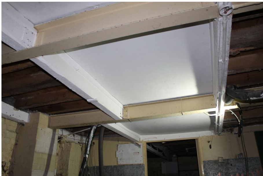
Photograph 11 Modern beams, both timber and metal, supporting the ground-floor of the Rising Sun. Photograph taken facing east.
