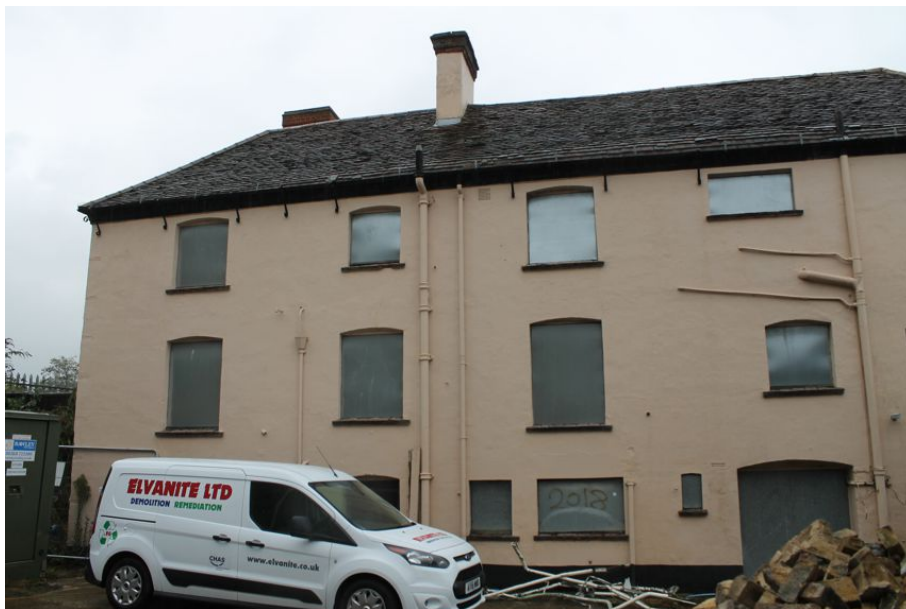
Photograph 7 South-west elevation of the Rising Sun (right of frame; Structure 1) and the house extension (left of frame; Structure 2). Photograph taken facing north-west.
