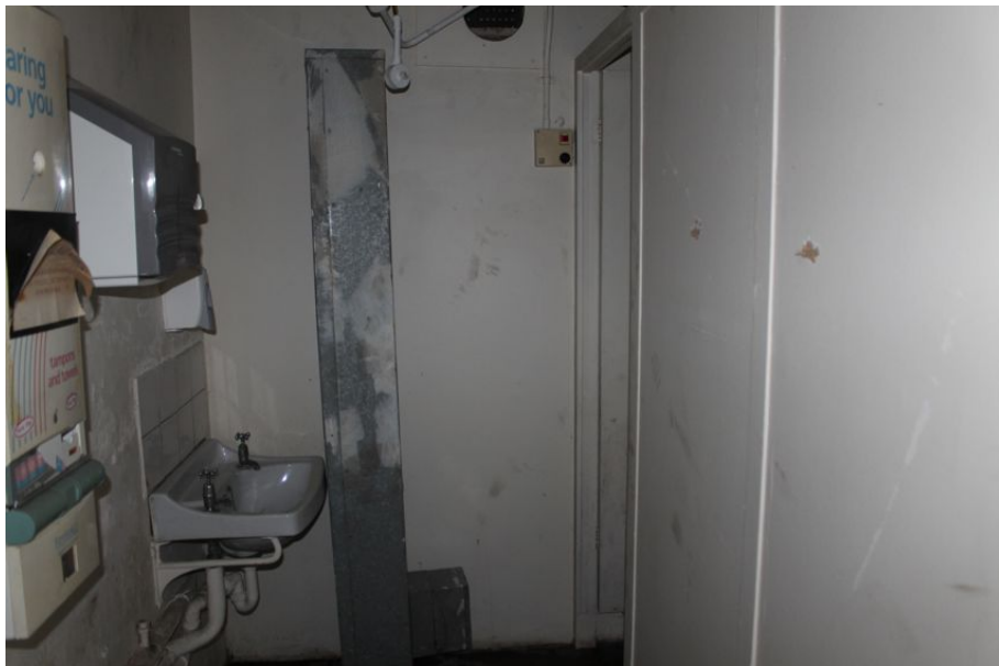
Photograph 37 Interior of Structure 4. Photograph taken facing north.
