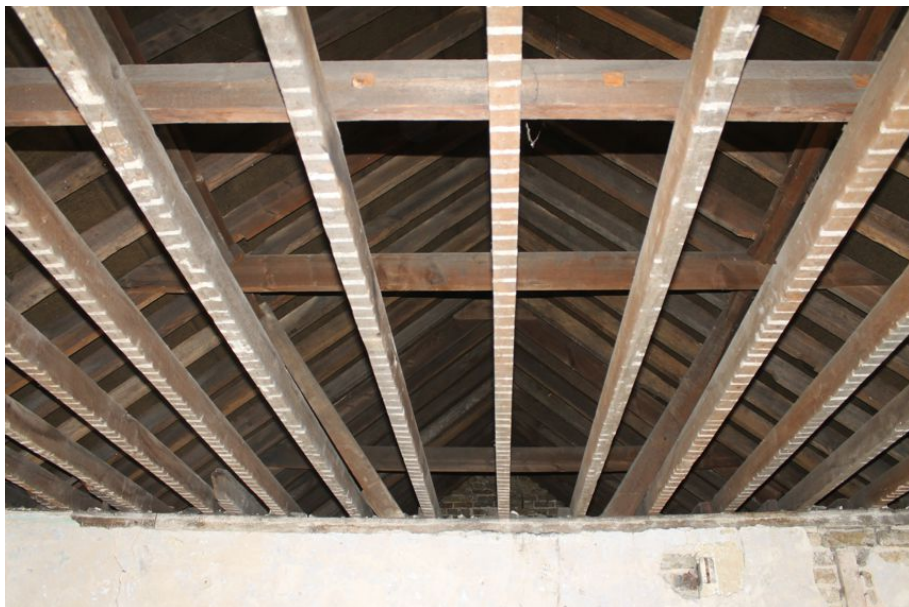
Photograph 51 Timber roof of Structure 5. Photograph taken facing west.
