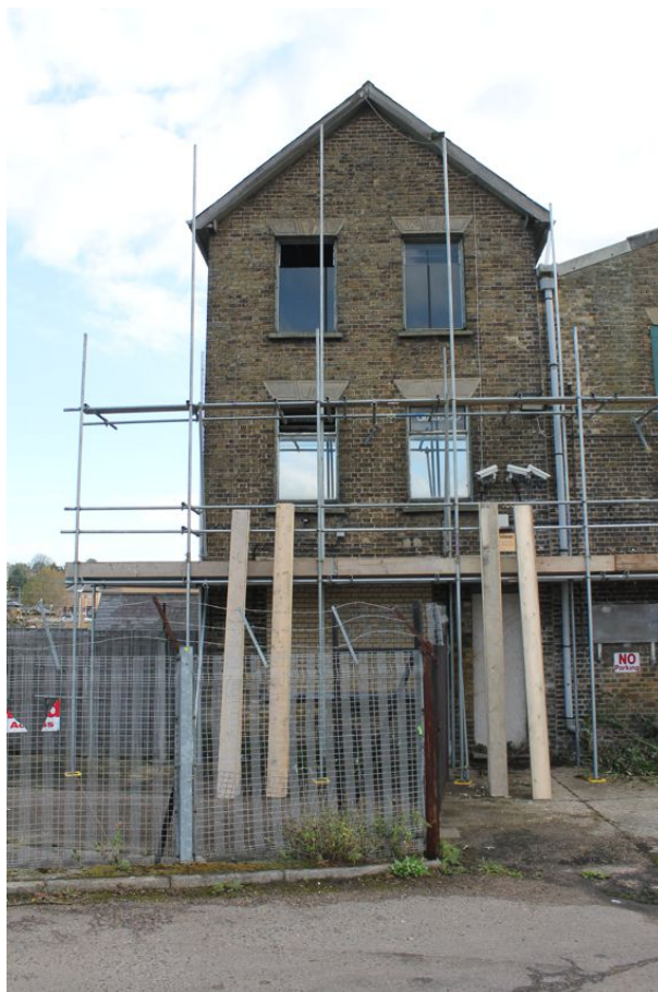
Photograph 40 Western elevation of Structure 5. Photograph taken facing east.
