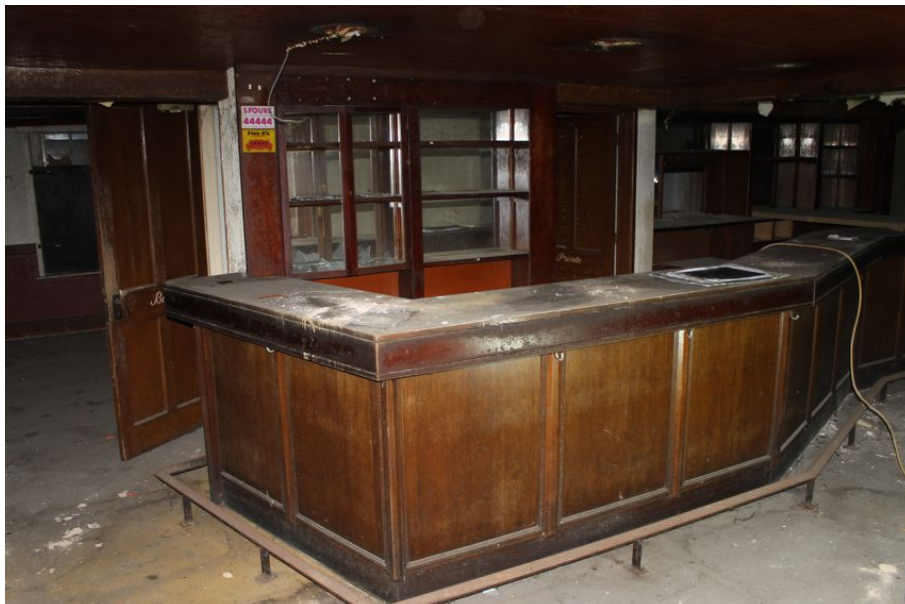
Photograph 13 Modern bar inserted into ground-floor of Rising Sun. Photograph taken facing south-west.
