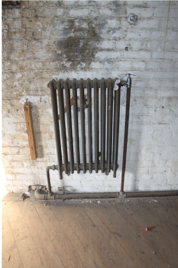
Photograph 91 Inserted radiator on second-floor of Structure 8. Photograph taken facing north.
