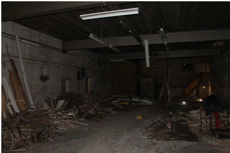
Photograph 57 Ground-floor of Structure 6. Photograph taken facing south-west.
