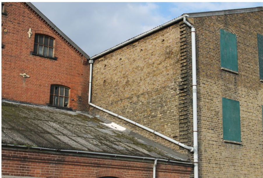
Photograph 83 South elevation of Structure 8. Projecting bricks visible. Photograph taken facing north-west.
