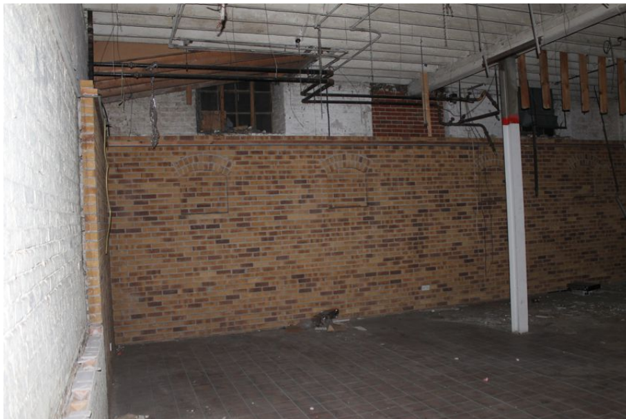
Photograph 72 Modern skin of bricks over original brickwork in western end of Structure 7. Entrance and windows on western elevation also visible. Photograph taken facing north-west.
