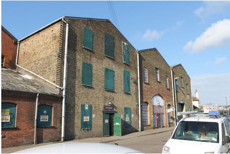
Photograph 66 East elevation of warehouse range. Structure 8 to left, Structure 6 to right. Photograph taken facing north-west.
