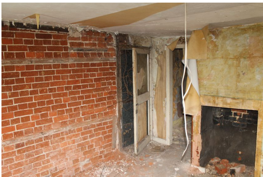
Photograph 28 South-west room on ground-floor of house extension. Showing external entrance, fireplace and exposed brickwork. Photograph taken facing north-west.
