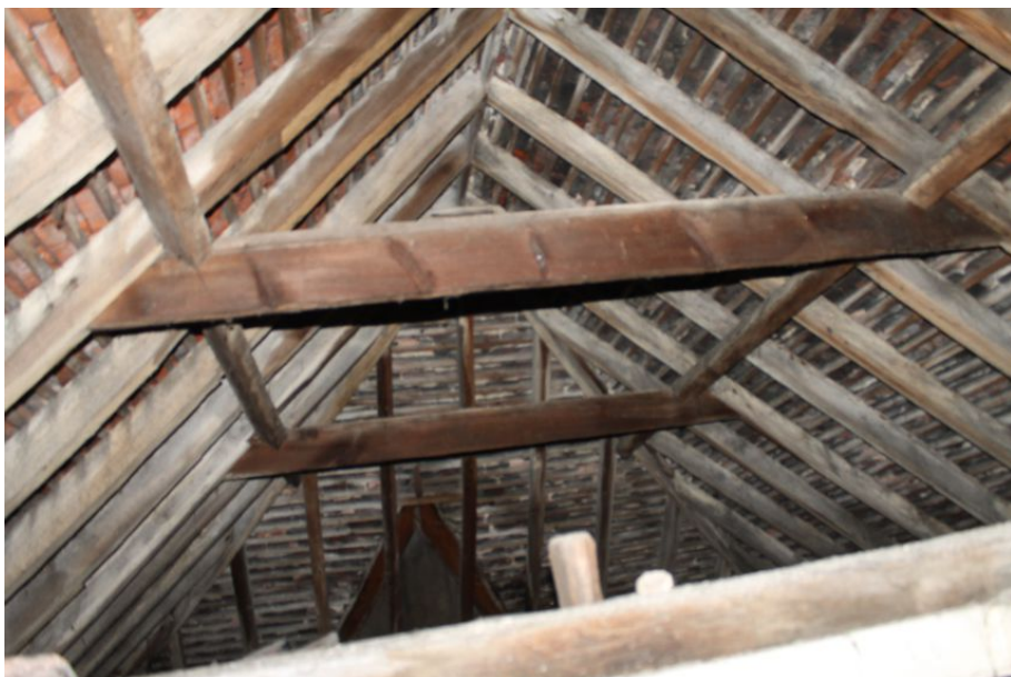
Photograph 19 Roof structure above southern range of Rising Sun, observed from first-floor. Photograph taken facing east.
