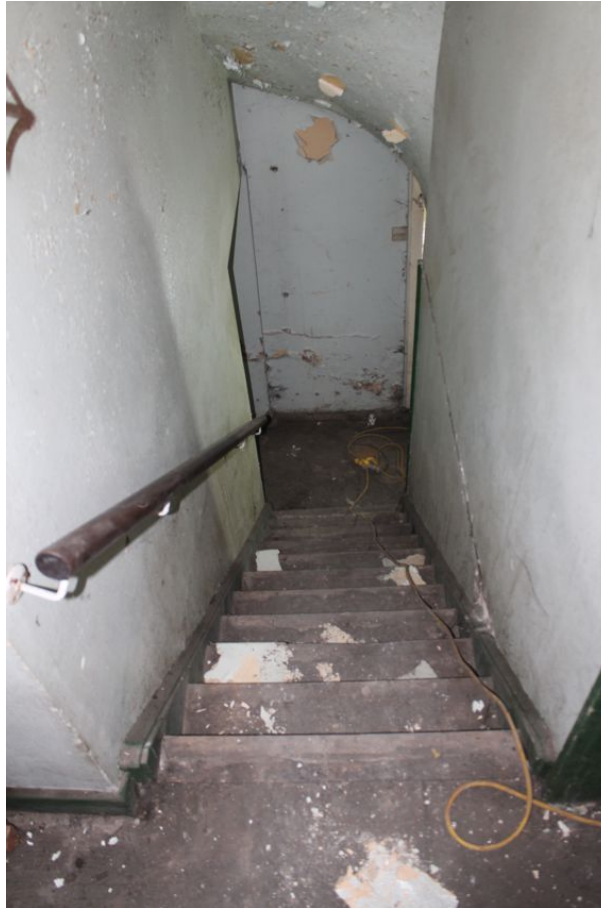
Photograph 12 Staircase leading down to basement from ground-floor of Rising Sun. Photograph taken facing south-east.
