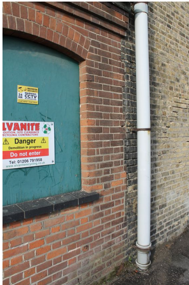
Photograph 94 Detailed shot showing joint between Structures 8 and 9. Alternating brick courses visible due to projecting bricks from Structure 8. Photograph taken facing north-west.
