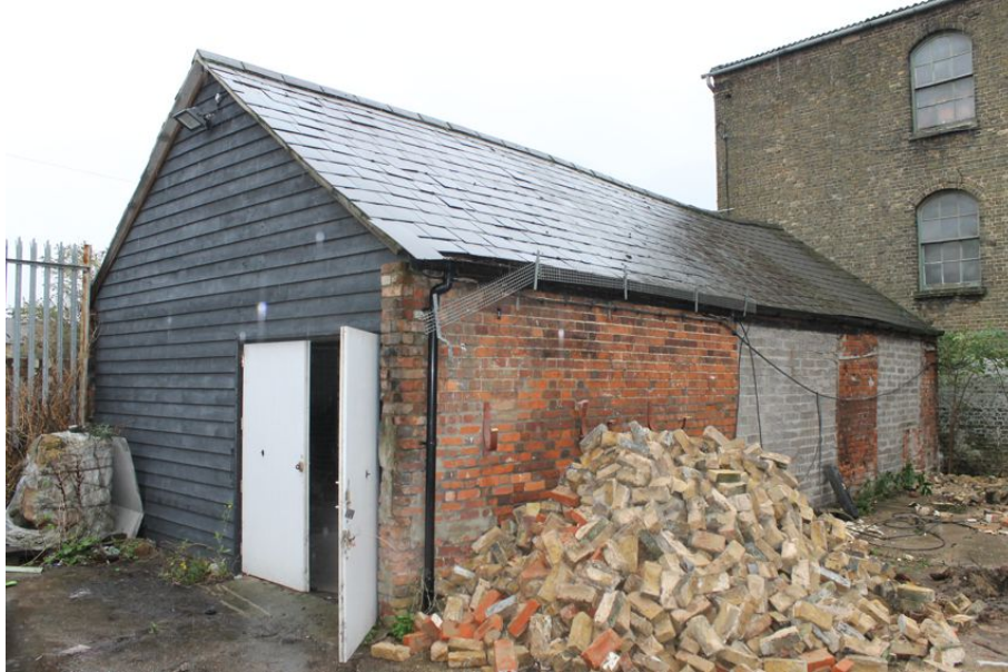
Photograph 34 North-west and south-west elevations of the outbuilding (Structure 3). Photograph taken facing south-east.
