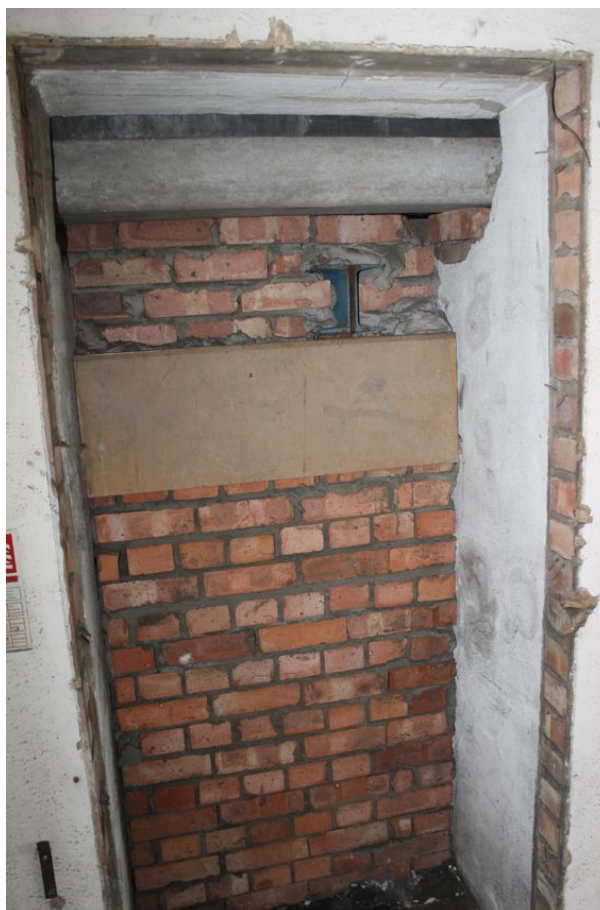
Photograph 49 Blocked entrance from second-floor of Structure 5 into northern warehouse. Metal girder supporting roof of northern warehouse visible. Photograph taken facing south-west.
