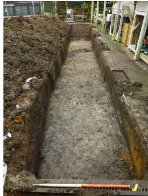
Photograph 2 T3 trench shot – looking SSE
