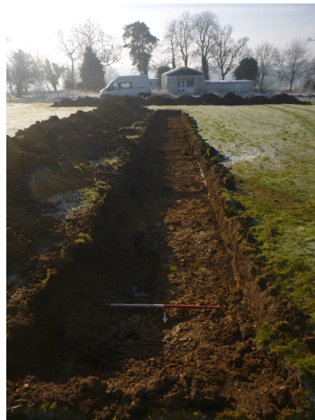
Photograph 2 T2 trench shot – looking south
