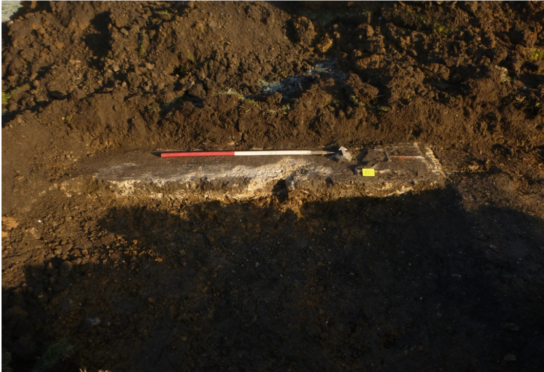
Photograph 3 Detail of concrete foundation F1 in T1. This foundation corresponds with the location of a Second World War building on the site, part of a camp attached to an ammunition dump at Wakes Colne.
