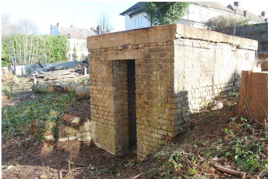
Photograph 4 South-west elevation of air-raid shelter, showing entrance. Photograph taken facing north.
