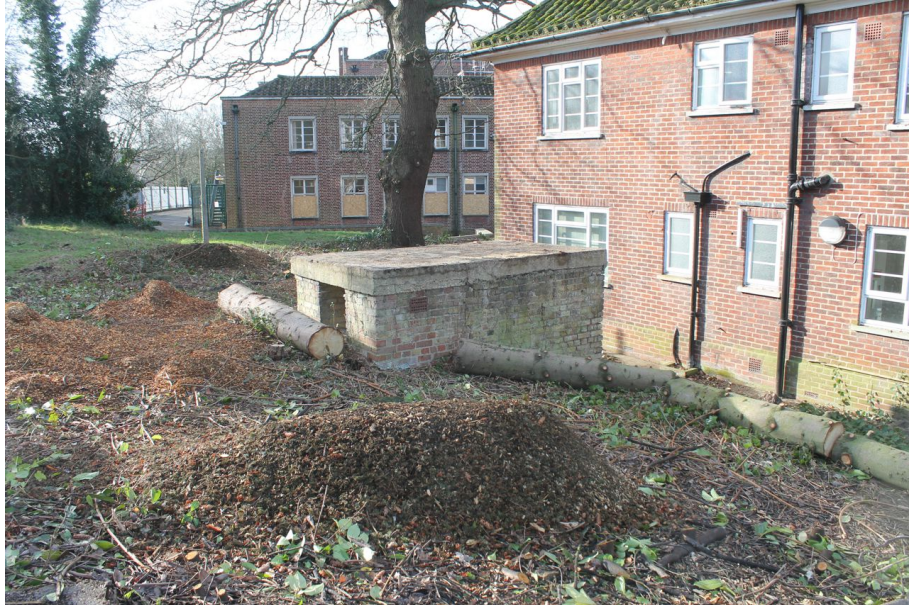
Photograph 1 North-west and north-east elevation of air-raid shelter. Police Station building visible in background. Photograph taken facing south.
