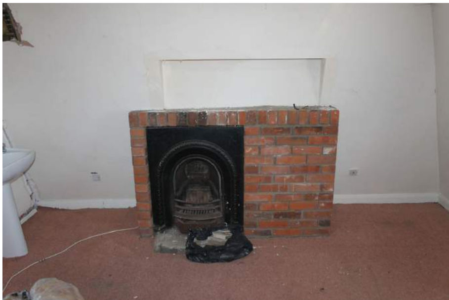
Photograph 25 Rebuilt northern fireplace surround on second-floor. Photograph taken facing west.
