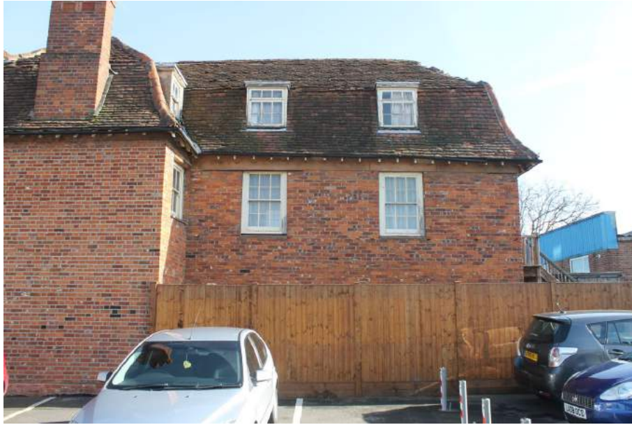
Photograph 13 West elevation of extension. Photograph taken facing east.
