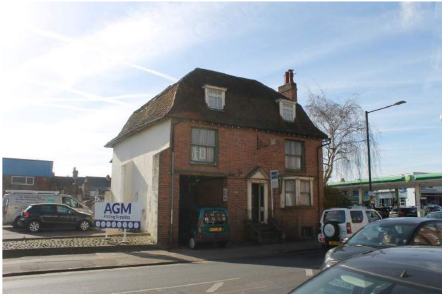
Photograph 1 North and east elevations of 79 Magdalen Street. Photograph taken facing south-west.
