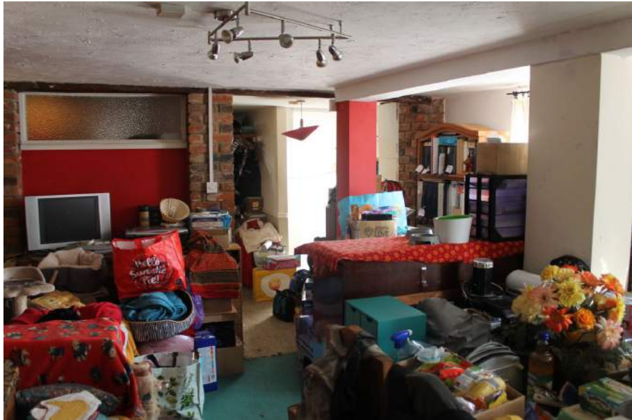
Photograph 20 Ground-floor of extension, showing brick pillars supporting upper floors of main range. Photograph taken facing north.
