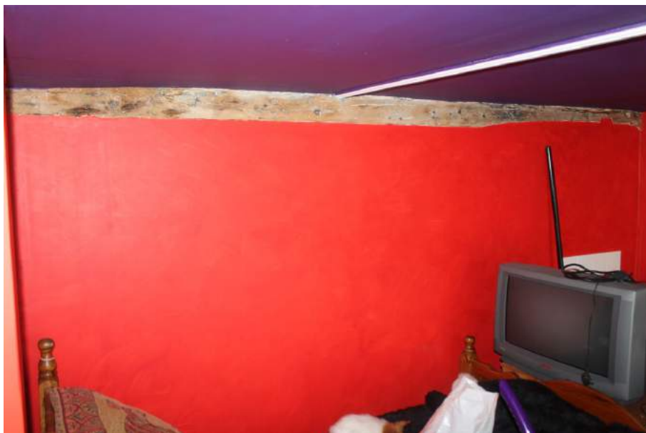
Photograph 23 Visible beam in north-west room on first-floor. Photograph taken facing south.
