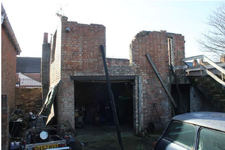
Photograph 28 North elevation of outbuilding. Photograph taken facing south-west.
