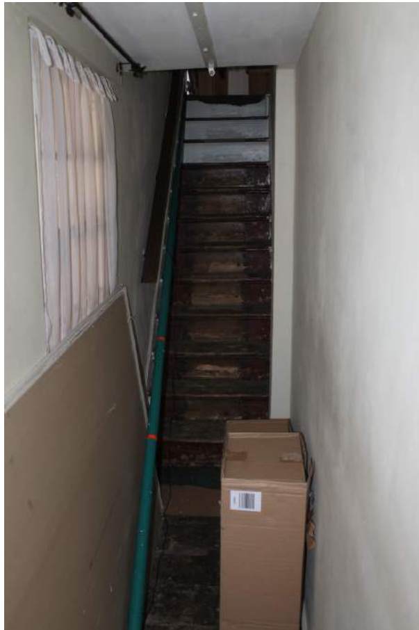
Photograph 21 Staircase leading up to first-floor. Photograph taken facing south.
