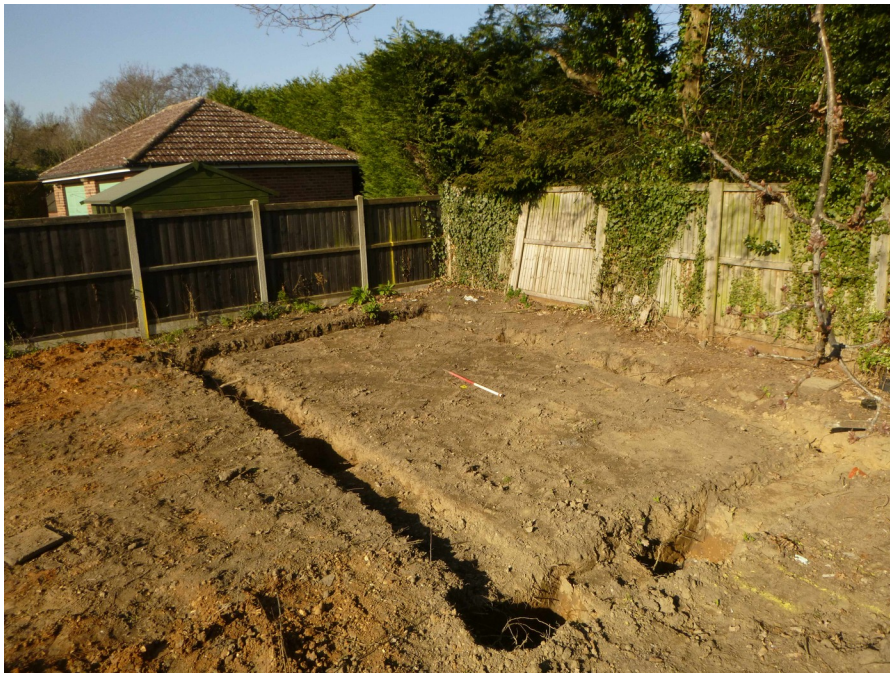
Photograph 1 Storage unit foundations, looking northwest
