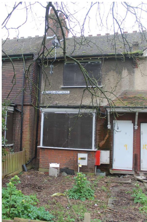
Photograph 7 North-east elevation of No 10. Photograph taken facing south-west.
