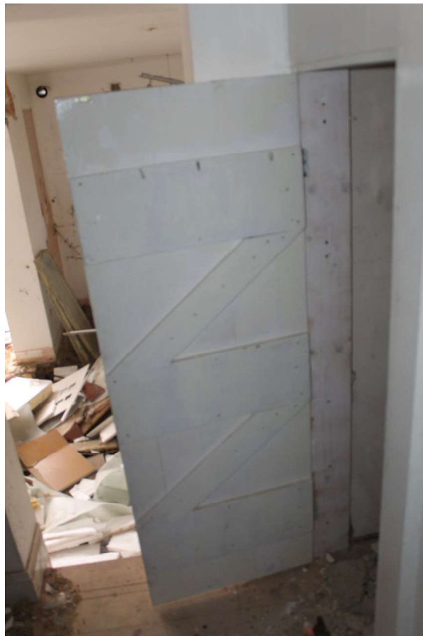
Photograph 17 Surviving vertical-planked door on ground-floor of No 10 leading into cupboard under stairs.
