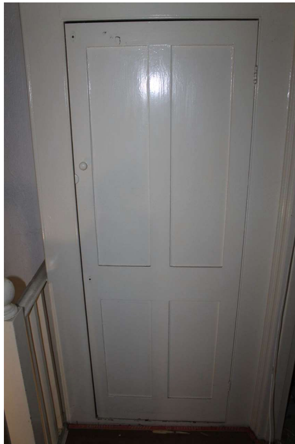
Photograph 15 Original cupboard on first-floor landing of No 12. Photograph taken facing north-west.
