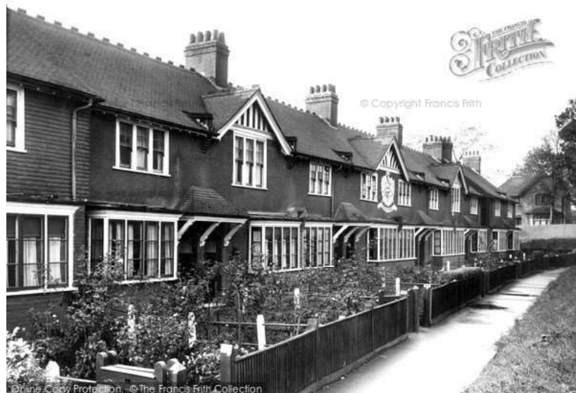
Photograph 3 North elevation of Botany Cottages. No 10 and 11 visible to left of frame. Taken from www.francisfrith.com .
