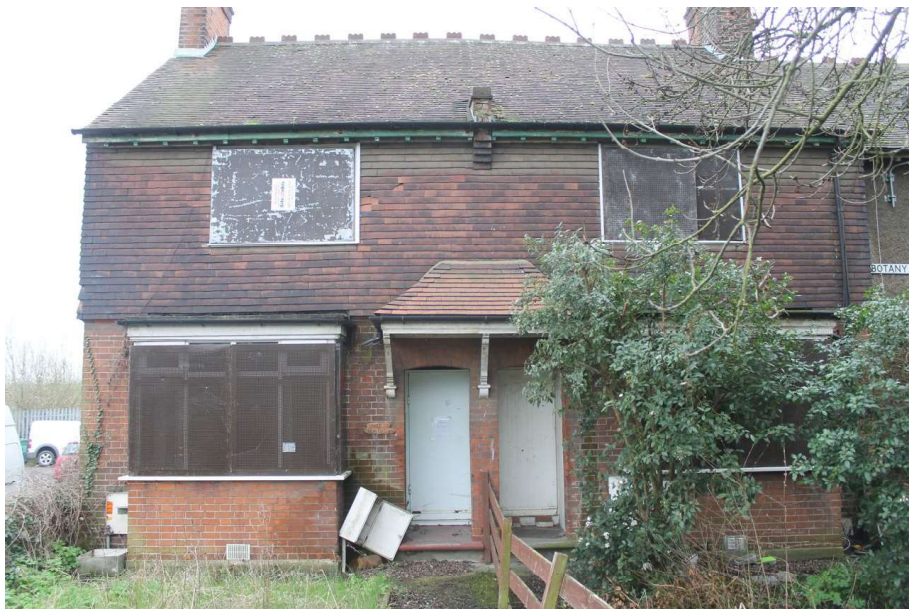
Photograph 6 North-east elevation of Nos 11 and 12. Photograph taken facing south-west.
