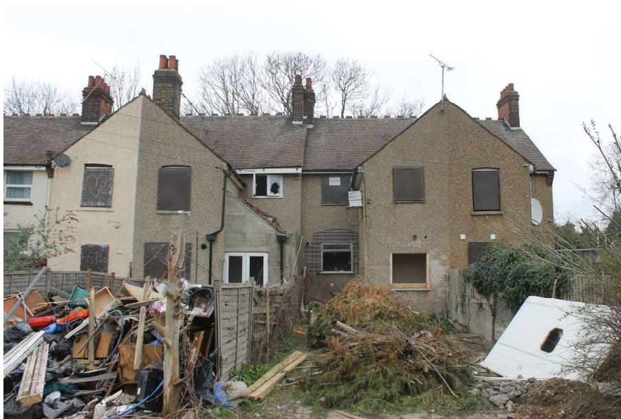
Photograph 4 South-west elevation of No 10-12. Photograph taken facing north-east.
