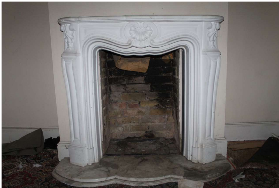
Photograph 8 Modern plaster fireplace surround in living-room on ground-floor of No 11. Photograph taken facing north-west.
