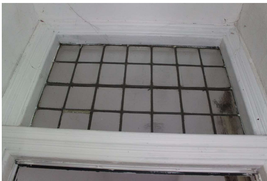
Photograph 10 Detail of original leaded light in entranceway of No 10 on ground-floor. Photograph taken facing north-east.
