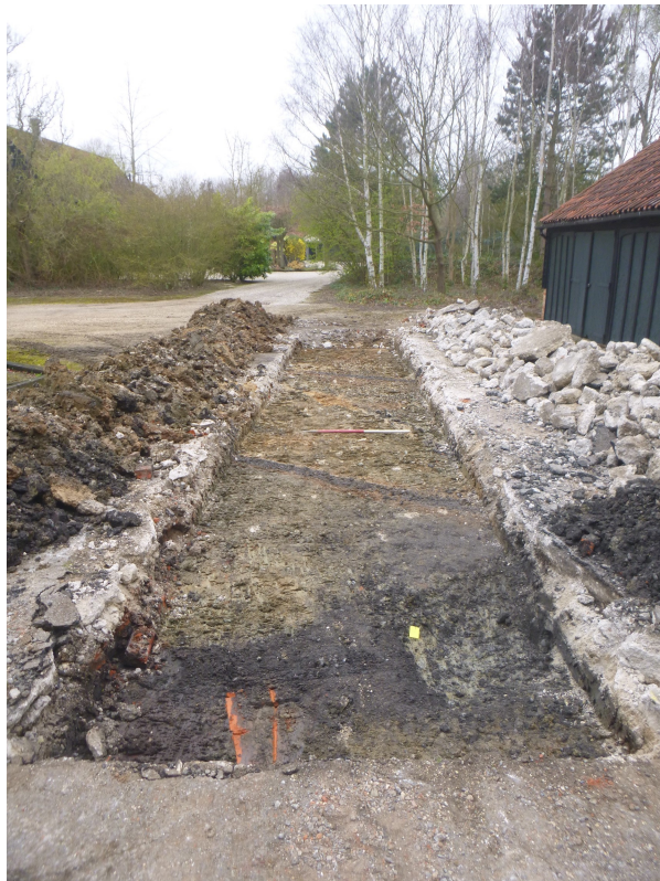
Photograph 1 T1 trench shot, looking west northwest
