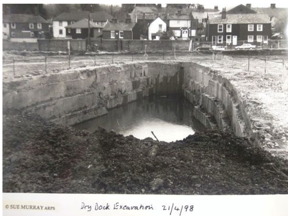
PHOTOGRAPH 1: Excavation of the Dry Dock in 1998, looking towards West Street.
