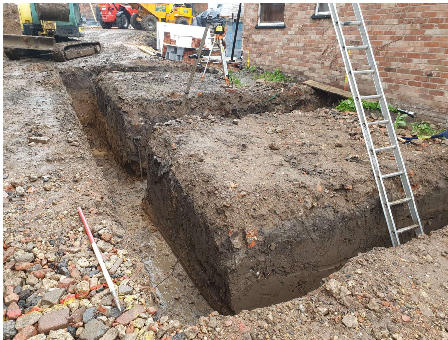
Photograph 1 Foundation trenching – looking east northeast
