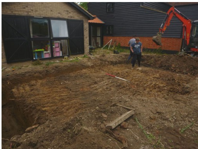
Photograph 1 Reduced level – looking northeast
