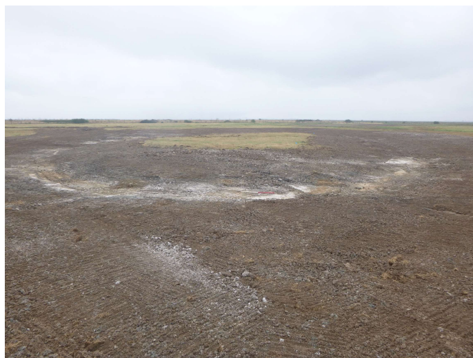
Photograph 1 Western scrape fully-excavated – looking southeast
