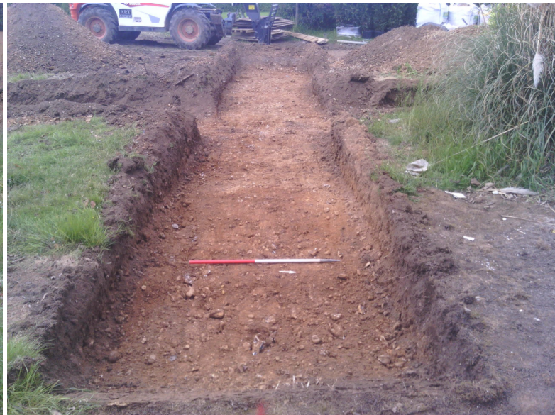
004 T2 trench shot - looking southwest (north arrow facing wrong direction)
