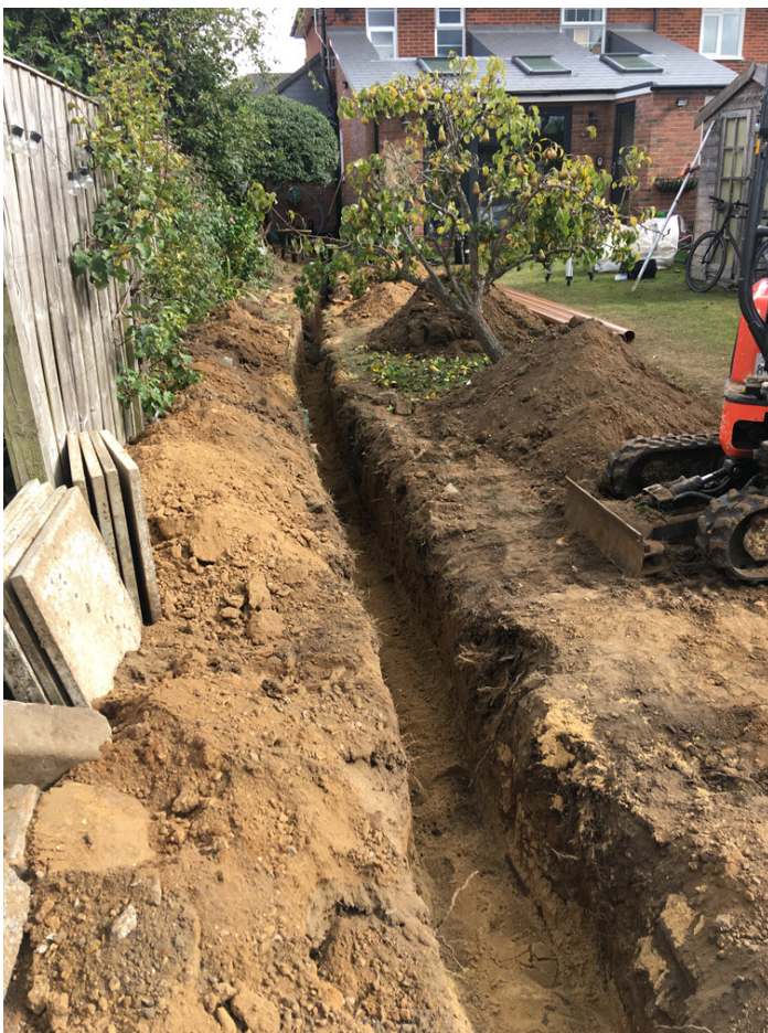
Photograph 3 Service trench, looking east
